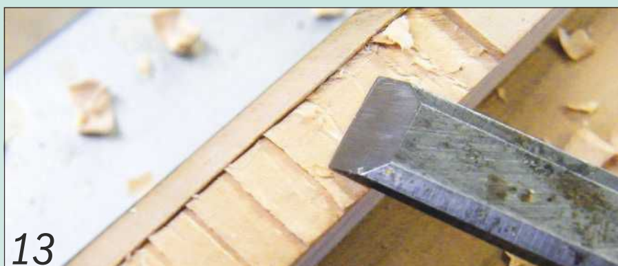
Mark the position of the lock catch on the lid and chisel out its recess
