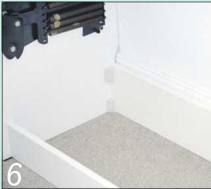
6 The rear base panel is fitted slightly forward to accommodate the skirting board
