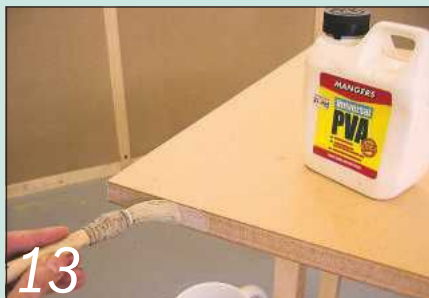
13 Seal the raw mdf edges with dilute pva adhesive to help counteract their natural absorbency
