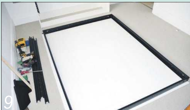
9 It was easier to have a single front panel as the metal bed frame was bolted together section by section...
