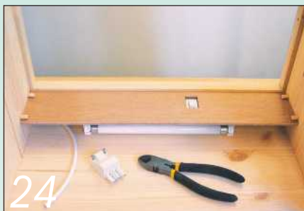
24 Make plywood blanks to screen the cabinet strip lights from view
