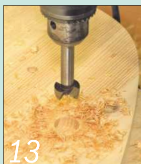
13 Drill 20mm diameter stopped holes in the shelves to take the drawer front adjusters
