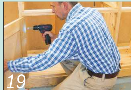
19 Hang the doors to check fit and clearance, and adjust them as necessary
