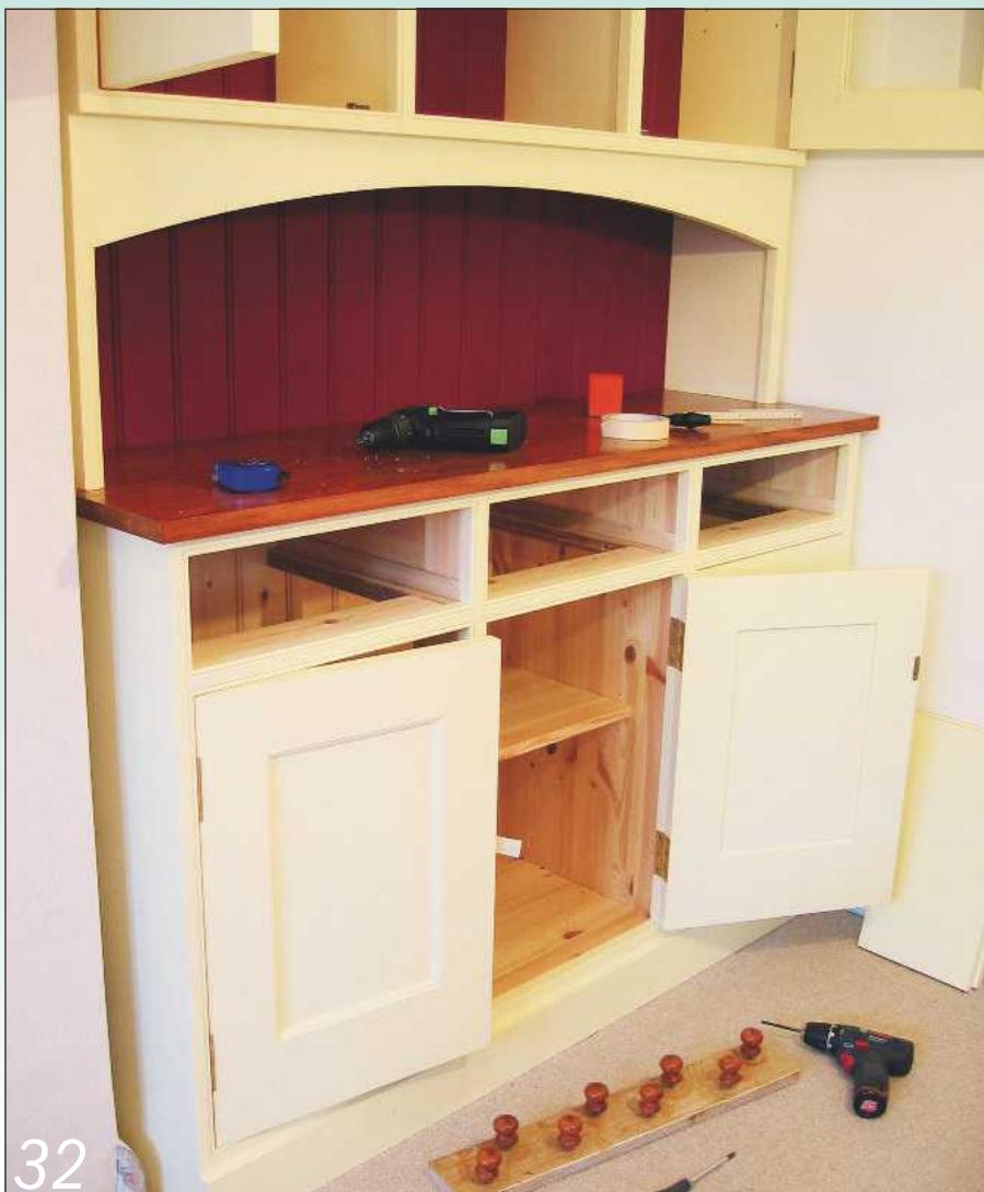
32 The fit couldn't have been much closer, especially at cornice level, but it went in smoothly
