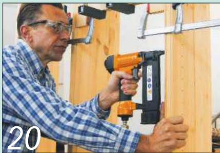
20 Pin on the scratch moulding; the arch blank above is clamped in place
