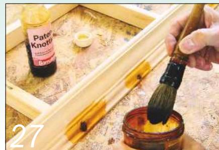
27 The cornice gets the knotting treatment before being primed
