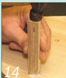
14 Knock in the adjusters using a block of scrap wood until they are flush with the shelf surface
