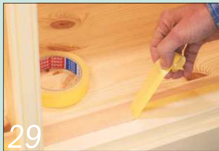
29 Judicious use of masking tape ensures cleanly painted edges
