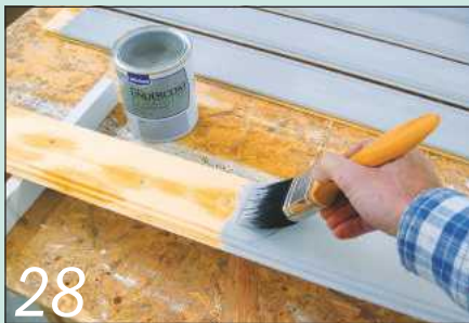
28 Prime and paint the boards individually to disguise shrinkage once the boards are fitted
