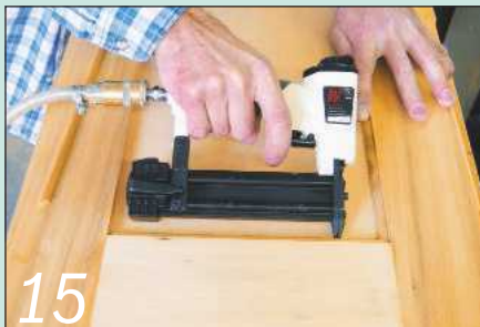
15 The panel mouldings were simply mitred and pinned into place
