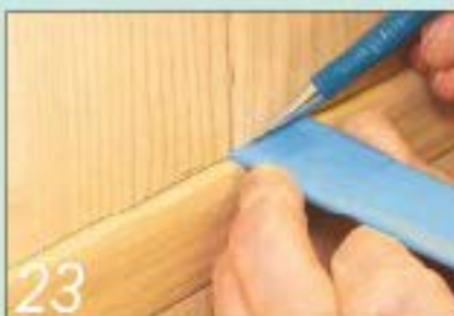
23 Using a spacer to mark the doors so you can trim them for a consistent fit
