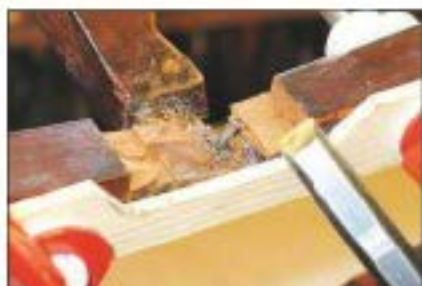
3 A brace is cramped across the cut area to give it strength at this stage. Note the shrapnel!
