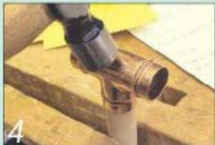
4 A gentle tap with a hammer ensured that the fittings were fully seated
