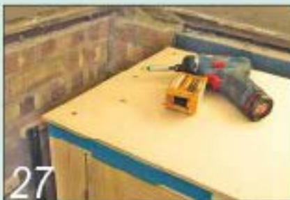
27 Fit the cornice panel temporarily with a 6mm overhang at the front and sides
