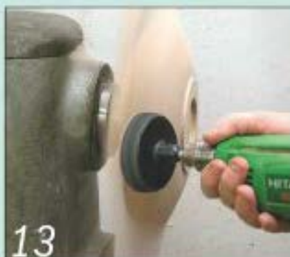
13 Power-sand the surface with the sanding disc held almost vertical
