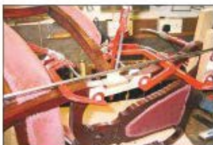
4 The first new half block is glued in place in the cut-out and securely cramped
