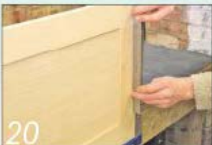
20 Cut the door panels to size, assemble the doors and check they're flat and square
