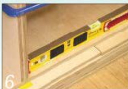
Position the two carcasses side by side and level them using shims
