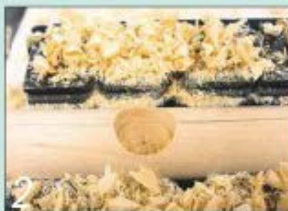
2 The 15mm diameter holes for the cross bars were bored with a flat wood bit
