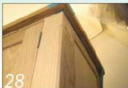
28 Cut mitres on the cornice mouldings and glue them to the plywood panel
