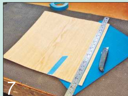
7 Cut the pieces of oak veneer slightly oversize to fit each tabletop
