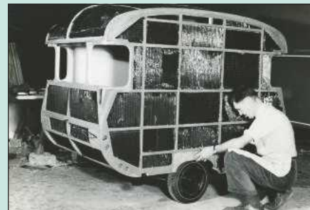
The caravan, now fully framed up and insulated, has a wheel arch support fitted. Note the pierced holes at the rear to lessen the weight
