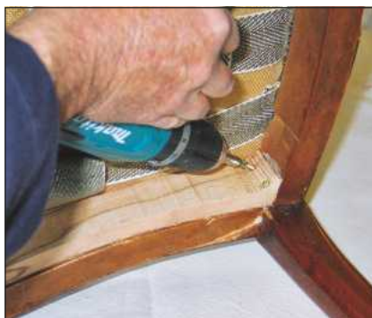
5 The strengthening piece is glued and then locked in place with a couple of screws
