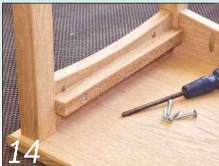
14 Cut oak slips to fit between the legs and screw them to the side rails
