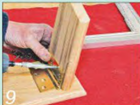
Offer up the first leg, drill another pilot hole and drive in one screw. Repeat for the other leg
