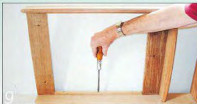
9 Glue and screw the two 16mm square vertical battens to the sides of the fitment, flush with the cross rails
