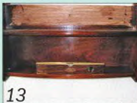
13 Check that the fitment is level, then drive fixing screws through the holes in the cross rails
