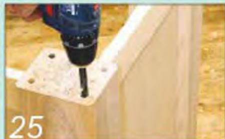
25 ...and finished the job with a 10mm twist drill bit to achieve the full depth
