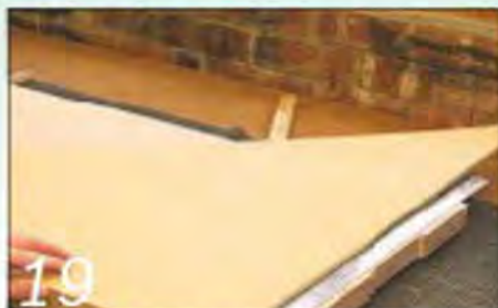
19 Mark and trim the panel ends square and to the required length
