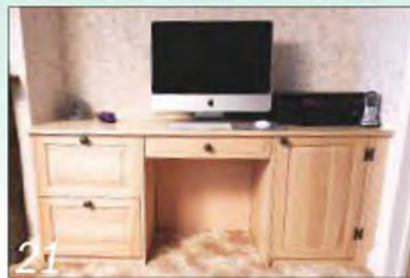
21 Finally, just add a back panel to the kneehole and the job's done
