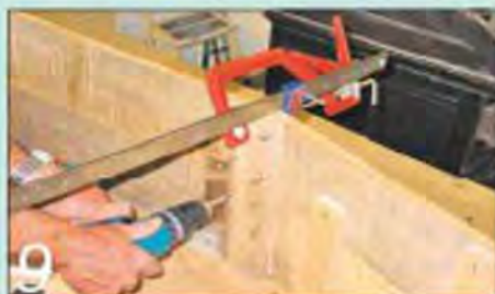
The two double-angled shoulder braces are prepared and fixed in place next
