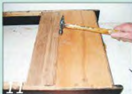
11 Glue and pin the plywood back panel into the rebate prepared for it earlier
