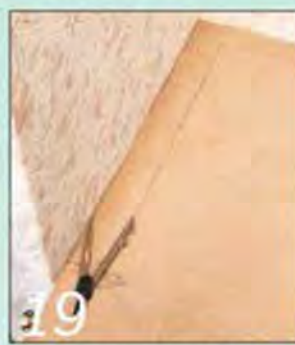
19 Use compasses to scribe a template on hardboard, then scribe round that onto the top itself
