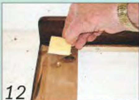
12 Stick four pieces of 12mm foam plastic to the cross rails to act as cushions for the mirror
