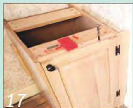
17 Prepare and fit the filler panel. Then repeat the whole process at the other side
