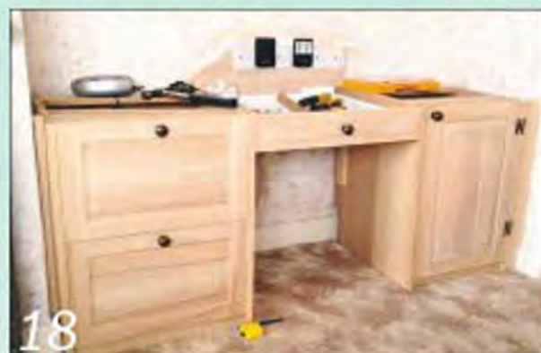
18 Screw the drawer unit in place. All we need now is the top panel
