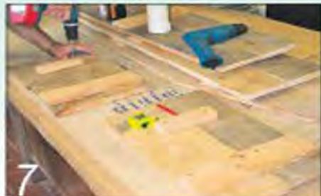
7 These short head-end side sections have a temporary brace fitted in place
