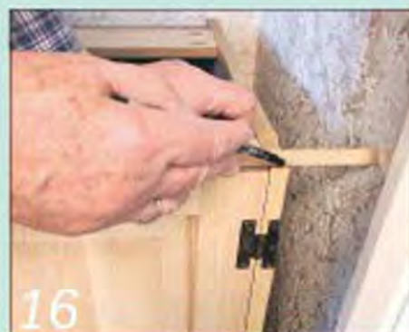
16 Use a rod to measure the gap between unit and wall at one end
