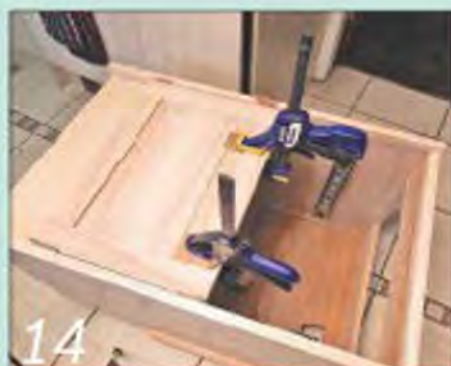
14 Place the base unit on its back, clamp the drawer fronts in place and screw them on from behind
