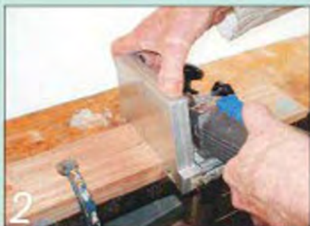
2 Cramp a cross rail to the side component to position the jointer as you make each cut
