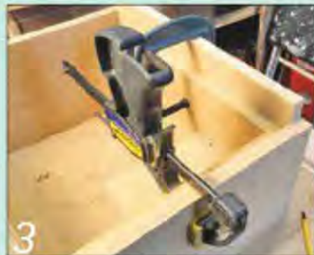
I used a clamping jig to hold the filing frame boards while I drilled and screwed them
