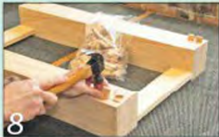
8 Dry-assemble the island legs and rails by tapping in the floating tenons
