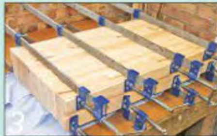
3 Assemble the legs by rub-jointing and cramping the laminations
