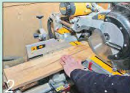
2 After planing and thickening the board, you can now cross-cut the seat to length...
