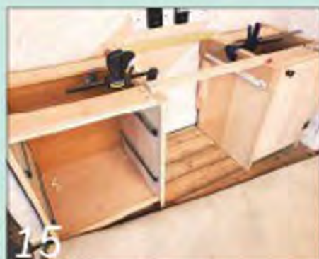
15 Cramp the base units together temporarily and set them in place in the alcove
