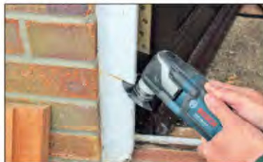
Cutting out a rotten door jamb ready for a scarf is a perfect application
