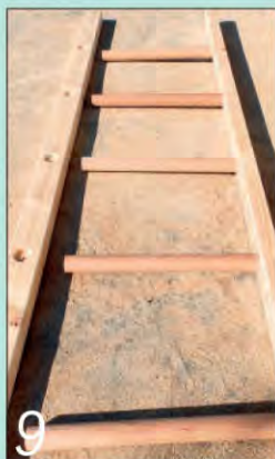
The ladder consists of dowel rungs set into the stiles, and has ladder hooks at the top
