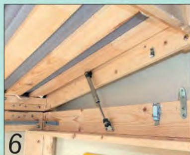
The gas piston, the latch and the guide peg are fixed to the side rail; see fig 1 for their positions
