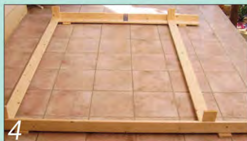
Repeat the same assembly procedure for the full-height frames
