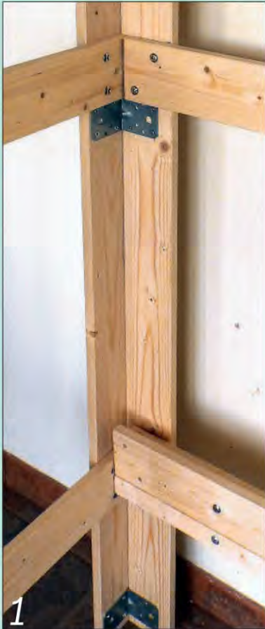
Two metal angle brackets are used to reinforce each of the four lower L-posts...
