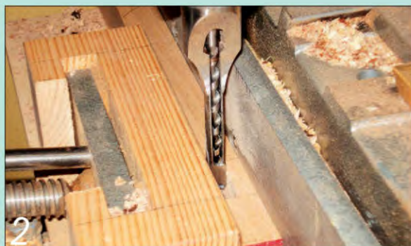
Use a bench mortiser (if you have one) to cut all the mortises
