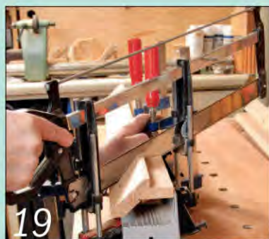
19 You'll need a packing piece to raise the cornice clear of the bed of the mitre saw
