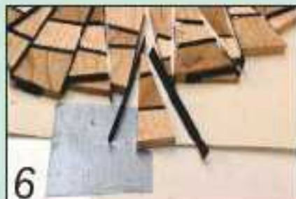
6 You'll need to shape the last piece carefully to fill the final gap
