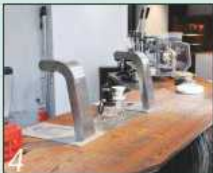
4 You wouldn't normally use softwood for a bar top, but this Kebonised version in a swanky London coffee bar will likely outlast even the espresso machine.
