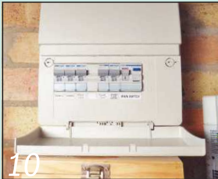
10 A complete rewire began with a small modern consumer unit fitted with a residual current circuit breaker for safety
