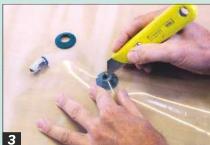
3 Pierce the membrane over the valve housing with the tip of a sharp knife blade
