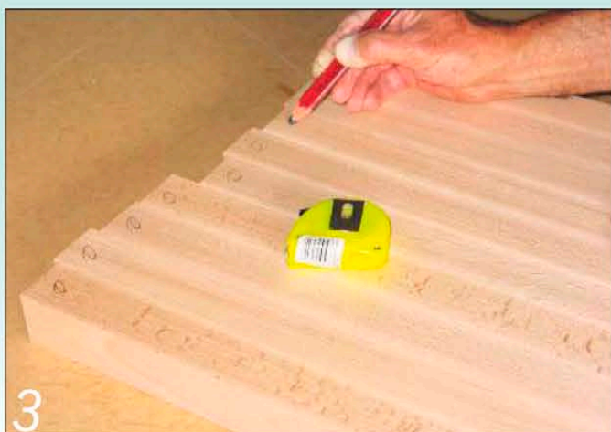
3 The strips will be assembled showing the 38mm faces; mark them all
