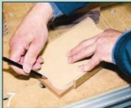
Use the template in the shaping jig to mark the curves on the bookcase sides
