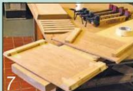
7 Stick packing pieces to the top and bottom of the carcass with masking tape
