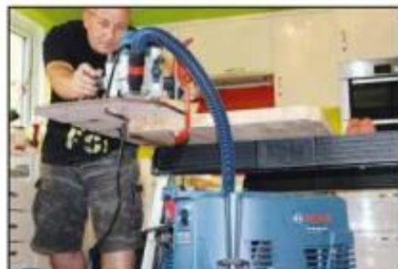
Take several passes to ensure a clean cut. Then reverse the worktop and make the mating cut
