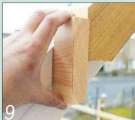
9 Use a fascia board offcut to mark the angled cuts needed on the gable rafters
