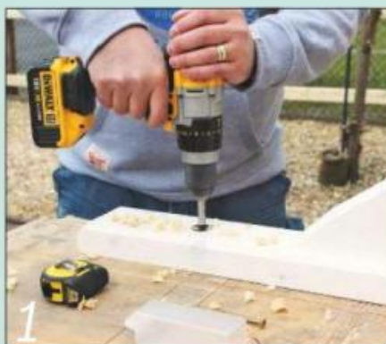
1 Drill counterbores and clearance holes in the two gallows brackets
