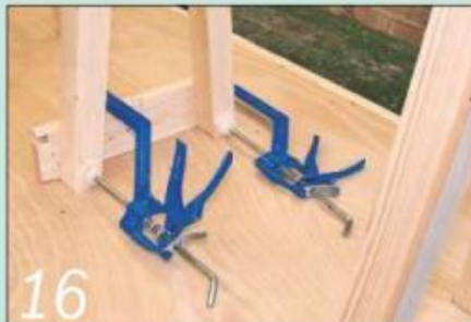
16 Cramp an offcut across each A-frame to keep it at the required level
