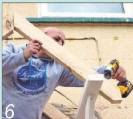
6 Fit the two front rafters to the gallows brackets with a single screw through each one
