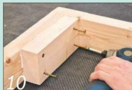
10 Add blocks to the inner corners of the base frame to take the wheel baseplate fixings
