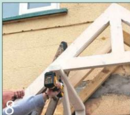
8 Lift the front gable onto the brackets and secure it with a screw at each side
