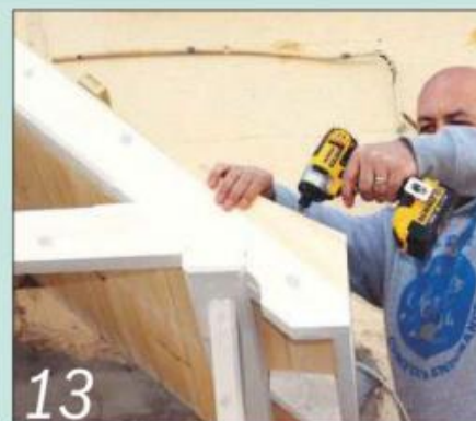
13 Add triangular tilting fillets to the gable to match the level of the fascias
