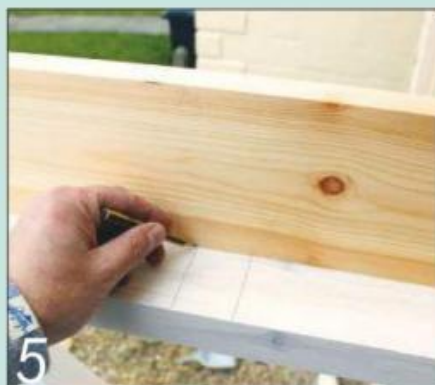
5 Set out the rafter positions on one bracket and transfer them to the ridge board
