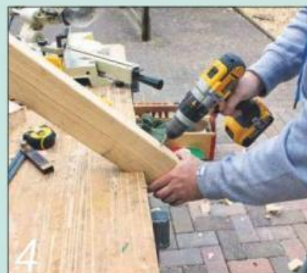
4 When you've cut the rafters to size, drill clearance holes for their fixing screws
