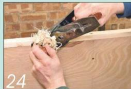
24 Use a hand plane to finish the top and side trims flush with the surface of the panels
