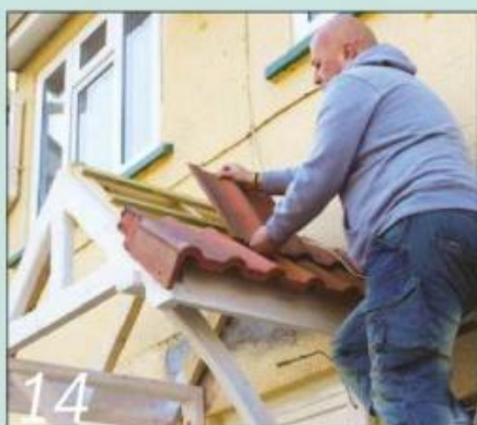
14 Position the tiles by hooking their rear lugs over the tiling battens
