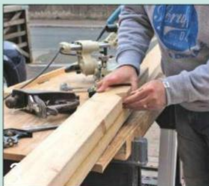
3 Mark up the birdsmouth position on one rafter and use it as a pattern for the others
