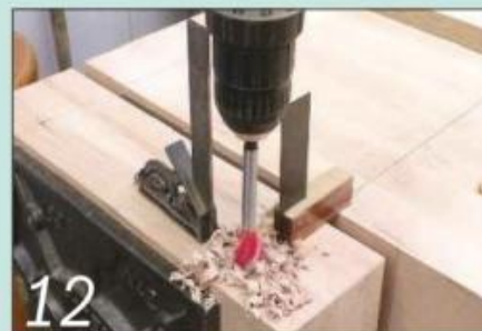
12 Drill vertical 19mm diameter holes in the vice jaw blocks to take bench dogs
