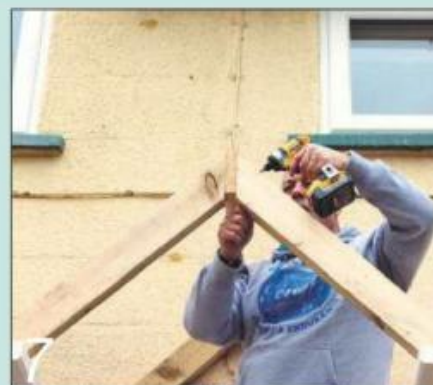
7 Fit the rear rafters, slot the ridge board in place and screw the sloping rafter ends to it
