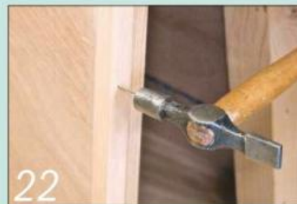
22 Fit the sloping side panels to the A-frames and attach the rebated side trims
