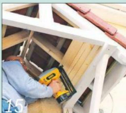
15 Line the underside of the porch roof with matchboarding, nailed to the rafters
