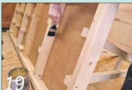
19 Seal all the parts assembled so far with a generous coat of clear varnish
