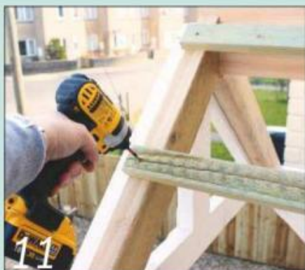
11 Position the tile battens to give an even tile overlap and screw them on
