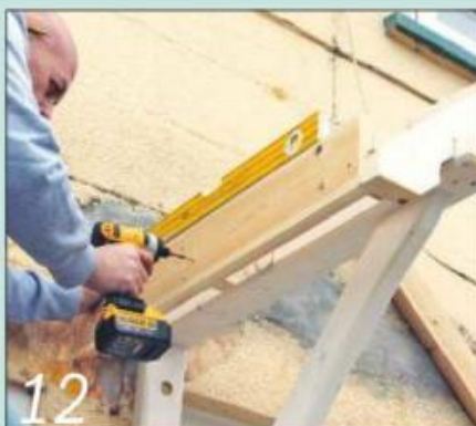
12 Position the fascia so its top edge will 'kick up' the bottom row of tiles
