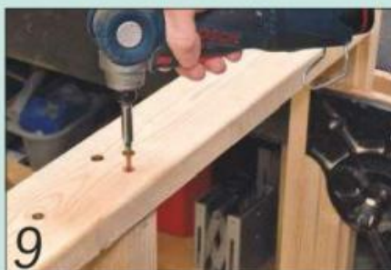
9 Cut the shoulders and fix the rails to the base frame with two screws per joint
