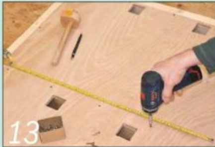
13 Put the base panel back in its rebate and fix it to the rails with countersunk screws
