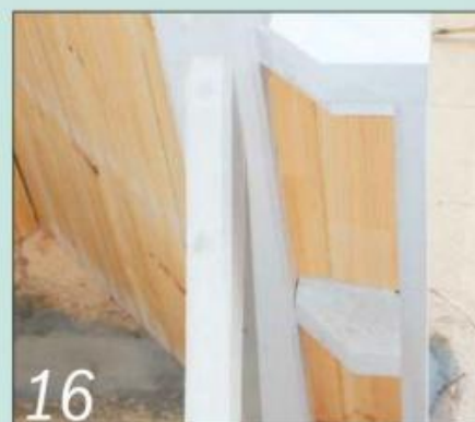
16 Finish off the eaves by pinning short board lengths between the rafters
