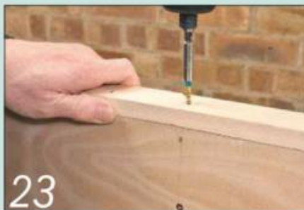
23 Add a softwood trim to protect the top edges of the two sloping panels
