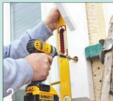
2 Offer up one bracket, mark the wall fixing positions and drill the holes in the wall
