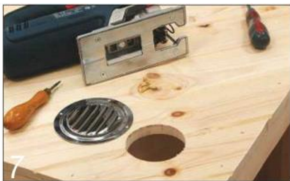
7 Plenty of ventilation is important in chicken housing. You can just drill open holes in the roof apex, but I added some cheap stainless steel grilles
