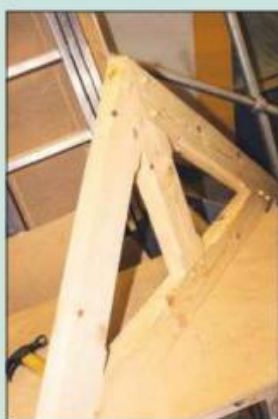
9 The truss is now ready for assembly. Note the complex bridle joint at the top
