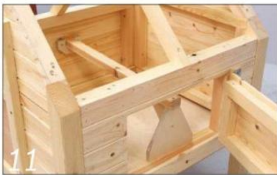
11 Here's how the perch fits inside the coop. The other end sits in a notched support fixed to the inside of the back wall
