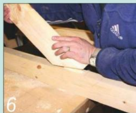
6 Always test-fit your joints. Here's the angled tenon on the cross-beam
