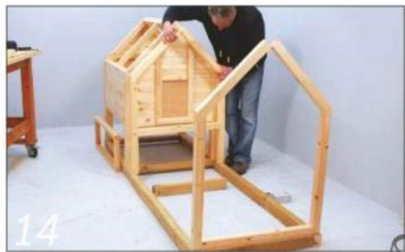
14 The rest of the run is another simple framing job, but keep the apex a bit lower so it will tuck under the coop roof
