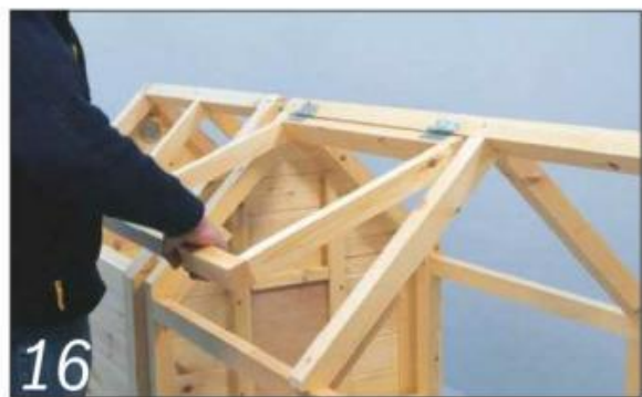
16 I made a hinged access door in the roof to give me easy access to the pophole so I could shut it at night
