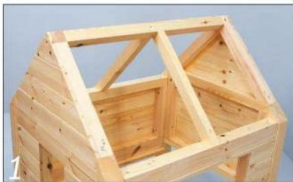
1 Screw in a square ridge piece and a couple of intermediate supports for the tongued-and-grooved roof cladding
