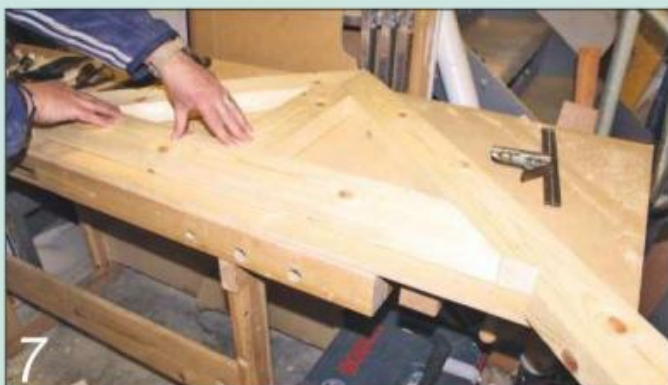
7 Check everything by laying the dry-assembled truss over the rod
