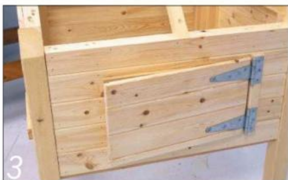
3 Use strong galvanised tee hinges to attach the side door. As it stands proud of the side of the coop, you'll need a packing strip behind the hinges to bring them flush
