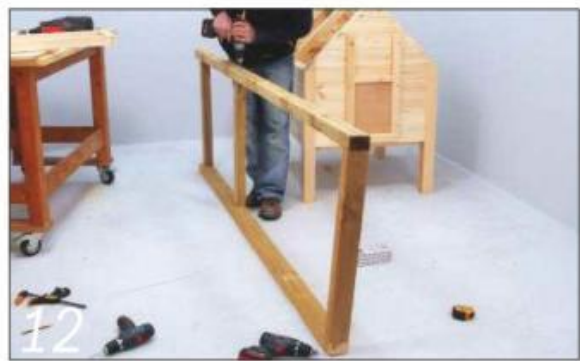
12 The base for the coop and the run is made from rough-sawn pressure-treated timber, as it will be in permanent contact with the ground
