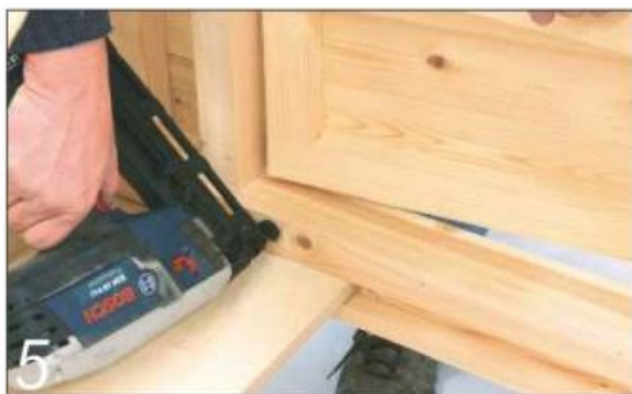
5 Fit the plywood tray in place and nail strips on above it to stop it lifting up. Leave plenty of clearance to allow for swelling... and muck!
