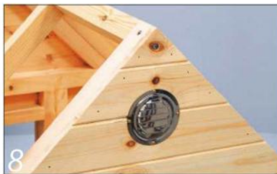
8 These just screw in place over a hole cut in the roof apex with the jigsaw, and give a much more professional look. The hens like them, anyway!
