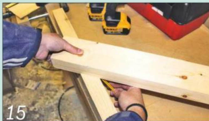
15 Lay the brace across the brackets and mark the shoulder positions
