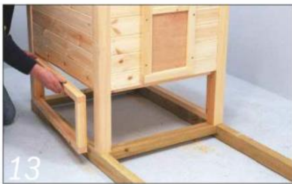
13 Wire-covered frames can then be made to enclose the rear and sides of the area under the coop
