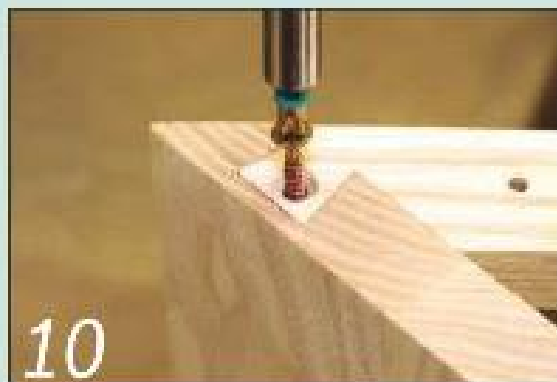
10 Glue the rail dovetails into the side panel sockets and add a screw for security
