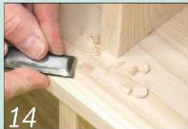
14 Hide the front screws with matching ash plugs and trim them flush when the glue is dry
