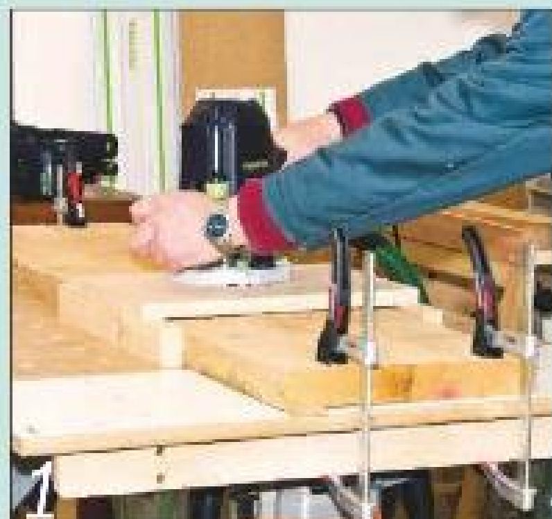
1 The levelling jig slides over the oak bench top to rout out the I-shaped channel for the frame
