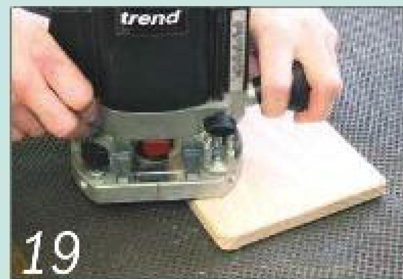
19 Then use a router cutter to round over the front edges of each section
