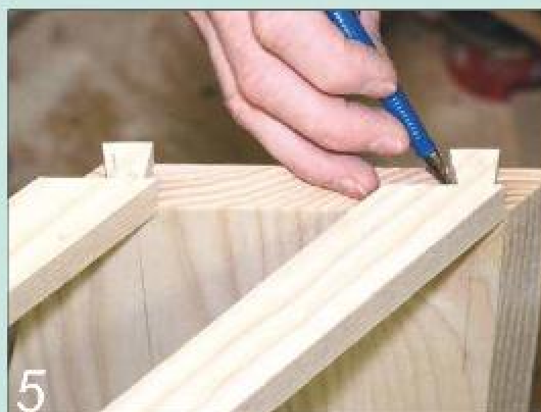
Use the angled tails to mark the socket outlines on the top edges of the side panels
