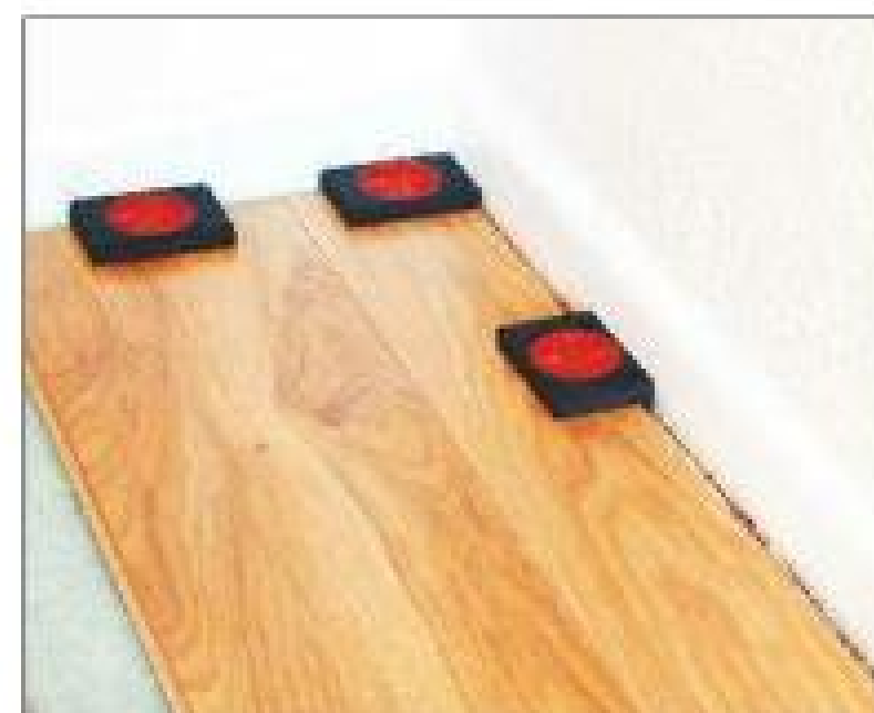
Set around the perimeter of the flooring, they take up any discrepancies in the walls
