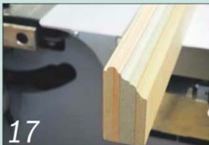
17 It took several passes with a multi-profile router bit to build up the cornice profile
