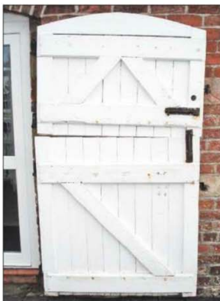
This crudely adapted two-part stable door has the lower brace running the wrong way
