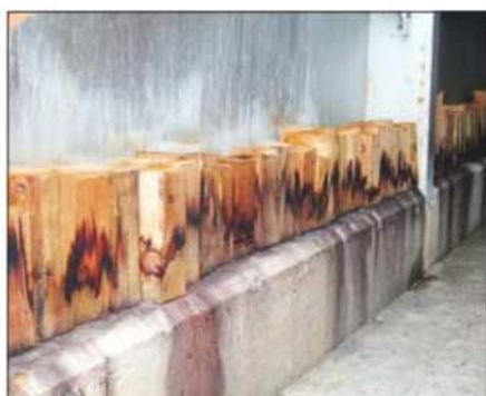
These blocks – now firewood – had to be trimmed off to allow the kiln doors to close
