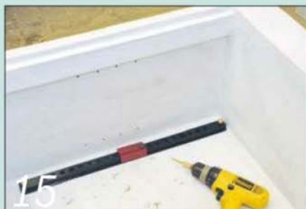
15 This Veritas jig makes it easy to drill accurate holes for the shelf support pegs
