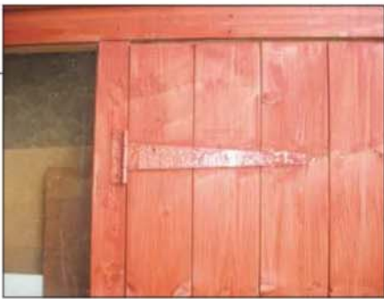
The T-bar hinges on this shed door align with and are screwed into the ledges
