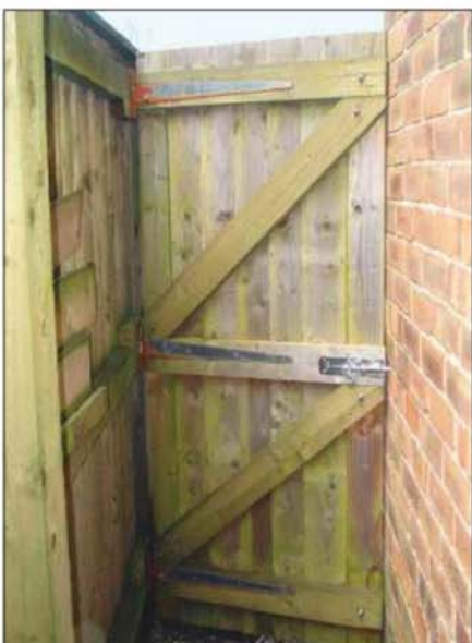
This standard garden door has a pair of correctly sloping braces between the ledges
