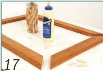
17 Mitre the ends of the top frame members and biscuit-joint them together
