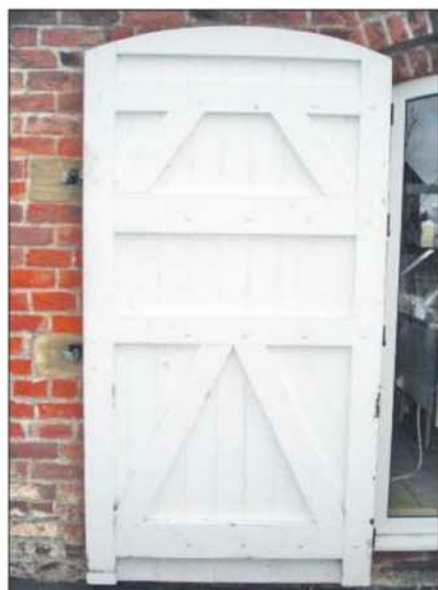
This old door has elaborate double braces and thus can be hung on either edge
