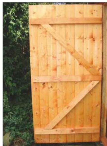
This basic commercially-made garden shed door can be hung on either edge
