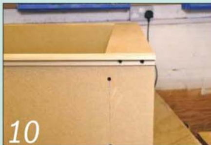
10 The T-section moulding needed drilling and countersinking so I could attach the plinth
