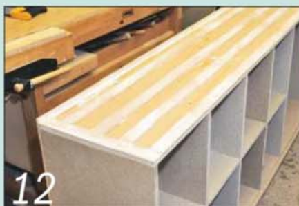
12 I applied glue to the rebate of the front T-section moulding and all the spacers
