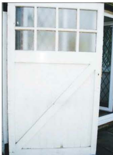
The left-hand one of a pair of traditional garage doors also shows the correct bracing
