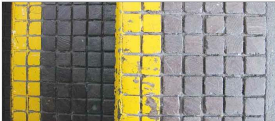
This endgrain staircase is still in everyday use at City College Brighton. Blocks are set in steel grid
