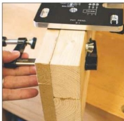
The jig is made up of a timber beam with a sacrificial mdf facing
