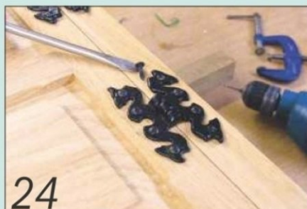
24 Hang the door in its frame with a pair of suitable surface-mounted hinges
