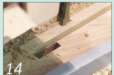
Cut 20mm deep mortises and grooves on the inside faces of the legs
