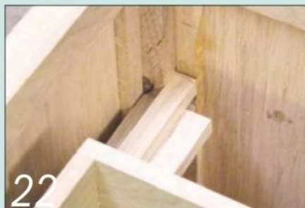
22 The drawer guides are slim strips glued to the tops of the drawer runners
