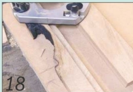
18 Use scrap wood to support the router as you cut the rebates in the frame
