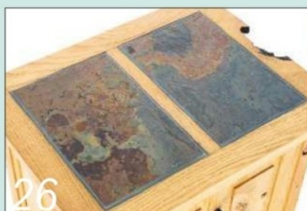
26 Fill the narrow gaps between the slate and the frame with flexible grey grout
