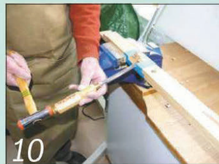
Cut down each side of the joint and chisel out the waste wood
