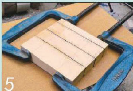
5 Use a good-quality glue and cramp the strips together securely while it sets
