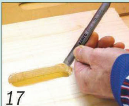
17 Clean up the inside edges of the saw cut with a chisel and a gouge
