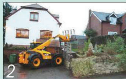
2 The granite worktop came on a steel frame which could be lifted over the steps by the forks on the Teleram. We couldn't have managed without it
