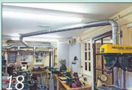
18 To get the pipe over to the drill press I cut a tee into the existing ducting
