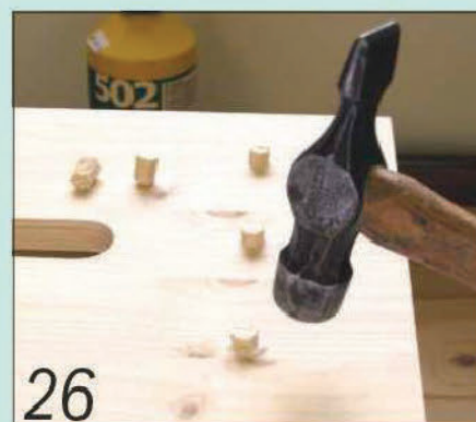
26 Tap a glued plug into each hole, aligning the endgrain carefully
