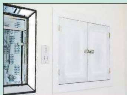
6 The fillet allows the hinges to be recessed into the edge of the door and will be invisible once it's been painted
