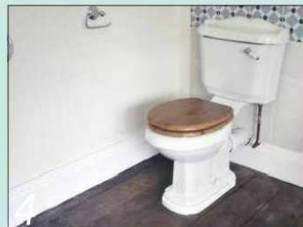
4 The plinth was needed to level the pan and to bring the pan outlet in line with the soil pipe fixed in the wall
