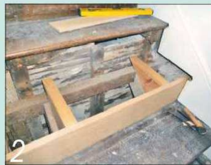
2 There were two joists under the stairs onto which we fixed some wedge-shaped blocks to support the treads
