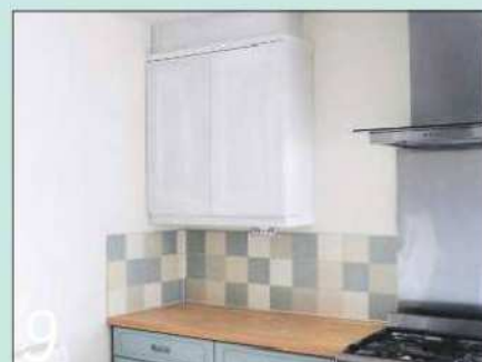
9 This necessitated a large cut-out in the top and back of the cupboard, neatly concealed by the cornice and top box
