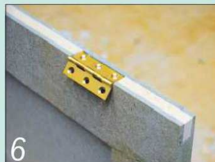
6 The fillet allows the hinges to be recessed into the edge of the door and will be invisible once it's been painted
