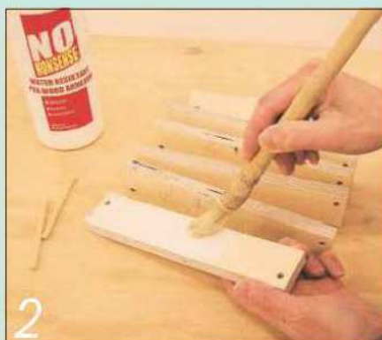
2 Each piece can now be separated, glued up and reassembled in the stack with confidence...
