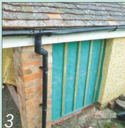
With the house walls being more out of square than we had anticipated, and with a coating of very rough pebbledash to cop with, the main infill panel ended up an extremely snug fit. After screwing it in place we used construction foam to fill in any gaps round the perimeter
