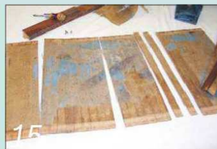
15 The old hessian backing underneath was splitting away in sections
