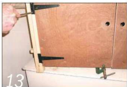
13 Cut the doors to size, bore a finger hole in each one and hang each on with a pair of hinges
