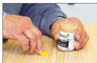
Osmo recommend the use of a plastic spatula for applying the filler
