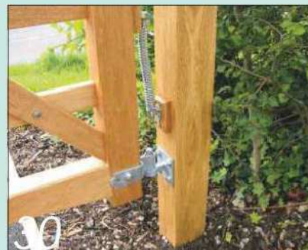
30 ...and to hang the gate and then fit the latch and the closing spring
