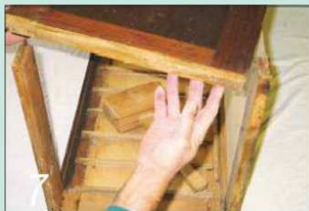
7 I started to dismantle the cabinet by knocking the frame joints apart
