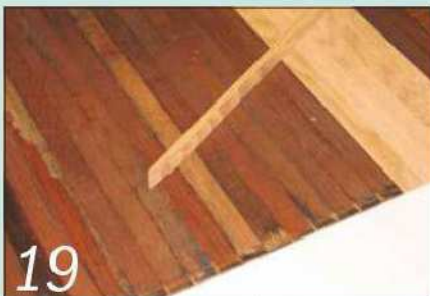
Six new slats were needed; the old ones were simply sanded down ready for refinishing
