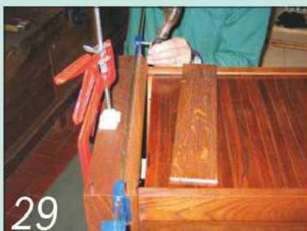
The new skirting was mitred, glued, pinned and cramped in place
