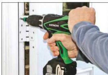
The torque control allows driving power to be kept low for fixings in uPVC
