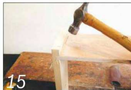
15 Drive in pins at an angle as shown to secure the drawer sides to the front
