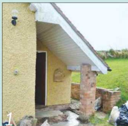
The house is on a very exposed site and the door had been set well back inside a large overhang. Our job was to build a porch by panelling in up to the pillar, so our first task was to dig some shallow footings for the dwarf walls
