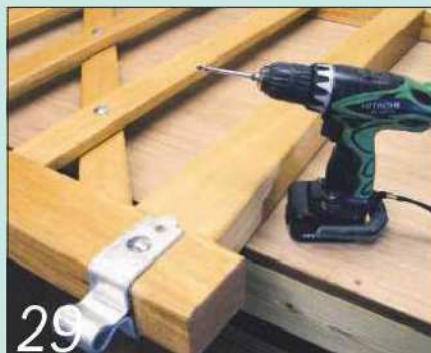
29 The last job was to attach the upper and lower galvanised double-strap hinges...
