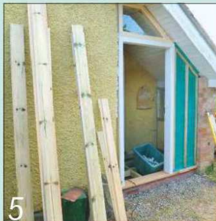
The door frame and sill were also made up in the workshop. The frame and glass above the door were added once the frame had been fixed in place on top of its engineering brick support wall
