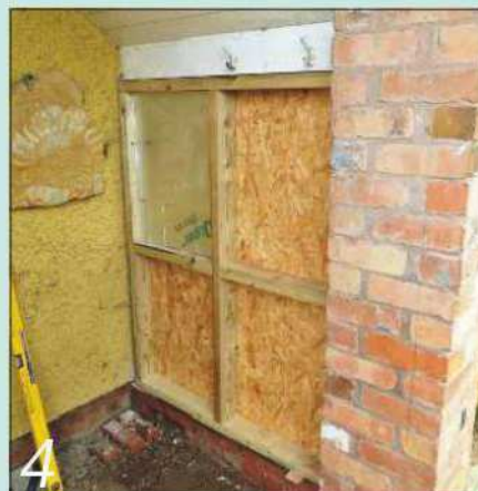
We fitted insulation into the wall panels on the inside and then covered them with a vapour barrier. This is a thin polythene sheet that prevents warm air inside the porch from condensing on the internal cold face of the OSB and soaking the insulation
