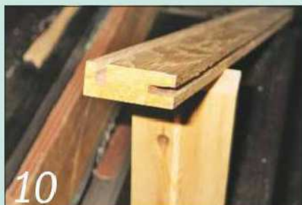
10 The new frame piece was planed and grooved to match the original
