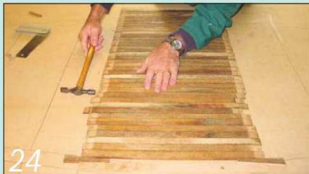
I wedged the tambour slats between two battens and lined them up
