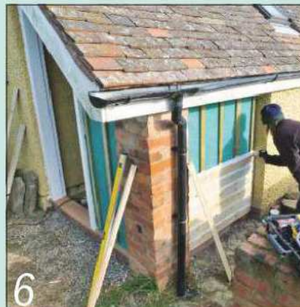
The biggest advantage of the Osmo Country Colours paint was that we were able to decorate the shiplap cladding as we applied it. All we had to do was to protect it from frost
