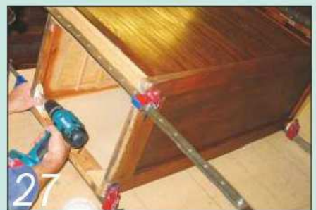
I decided to reinforce all the frame corners with some triangular glue blocks
