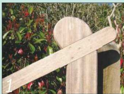
1 The existing gate had a long cross brace running into the hanging stile's curved top
