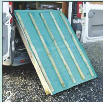
We made the wall infill panels up in the workshop. These consisted of a 100 x 50mm tanalised timber frame clad with OSB, covered in a breathable membrane and vertically battened with roofing lath ready for the external cladding to be fitted
