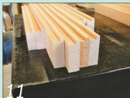
11 Rebate the stock for the glazed door frames before cutting the tenons on them
