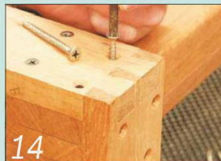
14 Fix the frame to the legs as shown, using four pairs of stainless steel screws per leg
