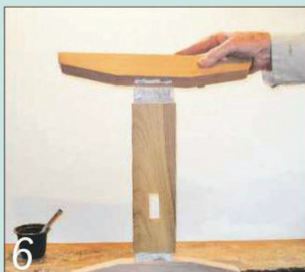
6 Use an outdoor grade of adhesive when assembling the components
