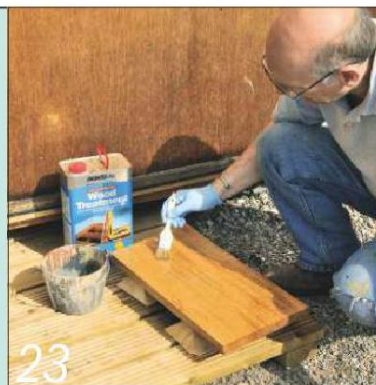
23 The two solid infill panels were treated with clear preservative before being oiled
