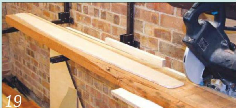
19 Use the shelf template to select the best section of the raw timber
