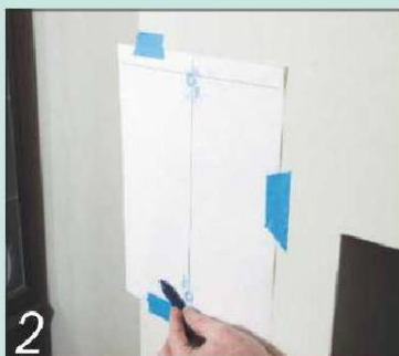
2 Drill the holes, fit the plugs and make a paper and crayon rubbing of their positions
