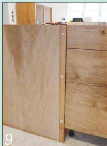
9 Once the two parts are pushed together there's no indication of where the connectors are, so I stuck some tell-tale patches of masking tape over them so I could locate the MiniMag. Once tightened, these fittings gave a very strong and completely invisible joint
