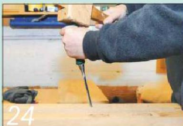
24 A taper is cut to the mortises on the outside face of the door stiles to take the wedges
