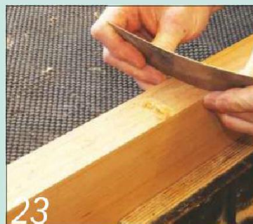
23 Scrape the excess material from the shelf to improve its fit against the wall
