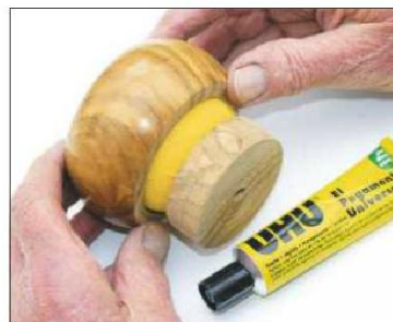
14 Push the cushion and plug into place after gluing the plug's edge, and add a felt base disc
