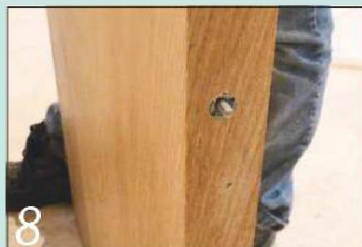
8 The connectors are screwed in with the driver bit until they're flush with the surface
