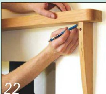
22 Scribe the mantelshelf to the wall if the chimneybreast surface isn't flat
