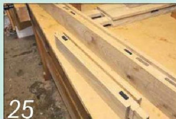
25 I glued short strips of neoprene window seal in the panel grooves to keep the panels centred
