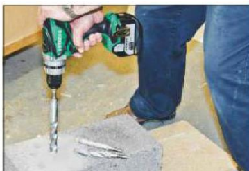
The 25mm masonry bit is soon driven through this 6-inch thick concrete block
