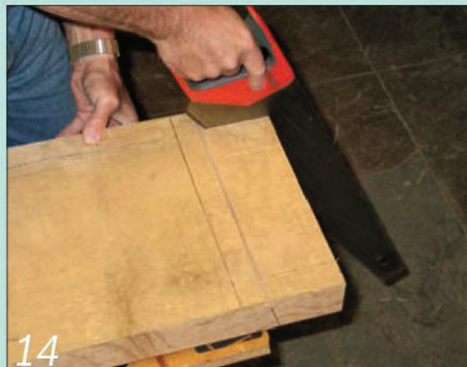
14 Finish off the cuts down to the angled shoulder line with a hand saw
