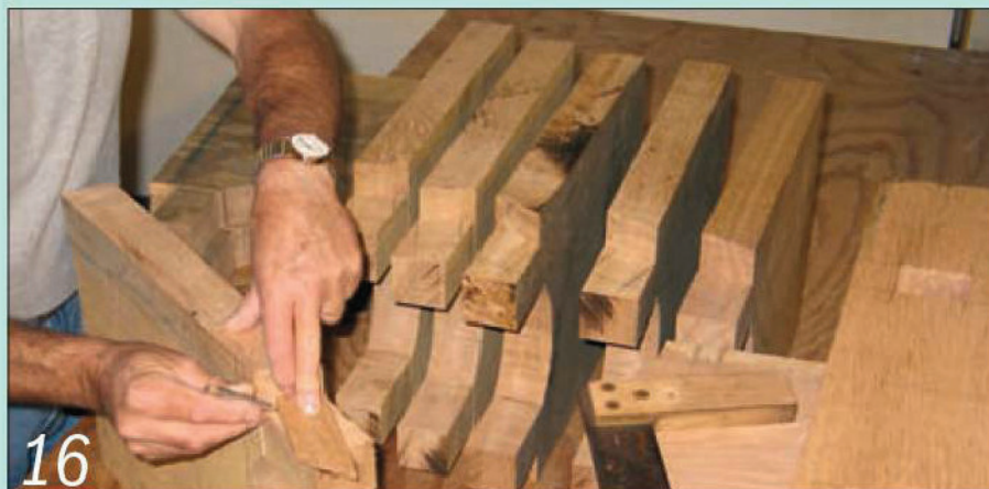
Use a small template to mark the angles to which the cheeks of the tenons need to be cut
