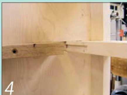
4 The oak drawer runners below the top drawer are stub-tenoned into the rear of the curved drawer rail
