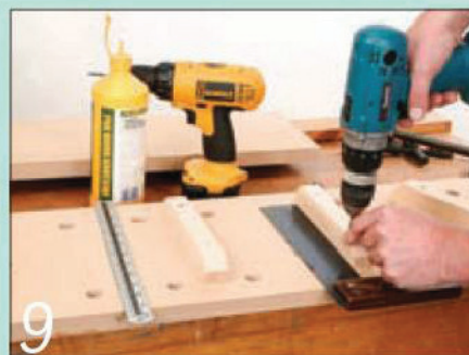
9 Glue and screw on the battens to which the four uprights will be attached
