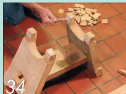
34 Fit two legs to each stretcher and apply plenty of glue in and on the joints
