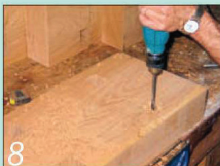
8 Use a large flat wood bit to remove the bulk of the waste from each mortise...
