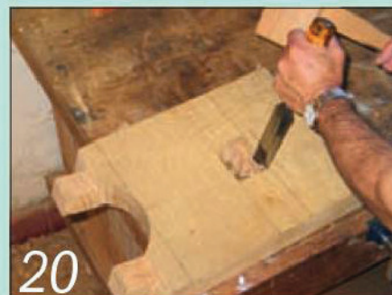
Square up each mortise with a chisel. Follow the sloping guide lines marked on the leg ends
