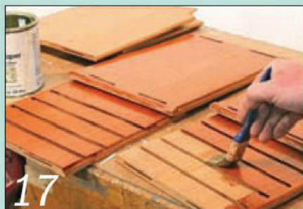
17 Apply brushing lacquer to all the internal surfaces before doing any assembly work
