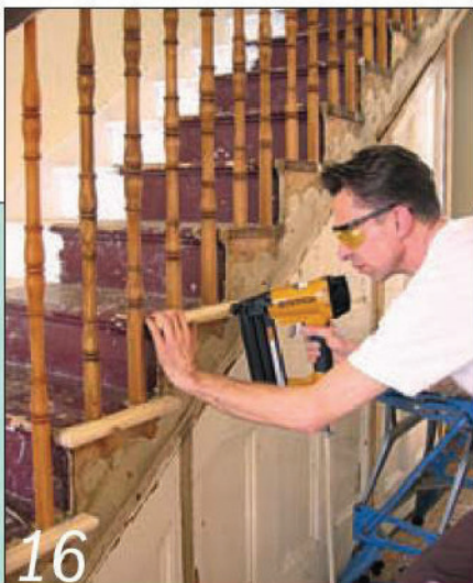
16 It makes sense to make and fit all these staircase mouldings in one go
