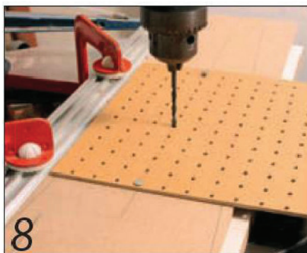
Boring the line of 4mm holes using pegboard
