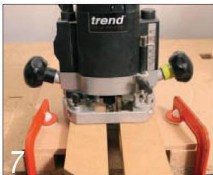
Trimming the slot to the exact size required
