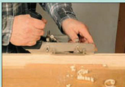
Ploughing a groove in the edge of a door stile; work progressively from the far end back towards you
