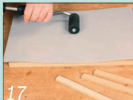
17 Apply pressure with a hard rubber roller as the strips are removed
