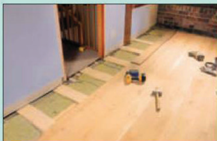
5 Wedge-shaped firrings on top of the joists take some of the slope out of the floor
