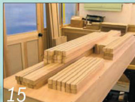
15 Frame components are stacked up, ready for the next stage
