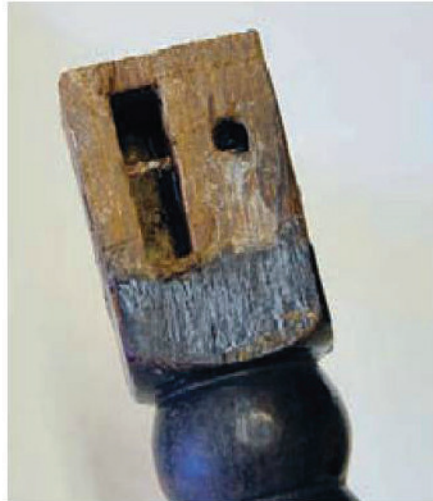
4 I couldn't remove this nail, and had to cut it flush with the sides of the mortise
