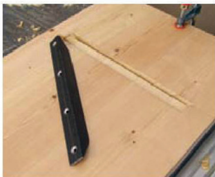
16 Form rebates for the strips with a router and circular saw
