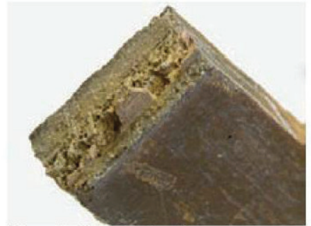
5 Several of the tenons has been seriously eaten away by woodworm
