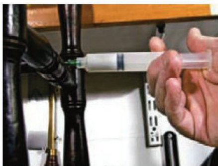
12 I filled the syringe with the glue and injected it into the joints
