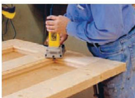
16 I used a laminate trimmer to remove the moulding from the glazing rebates
