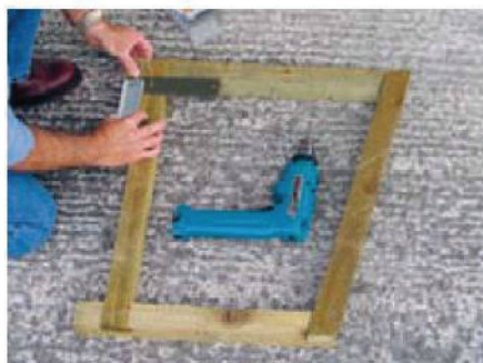
2 Make up the first end frame and check that its two bottom corner joints are square
