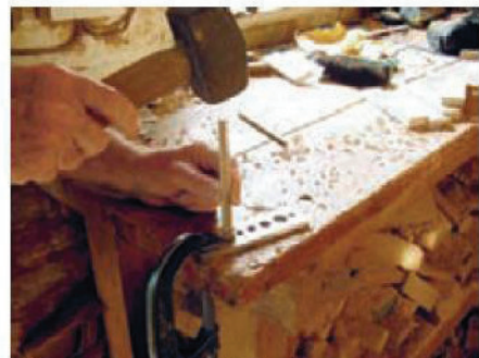
17 Use a dowel plate situated over a convenient hole in the bench to make the oak pegs, then use them to peg all the main joints
