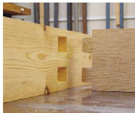
3 Check that the centre rail joints are a good fit
