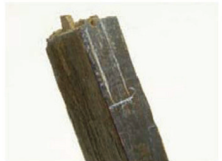
6 A white pencil is handy to mark out the positions of the new joints to be cut
