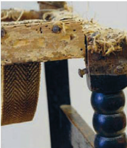
3 This joint had been repaired years ago by driving in a large hand-made nail
