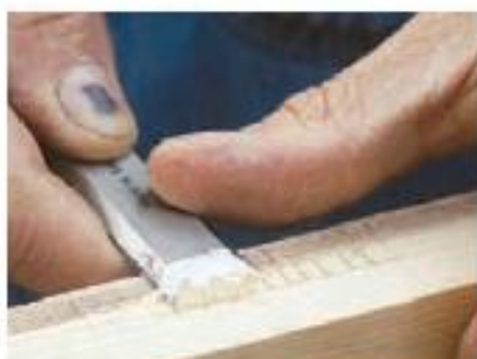
40 Remove the waste wood with a sharp chisel
