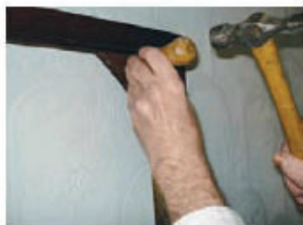
19 Offer up the frame and mark the holes
