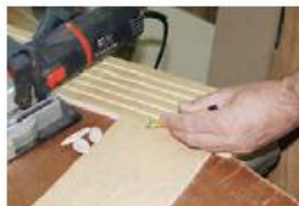
4 Mark the location of the biscuit joints on all the panels
