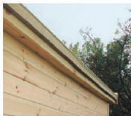
22 ...except along the back wall, where it's below the roof overhang
