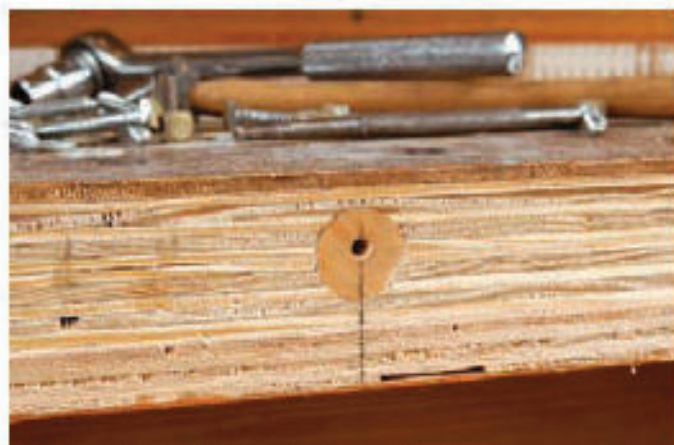
Beech plugs give a firm fixing for the edge lippings
