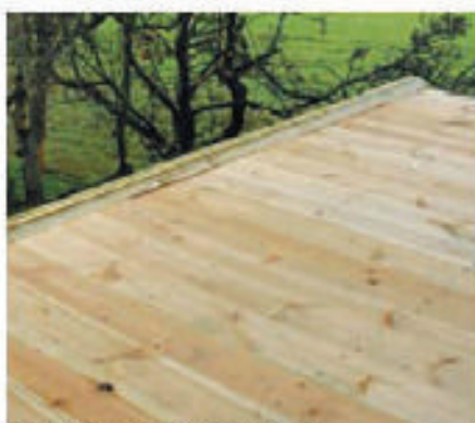
23 Nail angled fillets to the roof edges to slope the felt upwards
