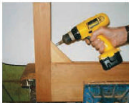
12 Drill clearance holes and screw each block.
