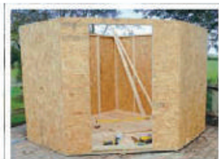
8 The boarding is complete; the window openings will be cut later
