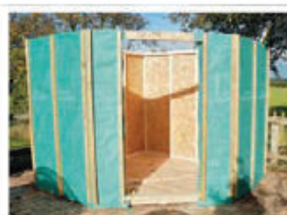
10 Fix treated vertical battens to the studs, with two at each corner
