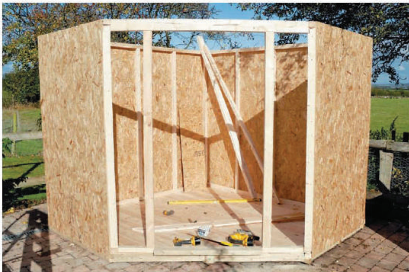
7 The head plate above the door takes the weight of the projecting canopy
