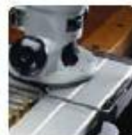
Vacuum box glides with router on beam.
