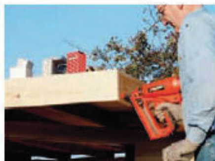
20 Nail the bargeboards into place; a nail gun saves a lot of time
