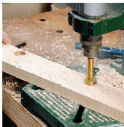
Counterboring the holes for the heads of the coach bolt
