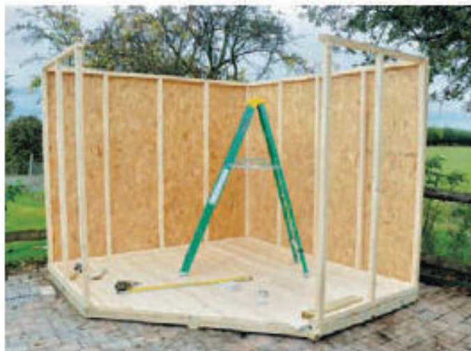
6 ...but fitting the sheets of OSB really stiffens up the structure
