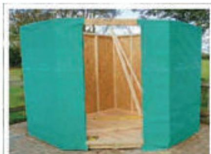
9 Staple the breathable roofing felt to the walls all round
