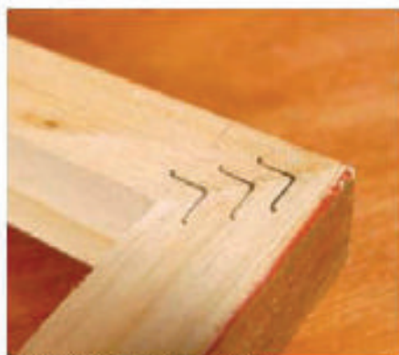
9 One of the pinned frame joints; three nails give a strong joint
