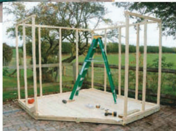
5 Adding the head plates makes the structure reasonably stable...
