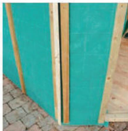
17 The angled fillet for the front corners is an awkward shape to machine
