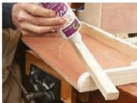
34 Apply glue along each hinge rail
