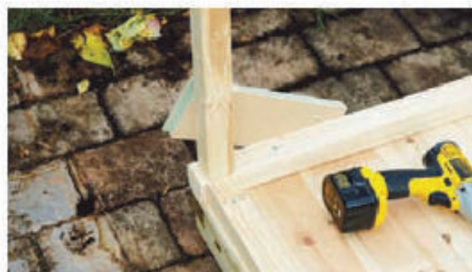
4 Fit temporary supports to keep the corner studs vertical
