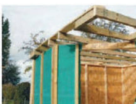
12 ... and fit one at each side of the building with joists in between
