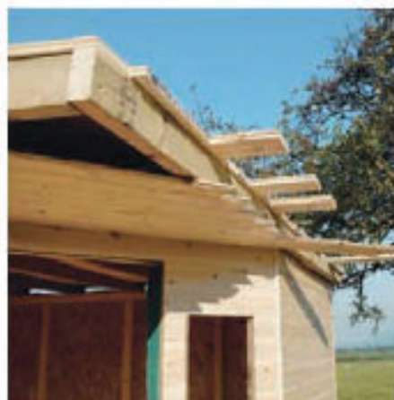
19 Add the tongue-and-groove roof boards and clad the soffits
