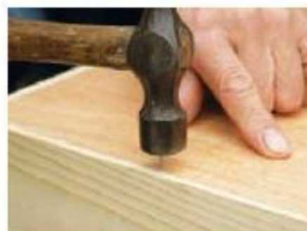
22 Pin the panel into the recess
