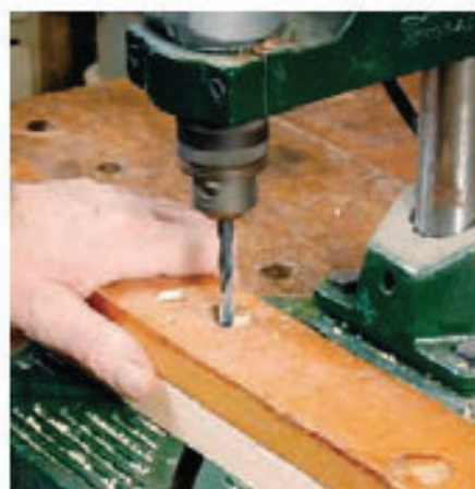
Using the old lippings as templates for drilling the new bolt holes
