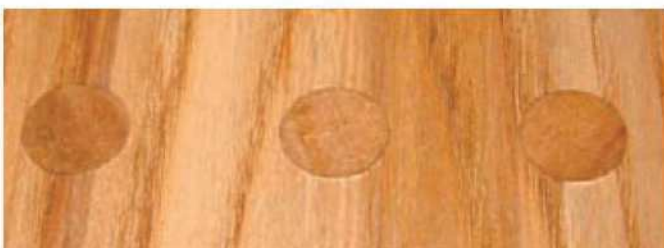
6 Sand the trimmed dowels flush and apply the surface finish
