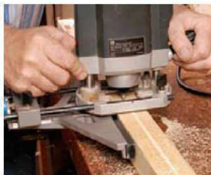
9 Cut the grooves for the polycarbonate sheet with a router
