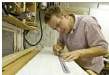
3 Use the pencil marks to position the screw holes on the board
