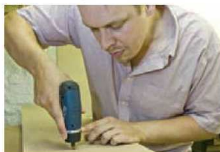
5 Screw the top board to the battens
