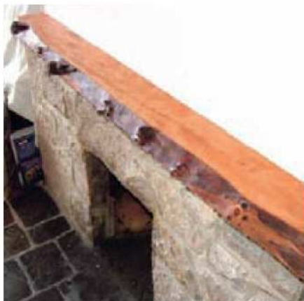
12 I bedded the new shelf in place on a generous bed of PVA adhesive
