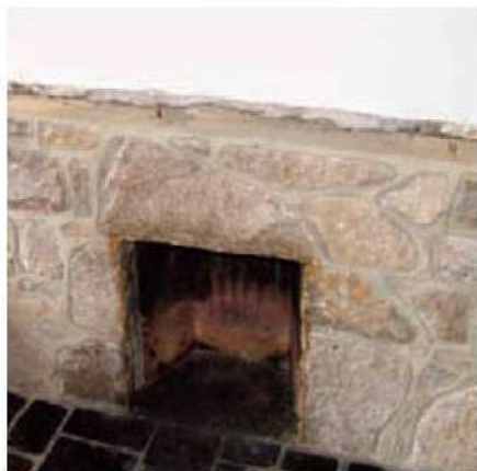
11 The old mantel shelf was held in place with several cut nails
