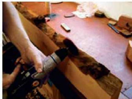
7 An abrasive wheel in a cordless drill cleaned off any edge debris
