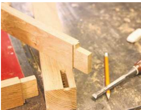
19 Cut the haunches and test for fit
