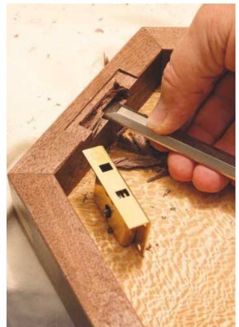
18 A socket is chopped out to house the lock's body in a similar way to chopping a mortise
