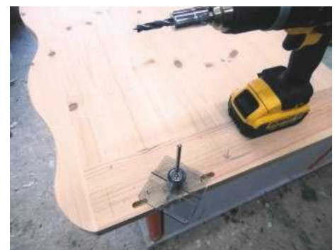
10 Drilling template for the leg bolt hole
