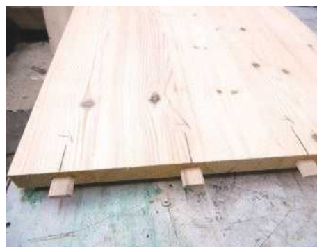
4 Tight Domino mortises in the panel
