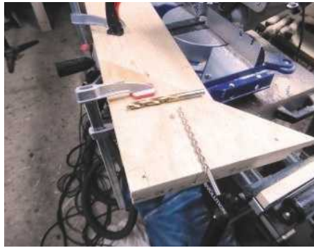
12 Jig for the side rail, dowel nut fitting
