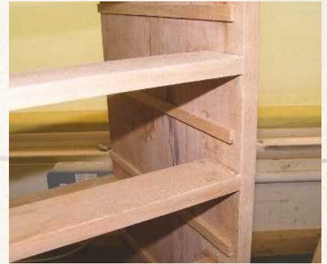
20 Drawer runners were made using thin strips of cherry glued and pinned to the side panels
