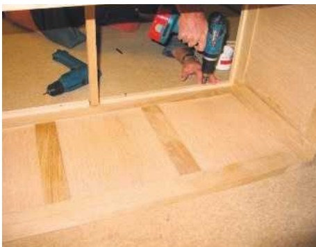
17 A few softwood battens are fixed in place to accept the bottom
