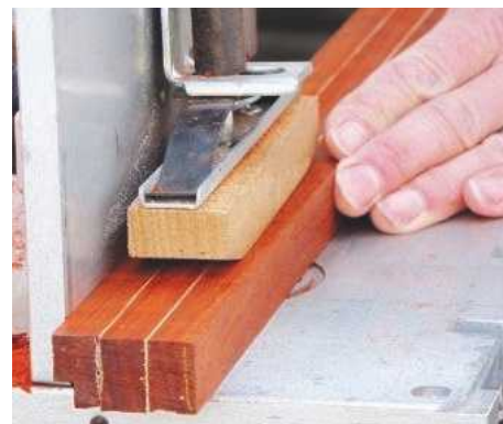
6 Cut a 10 x 7mm rebate on the timber's underside. It's easiest to do this on a router table with a straight bit mounted
