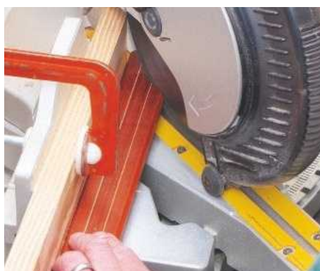
8 Mark the frame pieces to approximate length and saw one end at 45°. Do this on each component
