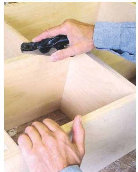
12 A clean-up of the edges with a sharp bench plane completes the job
