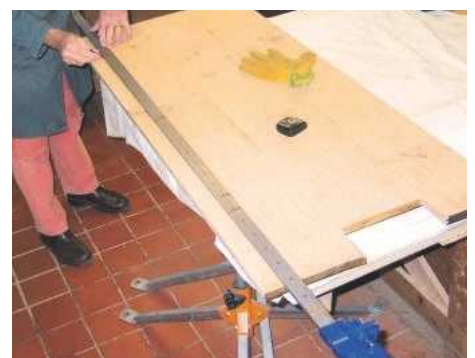
22 A long straightedge is handy for marking the top's finished size
