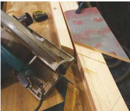
7 Note the use of spare timber to support the saw base
