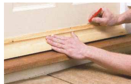
Fitting a weatherboard to a door
