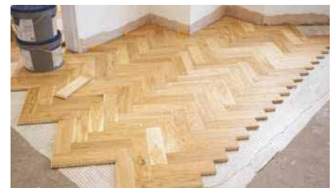
Laying herringbone parquet flooring
