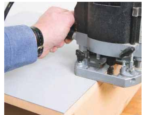
10 Use a bearing-guided cutter to trim the laminate all round...
