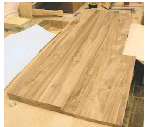
18 The next step was to prepare the solid sections for the laminated doors
