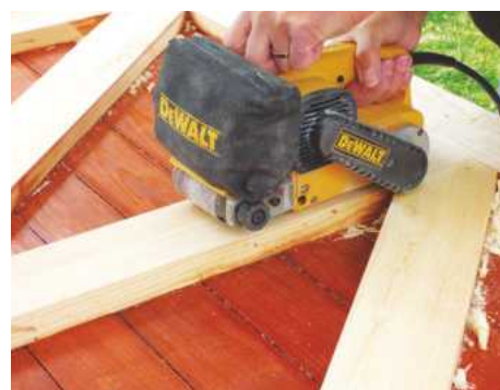
30 Fill all nail holes and any timber defects. Sand both sides of the door before routing a small chamfer along the rails and braces
