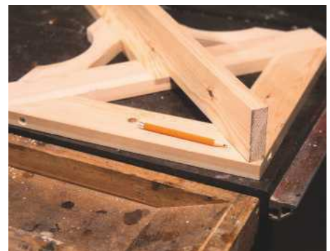
11 Mark out the notch's boundary using a piece of timber, ensuring it's centrally located
