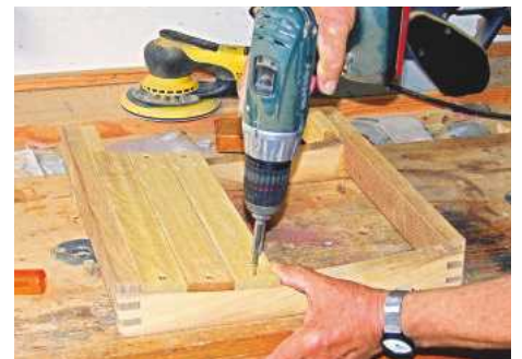
11 prepare the seat slats and drill to accept 4 x 25mm countersunk screws, then screw in place
