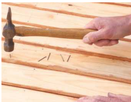
25 Slide the boards into place and mark rail positions ready for nailing. Fix with lost head nails, punching these below the surface
