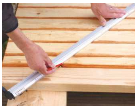
29 Mark out both brace positions across the matchboard. Nail through the boards into the braces and punch below the surface
