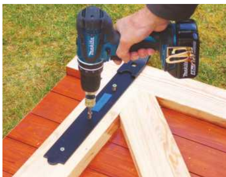
31 Position hinges on the top and bottom rails, then mark out. Drill and screw to the gate with 5.0mm screws
