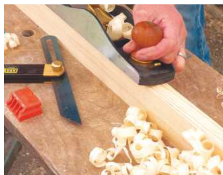
11 To allow rain water to run off, plane a bevel along the top edge of each horizontal rail. This angle should be about 5°
