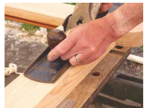
24 Ensuring the gate is cramped securely, clean up both faces with a long bench plane, checking for true with a straightedge
