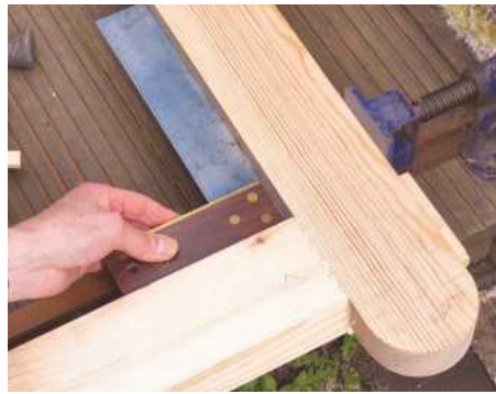
14 Check for square as you cramp the gate together, ideally measuring across the diagonals. Hammer wedges into each tenon
