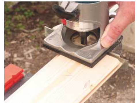
21 The top rail's underside is also grooved to accept the matchboard. Rout rebates along the top edge of each board
