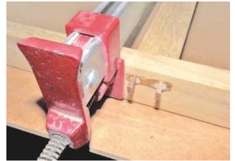
8 Check for squareness and insert wedges into the tenons
