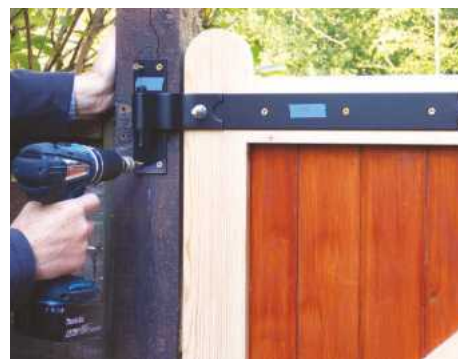
33 Wedge the gate in the opening and mark pin positions on the post. Drill and fix in place with 5.0mm screws
