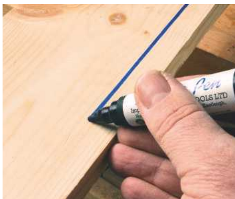
2 Basic marking out can be as simple as a felt pen guided by fingertips to produce a straight line parallel to the edge
