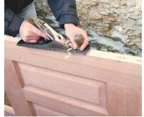
5 Mark both edges with a gauge and plane the door to width. Remove an equal amount from each side
