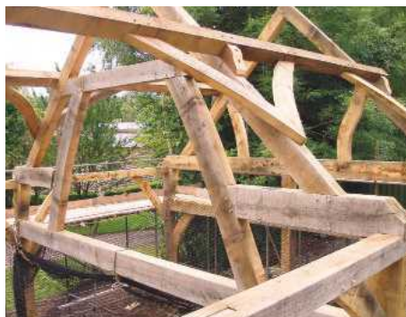
Traditional oak barn construction
