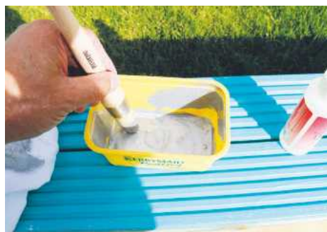
A sparse amount is needed; a small squirt of Extender allows for a longer working time
