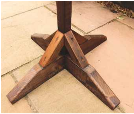
10 The post is supported by four lengths of 2x2in, screwed to both base and post
