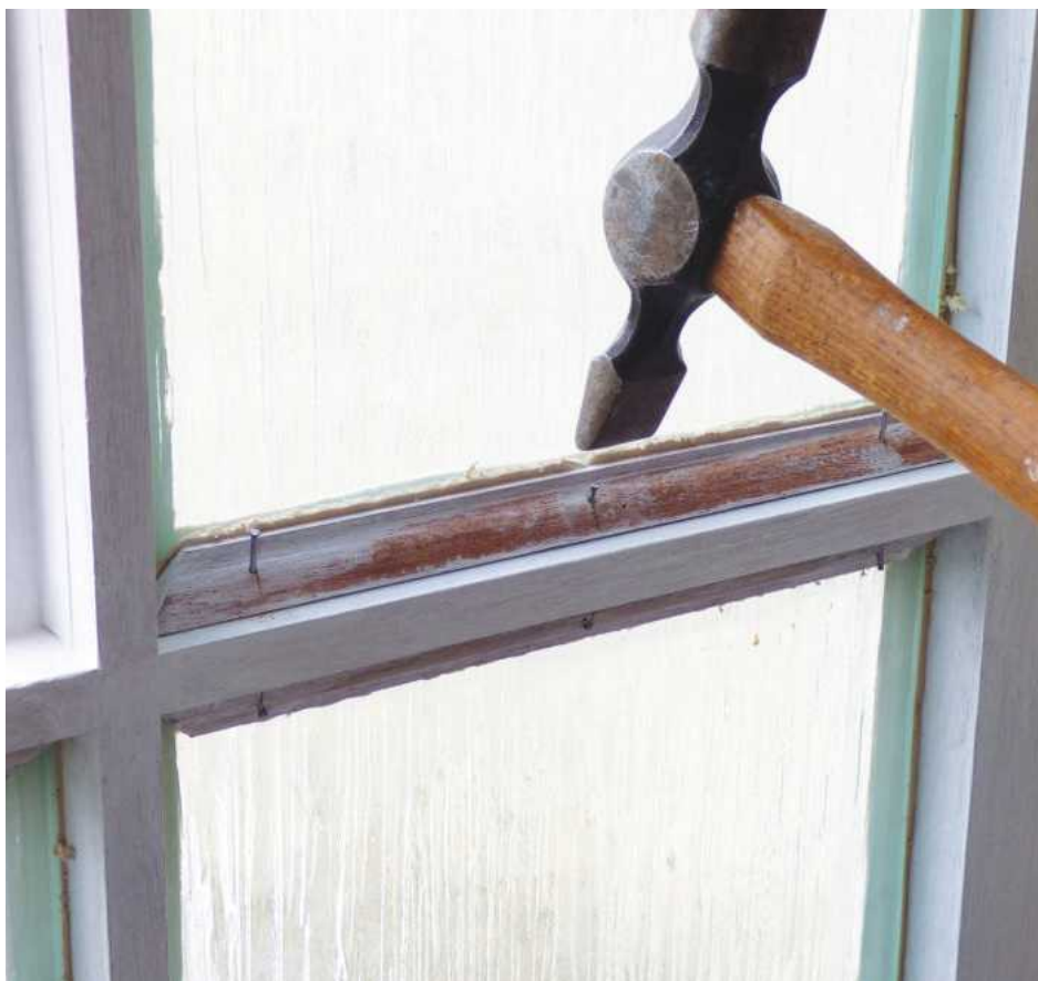
23 Putty the back of each beading strip and push against the pane. Carefully pin the beads, pre-drilling the ends to prevent splits ✂
