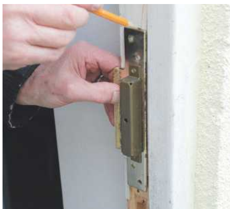
19 Screw lever handles to the door. Mark the striker box against the jamb, drawing around it in the new position
