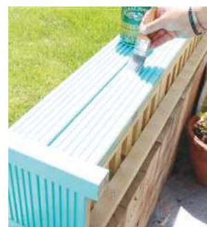
An external top coat is applied to seal the surface, ready for the Pearl Effects
