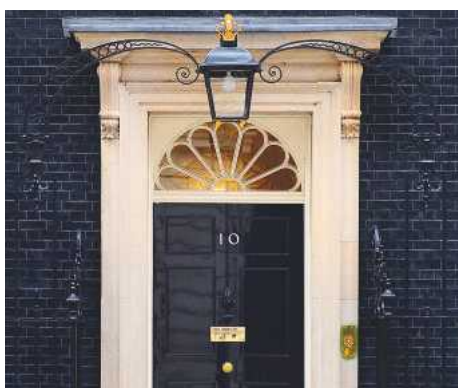
A transom is a transverse horizontal structural beam or bar, or crosspiece, which separates a door from the window above it
