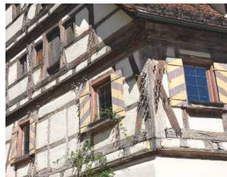
Treenails used in timber framing of a former cooperage and monastery cellar from 1478 at Blaubeuren Abbey
