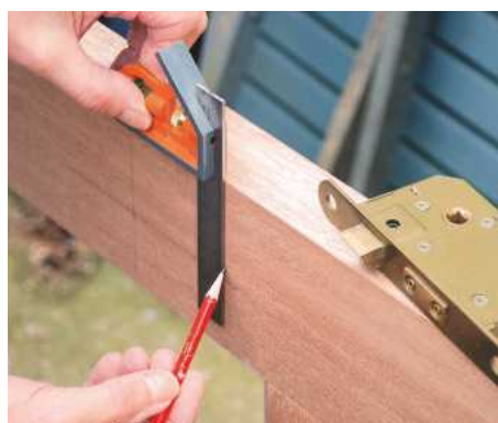
13 Next, mark the lock position on the door edge, transferring spindle and keyhole heights to both faces
