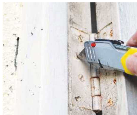
2 Old hinges are often caked with paint, so clean out slots with a craft knife or screwdriver before removing the door
