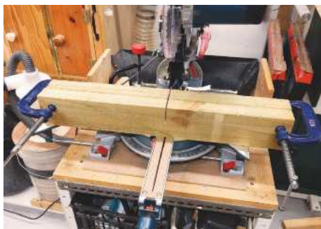
1 Trench-cutting the cross-lap joint on the 4×2in base pieces
