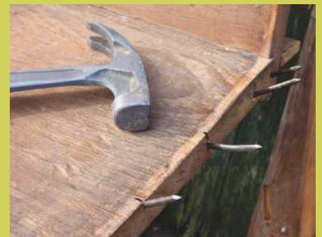
One or two hefty screws had been used, but the pieces came apart easily with little damage
