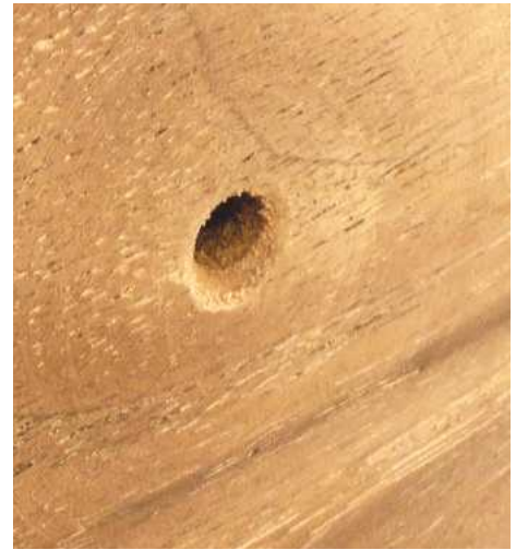
33 The hole in the top can be rounded over slightly so that you don't experience any chafing of the string. Sand the top to a very fine finish and take care not to leave any scratches on the surface, as these stick out like a sore thumb on walnut
