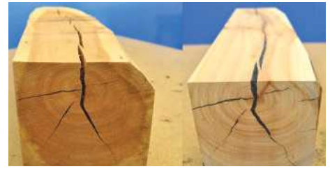
The split on this piece of wood – left – was filled with polyester resin, put aside to cure and repaired structurally – right
