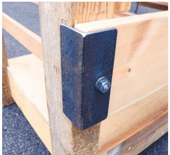
4 A longitudinal brace across the two back legs is glued and permanently clamped in place, with a bolt and steel plate to spread the load
