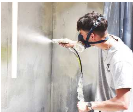
Spraying components using an air-assisted aerosol sprayer
