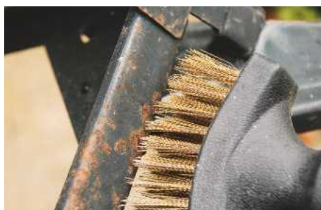
14 Remove springs and rubber feet from the folding legs. Clean off heavy rust using a wire brush or sanding. Get into crevices with an old toothbrush
