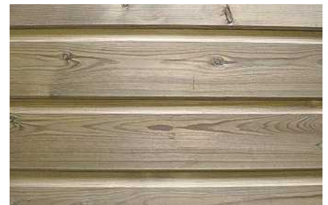
Shiplap is a tongue & rebated board – 12 x 120mm
