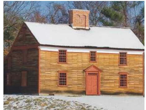
Captain William Smith House at Minute Man National Historical Park – a restored saltbox style house with unpainted clapboard siding
