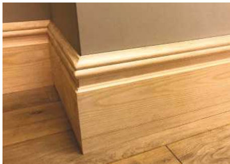
Large Victorian skirting board – 8.5in deep
