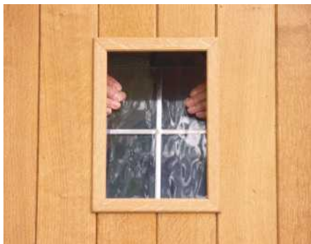
7 Check the glass for size. Run a bead of glazing sealant around the inside rebate and then insert the glass
