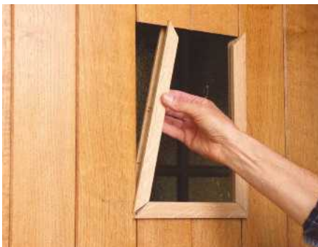
6 Continue to fit the remaining pieces, ensuring the mitres are tight. Check for accuracy with a small square
