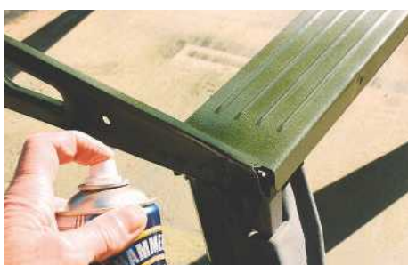
16 Spray two or three coats of your chosen colour, allowing at least 15 minutes between each if using aerosol. Work in a ventilated area and wear a mask
