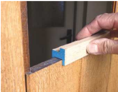
3 Try an offcut in the opening, adjusting groove depth and width if required. It should be a sliding fit
