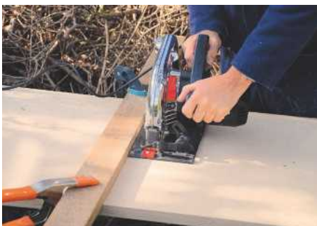
4 If you don't have a table saw, cut the ply to size with a circular saw. Cramp a length of timber to the board to act as a straightedge
