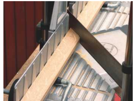
5 Measure the opening and cut the first frame piece to length. Try it in position and trim if necessary
