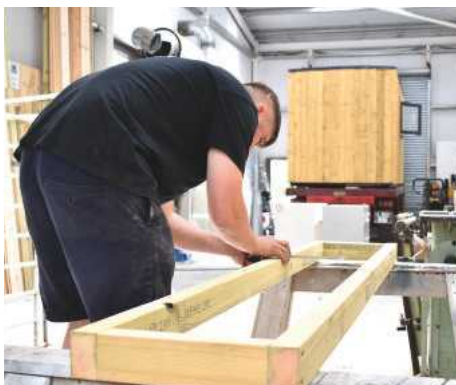
Using softwood timber stock, construction gets underway
