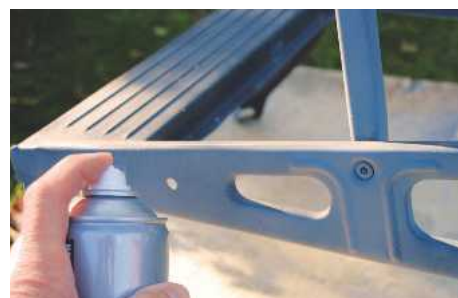
15 Cover plastic locking levers that cannot be removed with masking tape. Brush away dust and dirt, then wipe over with white spirit. Apply primer
