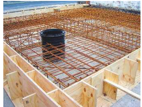
Concrete shuttering by B A Boyle & Son
