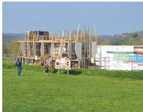
March 2019 – construction is coming along steadily
