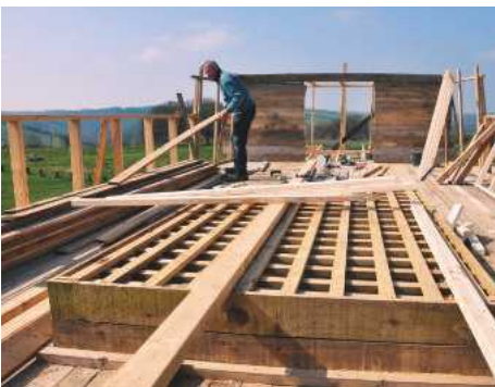
March 2019 – construction of the main deck with grating visible
