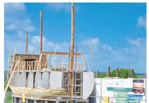
Hull progress as of April 2018
