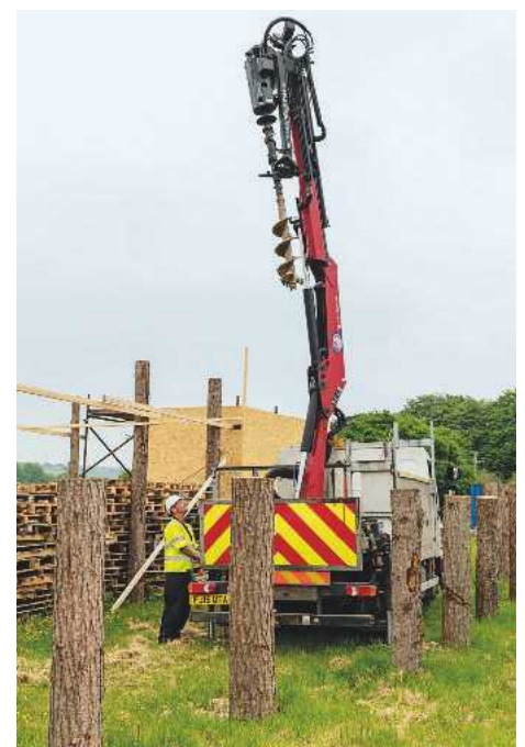
BT Open Reach drill holes for the 40ft logs that will support the 5ft platform. Mast holes are also drilled
