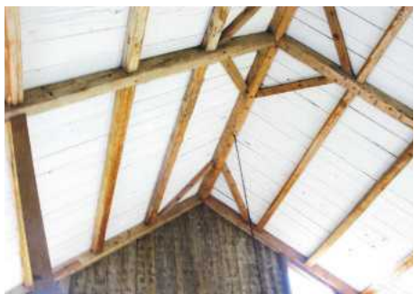
View of a roof using common purlin framing. The purlins are the large beams perpendicular to the rafters
