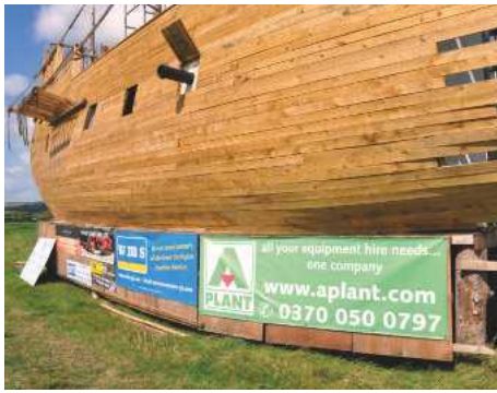
Construction progress as of August 2019. Gun ports are visible with cladding required just to the bow
