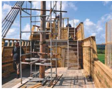
Extensive work has been carried out on the stern end of the ship up to the poop, half and upper decks
