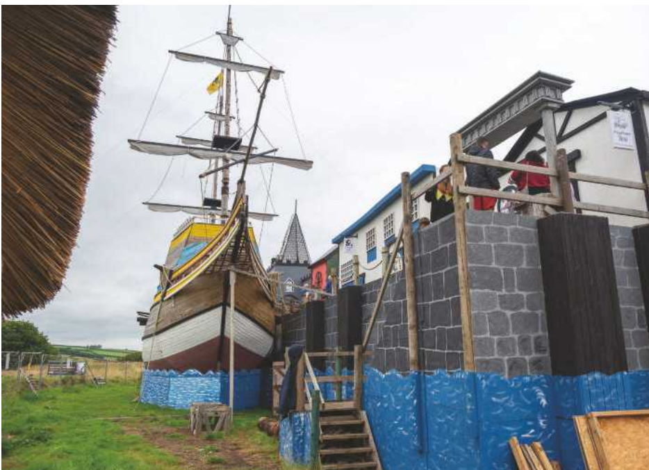
Work is now completed. Here you can see the steps from quayside to the ship
