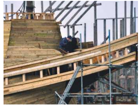
Beak head under construction and the quayside is starting to take shape
