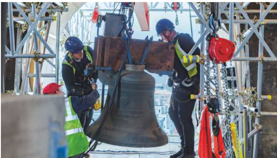
One of the 12 Bells of St Paul's being removed from the bell chamber opening Photograph courtesy of The Worshipful Company of Turners
