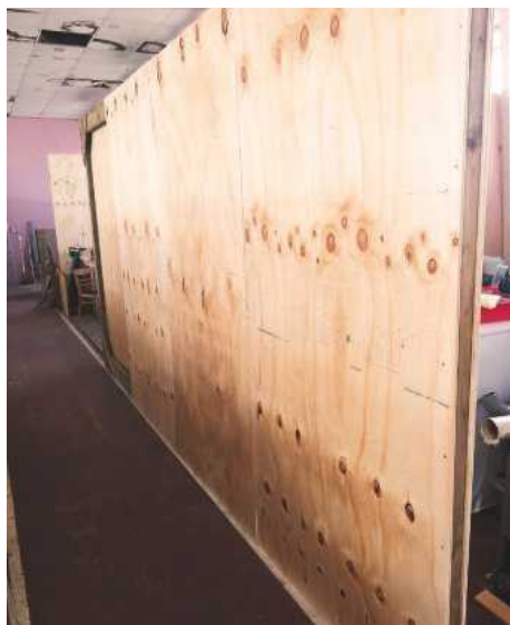
3 The middle wall, once constructed
