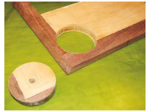
4 Cutting an internal radius in the corner of the upper octagon's bottom frame
