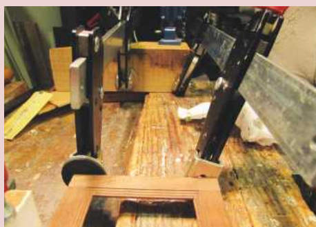
8 In this case, the frames are compressed while glued joints set
