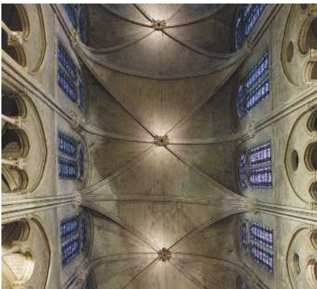
The nave's early six-part rib vaults. Ribs transferred thrust of the roof's weight down and outwards to pillars and supporting buttresses
