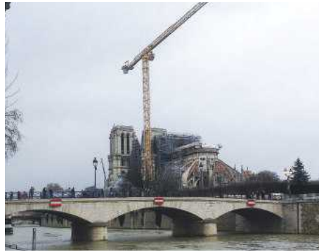
Stabilisation of Notre-Dame and removal of roof debris and scaffolding (29 February 2020)
