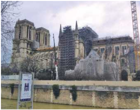
Ongoing stabilisation of Notre-Dame (29 February 2020)
