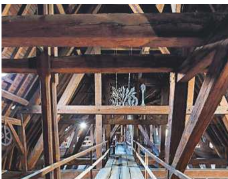
The framework holding up the cathedral's roof, known as 'the forest'
