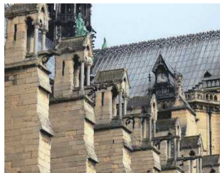
The massive buttresses, which counter outward thrust from the nave's rib vaults. The weight of the building-shaped pinnacles helps to keep the line of thrust safely within the buttresses
