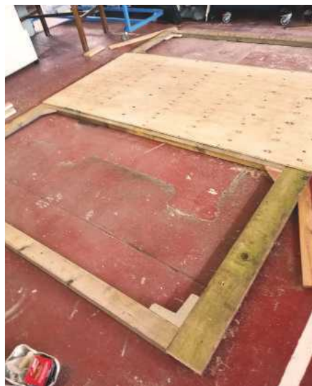
4 Construction of a wall
