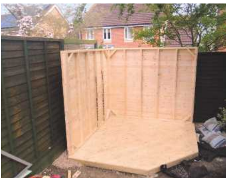
7 First walls in place
