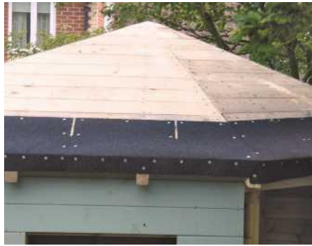
20 First row of shingles
