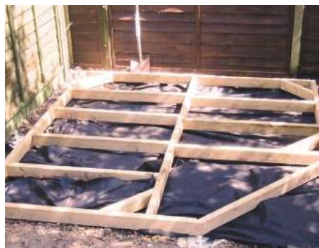
5 Final levelled base
