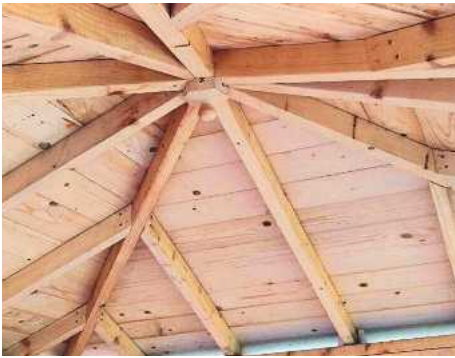
19 Roof fitted – internal view
