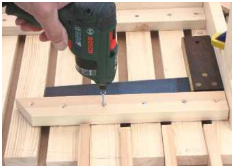
17 Cut two shorter battens to support ends of the slats; mitre the ends and screw into position
