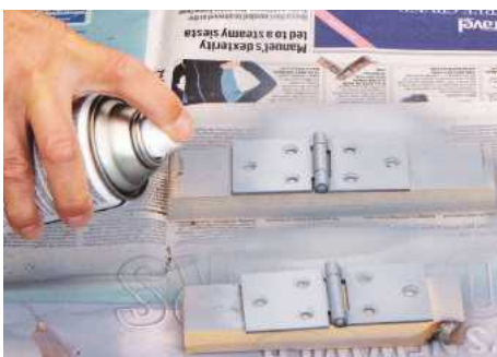
23 Remove the hinges and spray with primer to prevent the steel rusting, followed by exterior paint
