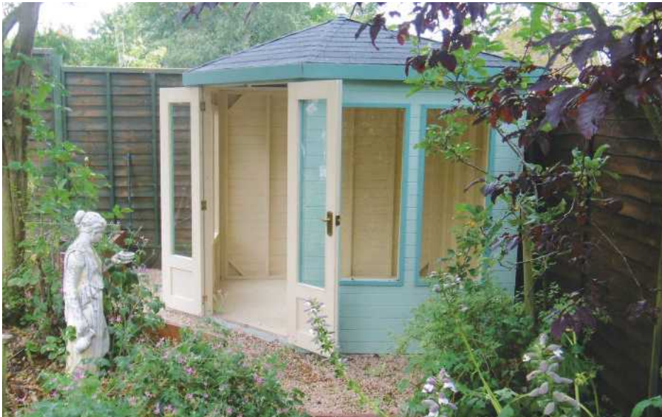
23 The completed summerhouse with cathedral roof
