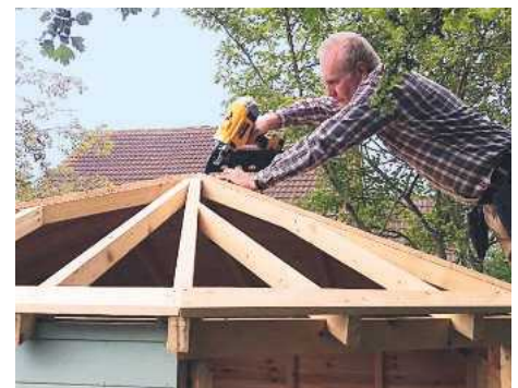
18 Roof in progress
