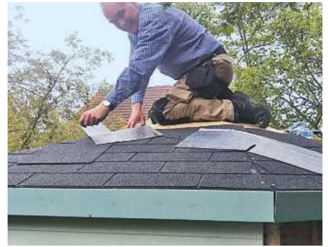
21 Working on the roof
