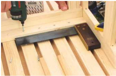
14 Cramp frames to slats and cut the support batten; screw across slats, checking for square
