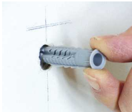
5 Insert rods into the rear of the shelf and mark screw tips against the wall. Using a masonry bit, drill 10mm holes for the plastic plugs provided
