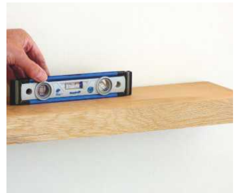
9 Check the shelf with a spirit level. The advantage of BespOak brackets is they can be adjusted with a spanner to get the timber dead level
