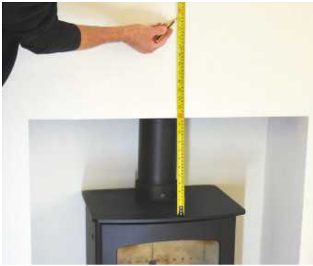
1 Mark the height of the mantelshelf on the wall. Combustible building materials (such as timber) must not come within 300mm of a woodburner
