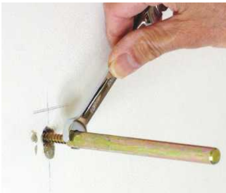
7 Insert a bracket into each plug, driving it home with a 10mm spanner until the end of the rod is tight against the wall. Then allow the resin to dry
