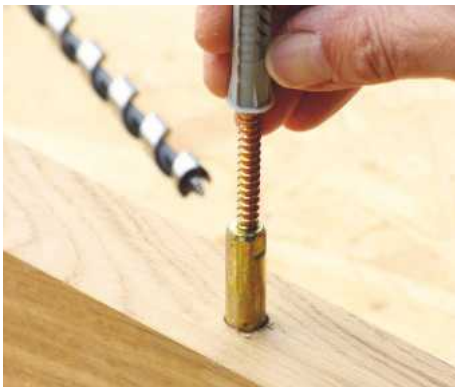
4 Remove debris and check drilling depth by inserting a bracket into each hole. Tape around the bit acts as a guide to warn you if drilling too deep
