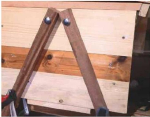
14 Bolting the legs in place
