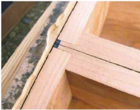
11 You can see where the cutter nibbles into the template
