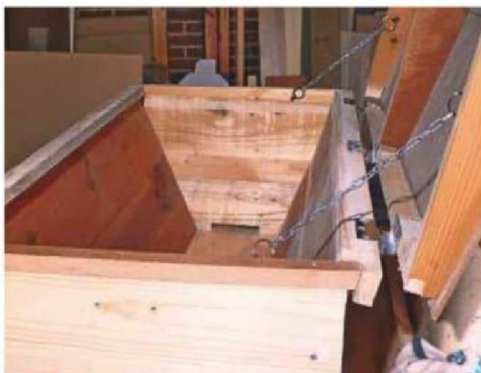
16 Roof chains on reinforced back
