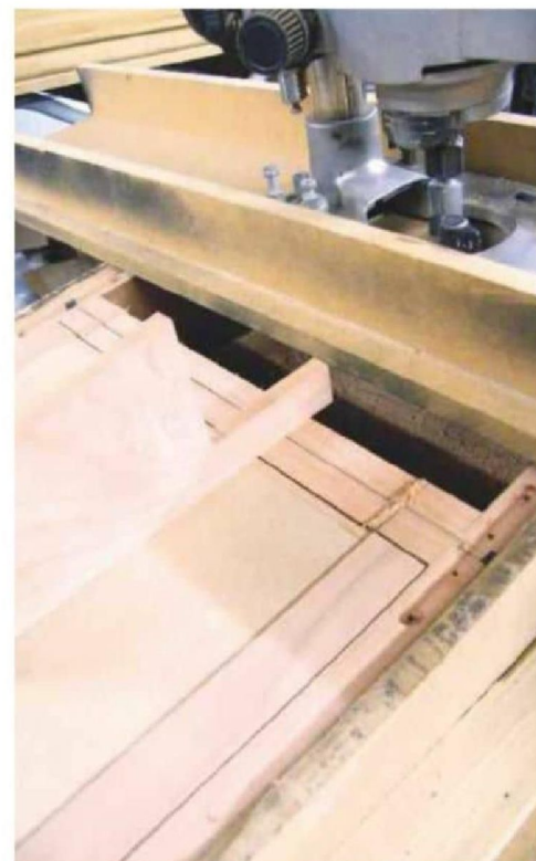
24 Check the slope is level with the recess
