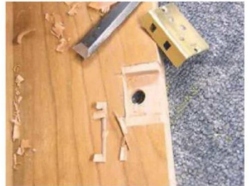
14 A sharp chisel is used to fit the lock
