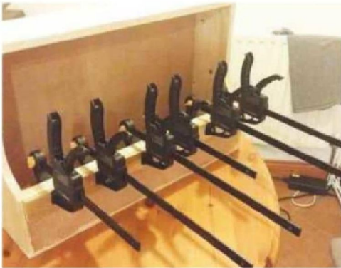
16 The bottom hinge rail, cut and glued in
