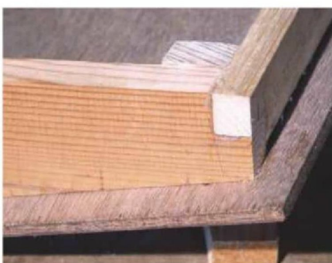
8 Half-lap joints in the roof frame
