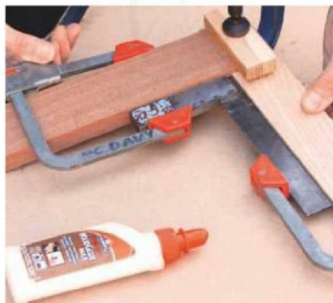
14 Brush PVA on the joint and cramp together. Cramp an accurate square in position while the glue sets
