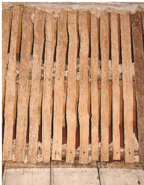
Lath and plaster work
