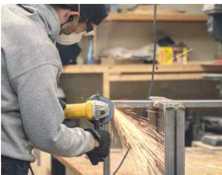
20 Using the angle grinder to clean up my welds
