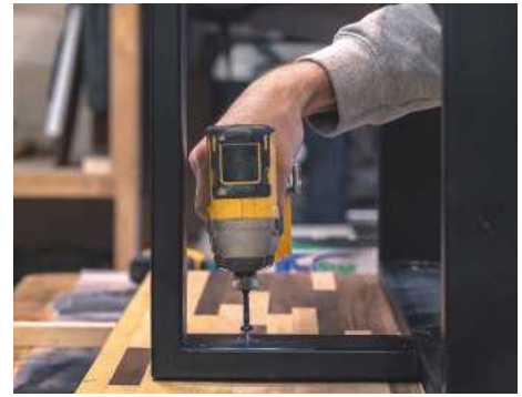
25 Drilling the five holes in the leg assembly to take 38mm long No.10 screws
