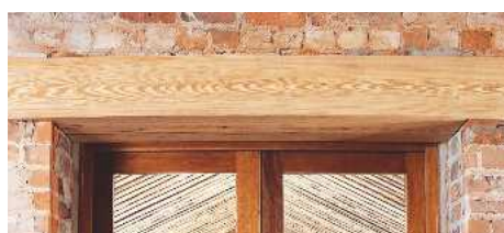
A wooden lintel
