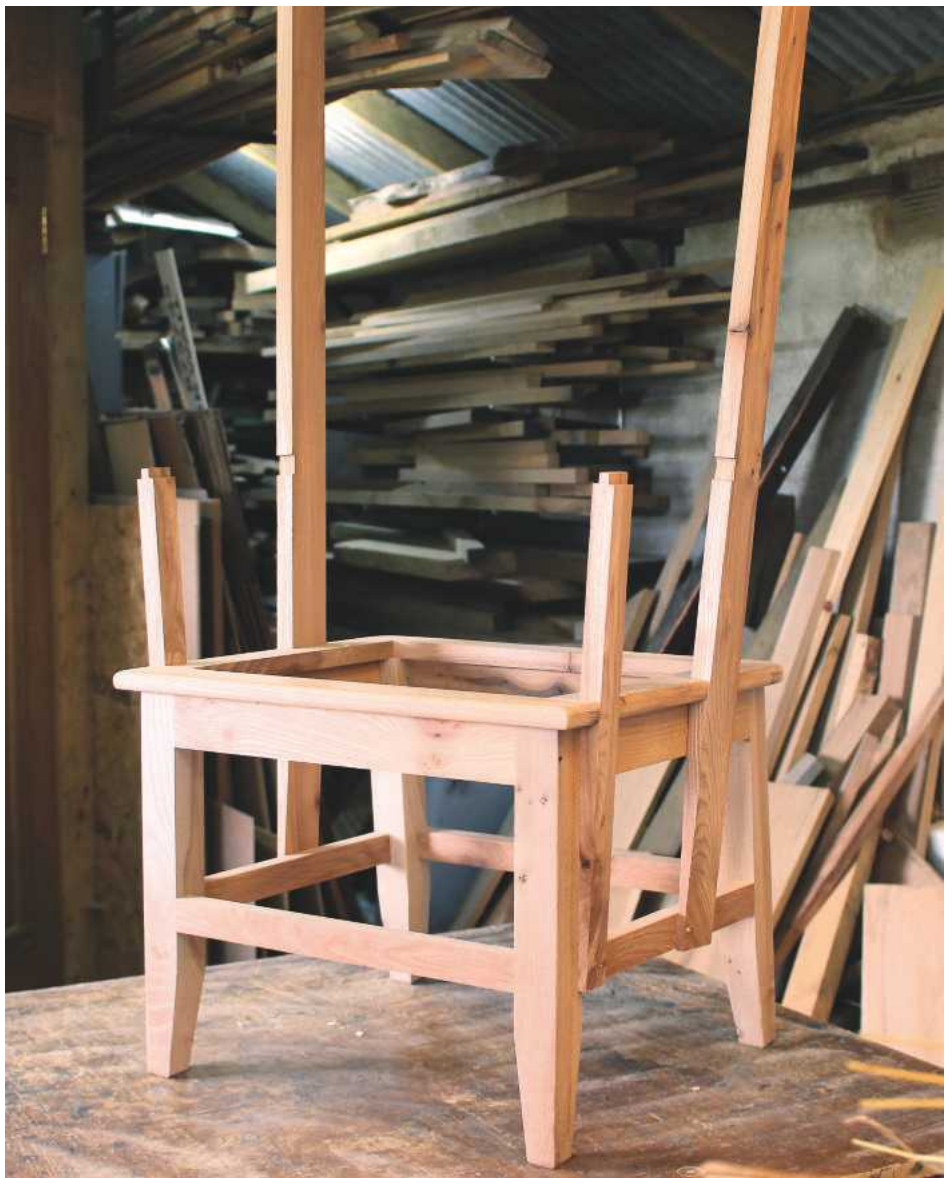
12 The uprights are temporarily attached
