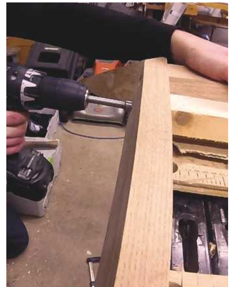
31 Recesses drilled for the connector bolt heads
