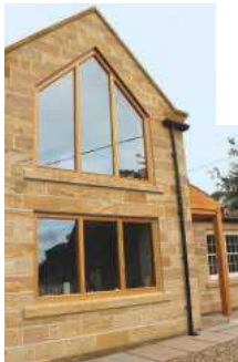
Oak gable end frames by S Taylor & Son Ltd
