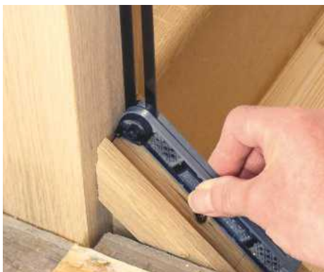
25 Check the angle between the capping and newel with a sliding bevel. You'll need this angle to cut the bevells accurately on each fillet
