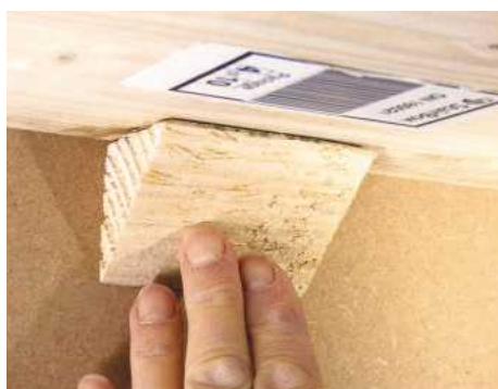
19 Glue blocks underneath the treads and risers add strength and help prevent the stairs from creaking when walking up and down
