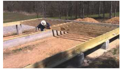
Laying out floor joists
