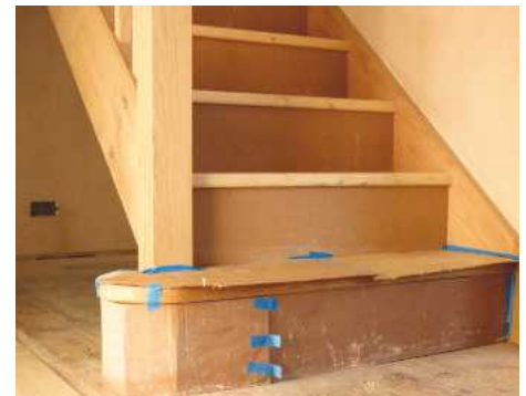
45 Protect oak surfaces temporarily with cardboard if there's likely to be other building work going on before finally finishing the stairs
