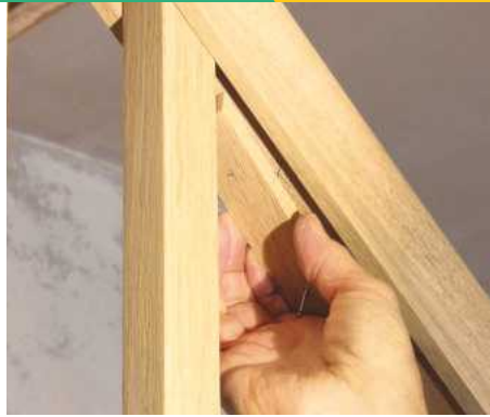
38 Cut and fit matching fillets to the underside of the handrail. You may find a nailgun easier here rather than hammering panel pins upwards
