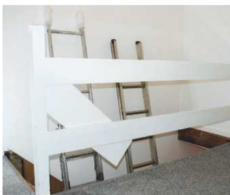
4 The landing balustrade is straightforward to remove with a handsaw. Newel posts can be sawn off and levered out where fixed to a wall
