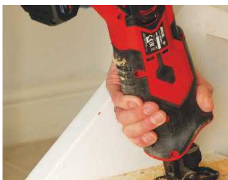
2 Begin by removing the treads. The safest way is to cut through them with a recip saw, starting at the top and working your way down
