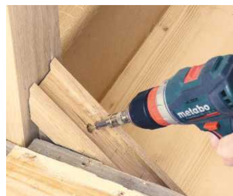
24 Spindles are seated in a capping rail that runs up the outer string, already cut to length at the correct angle. Drill and fix with 5 x 50mm screws
