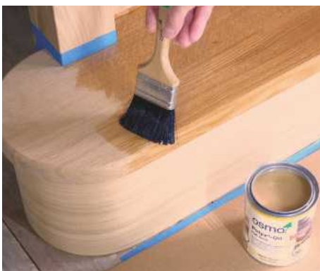
46 Vacuum surfaces after final sanding, then brush on two coats of Osmo Polyx Oil (semi-matt). Lightly denib once the first coat is dry
