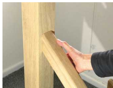
33 Carefully lower the handrail so that it clicks into place. Alternatively, use Zipbolts so that the handrail can be removed fairly easily
