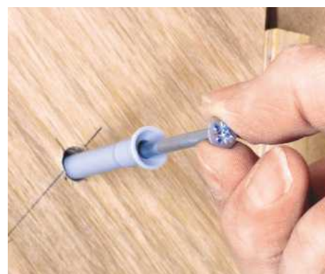
18 Insert hammer fixings through the string and tap them home with a hammer. These can be removed again with a screwdriver, if necessary
