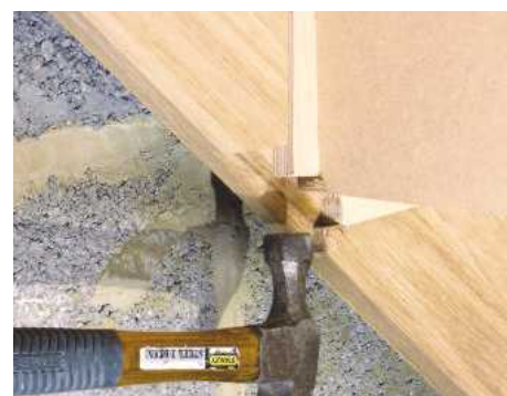
21 The bottom two steps will still need wedging and gluing. Coat with glue, then tap loose wedges into the strings on either side
