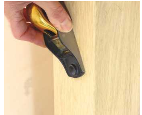
42 Fill any remaining screw holes in the newels with matching oak plugs. Glue and tap in place, then trim flush with a block plane
