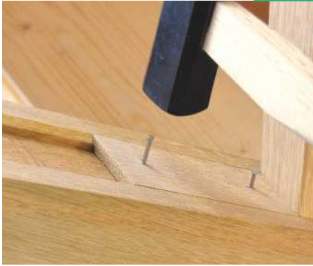
37 Pre-drill fillets for 25mm panel pins, apply glue and carefully nail to the capping rail after installing a spindle. Punch heads below the surface
