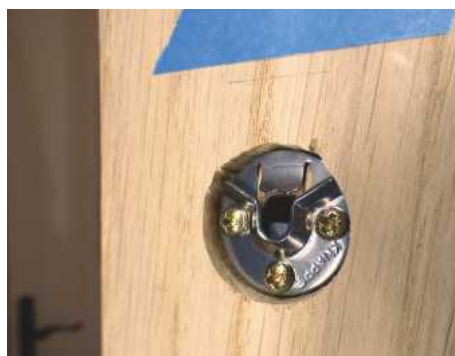
32 Screw the steel plates in place. These consist of sprung sockets to receive screws that are fitted at the ends of the handrail
