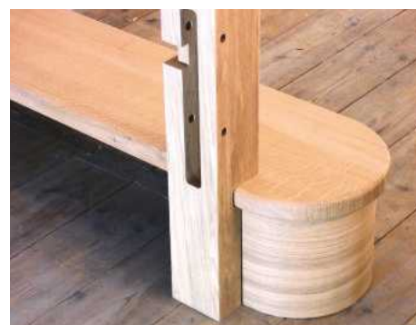
9 Most of the stairs will be carpeted, apart from the bottom half-round step, which is oak. Check the newel fits before installing the actual flight
