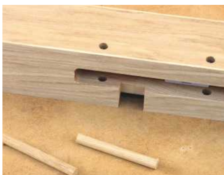
7 Mortises in both top and bottom newels are draw-bored. Tenons at each end of the string are pre-cut and should be a sliding fit into the newels
