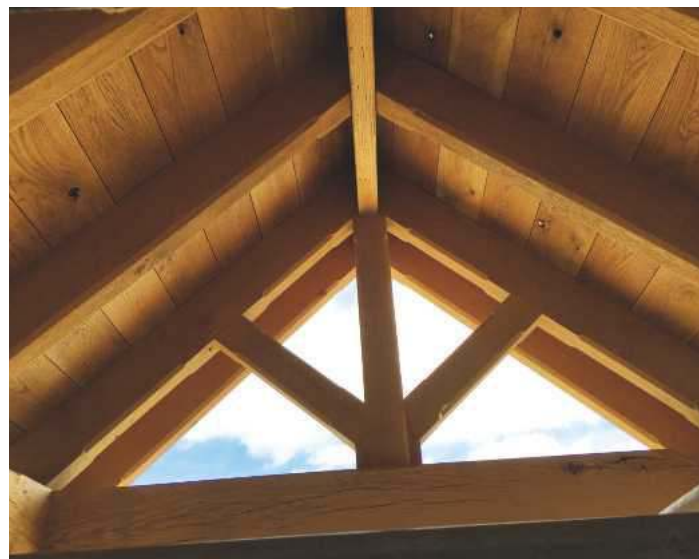
Porch. He is more than capable of conventional carpentry, though a job this size requires another pair of hands. "With angles and things I need a second brain"
