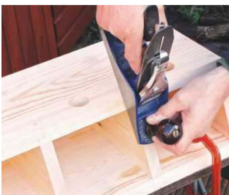
10 Check top edges are flush, trimming with a finely-set plane if necessary; tidy up internal arrises
