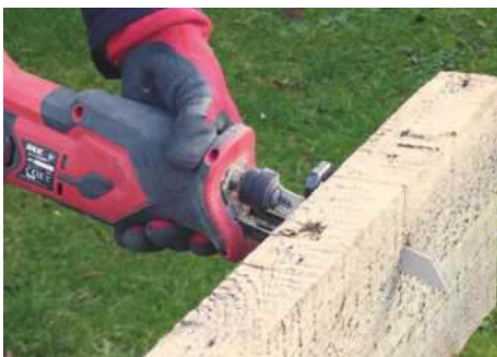
Similarly, cutting through 50mm reclaimed softwood joists was no problem
