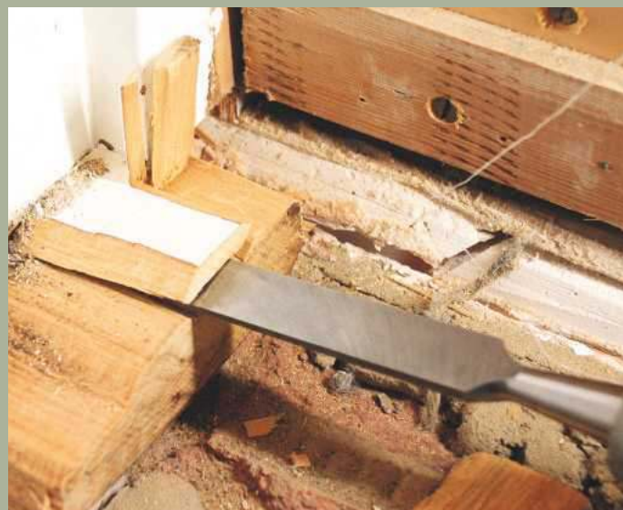
Since then, I've used one chisel to chop out the ends of treads when installing new stairs
