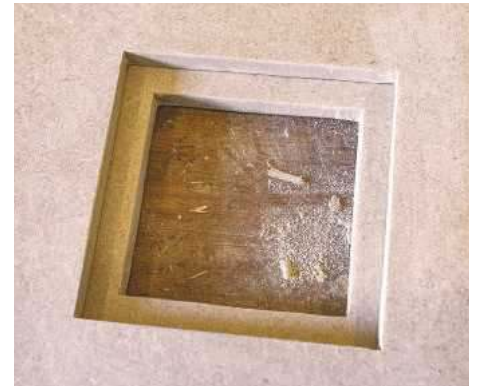
24 The finished stepped opening in the lid
