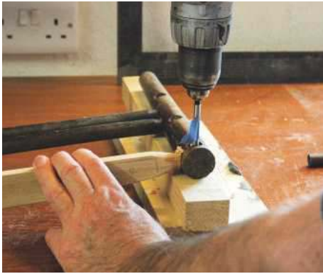
12 Re-drilling the mortises with a 1/2in Forstner, to remove the ends of the new tenons
