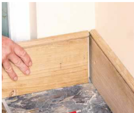
14 Check joints butt together neatly at internal corners. Trim edges carefully as required
