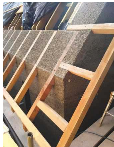
7 'Hempcrete': fibres of hemp bound with lime and cement. A quicker, more precise alternative to cob. Inside the hall, window reveals are rounded as if they were cob, adding vernacular charm and softness
