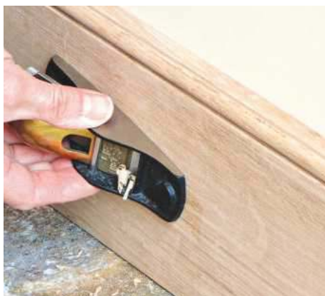
22 Carefully trim plugs flush with a block plane or chisel. Fill any defects and sand the surface
