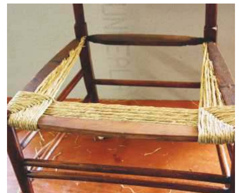
19 Starting off on the wrong foot, with incorrect weave pattern
