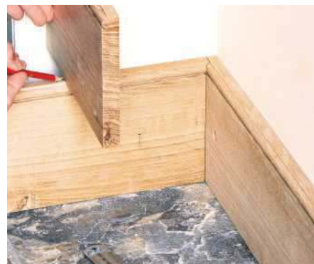
15 Mark external mitres with a pencil by holding the next piece of oak above the existing skirting
