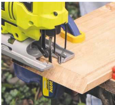
11 For internal corners, mitre the next board at 45°, then cut along the profile with a jigsaw
