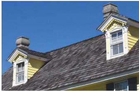
A pair of dormer windows
