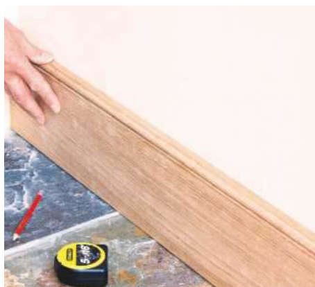
5 Start fitting skirting to a long section of the wall. Cut to length, drill and counterbore for oak plugs
