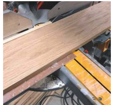
10 Sacrificial plywood on chop saw to ensure perfect cuts
