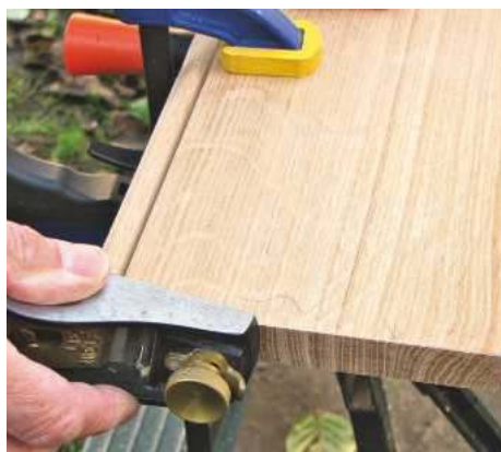
7 Cut the first board to length. If too tight between internal corners, trim sawn ends with a block plane
