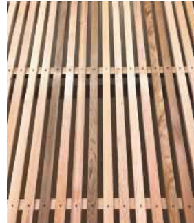
Cedar clad gate, countersunk and screwed with correct spacing
