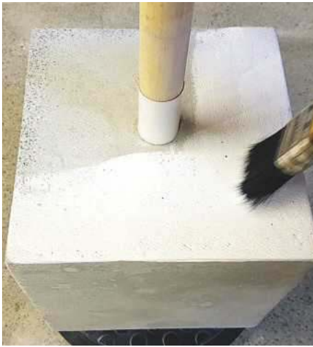
6 Painting the concrete block 'gift box' with an initial coat of white masonry paint
