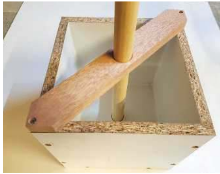
2a Timber dowel and brace in place, ready for the concrete to be poured into the box
