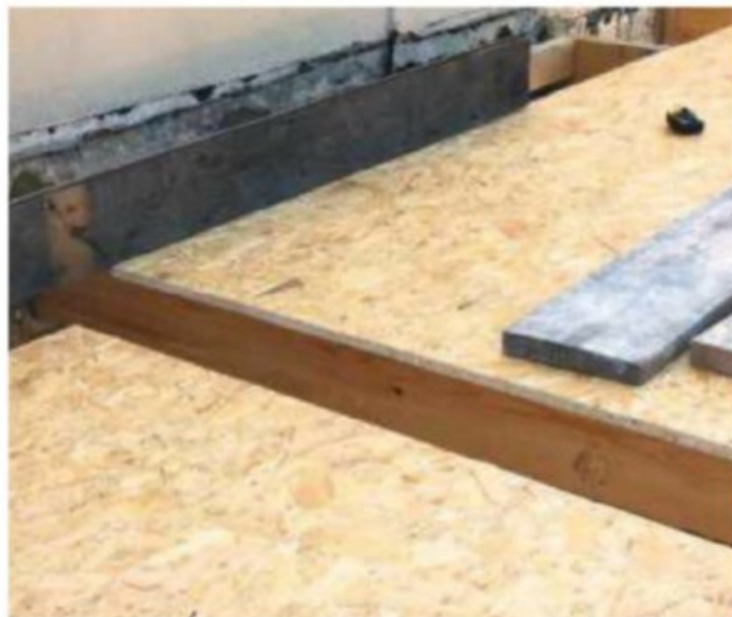
17 Lay the first OSB sheet across the roof, checking one edge is centred along a joist. Sheets should be fixed with markings face down
