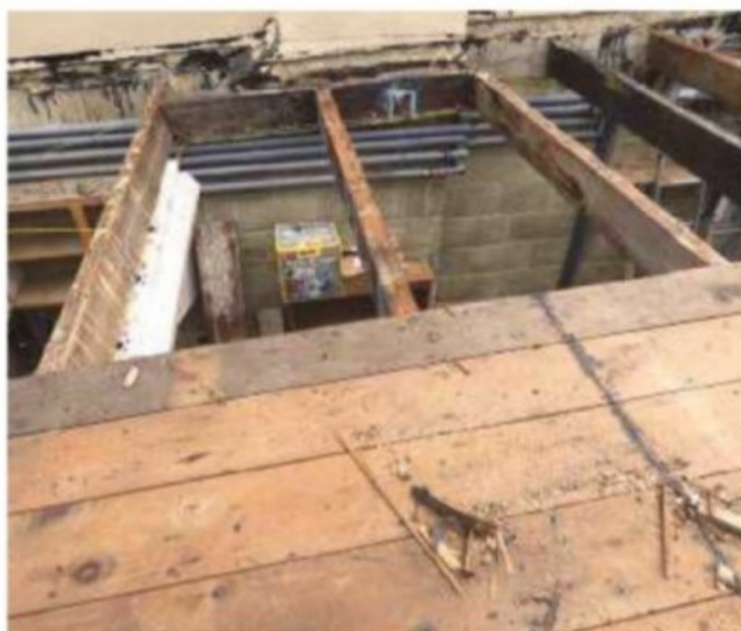
5 With the debris removed you can start removing the deck boards, working across the roof. Make sure you have at least one ladder in place first
