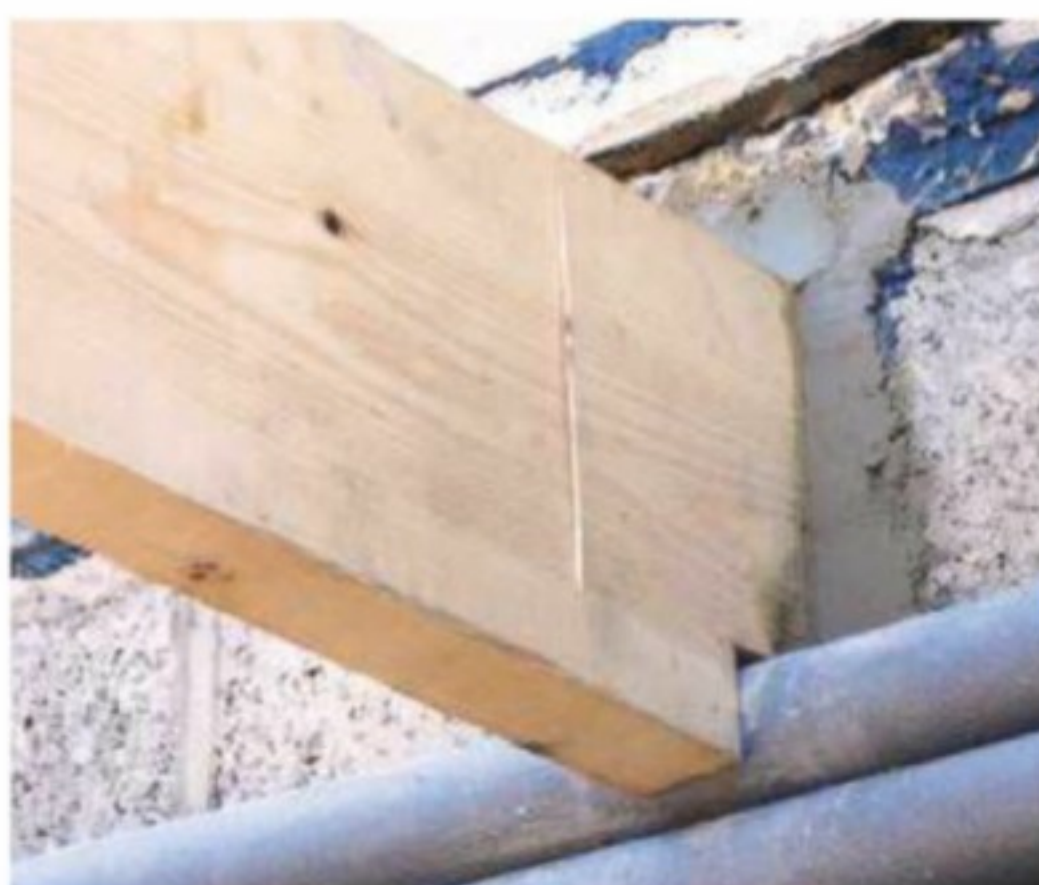
11 Notch joists around pipework or other obstructions. Insert joists into the wall and fill each cavity with mortar once they're finally in position
