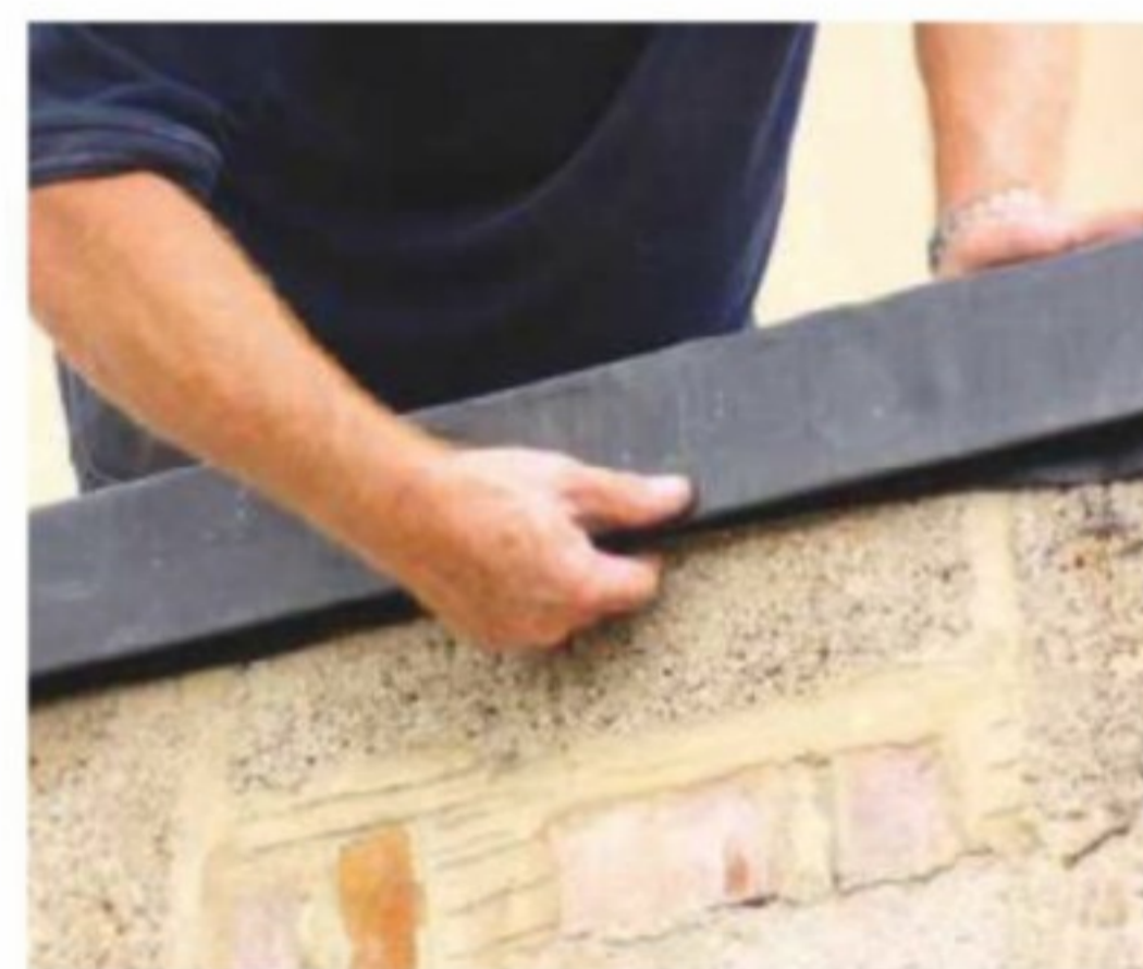
30 An industrial contact adhesive is used to glue the rubber up and over the parapet wall. It's then tightly tucked beneath a horizontal batten
