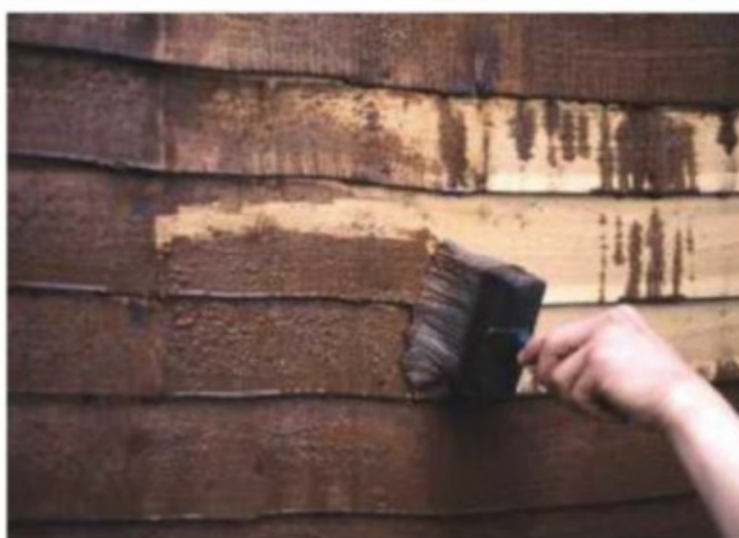
Painting a timber building with creosote
