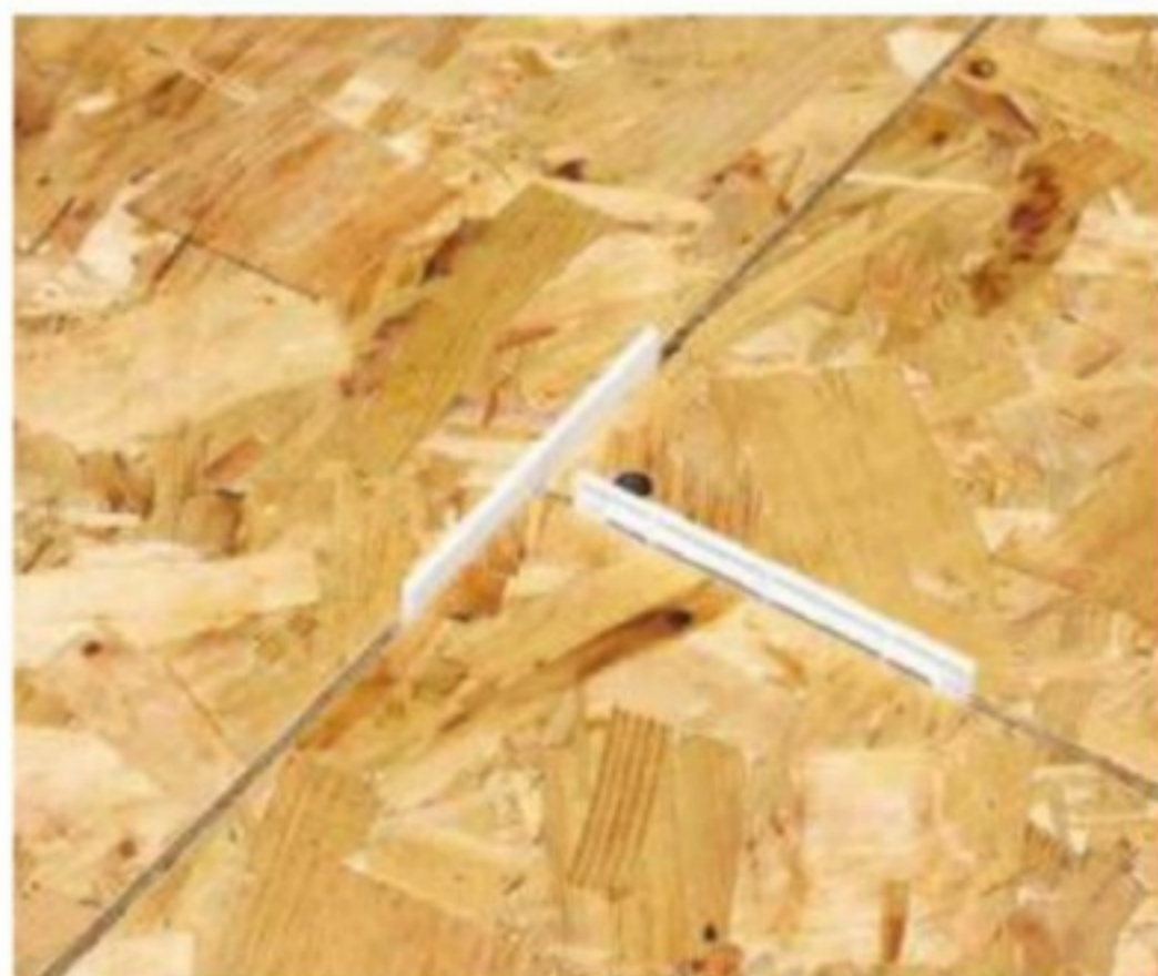
20 Joints should be staggered where the sheets are butted together. To allow for expansion, use 3mm thick spacers between each board
