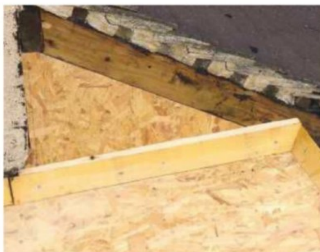
26 The gap at the end of the adjoining roof is filled with a piece of OSB board. Use a sliding bevel to determine the angle for marking and cutting
