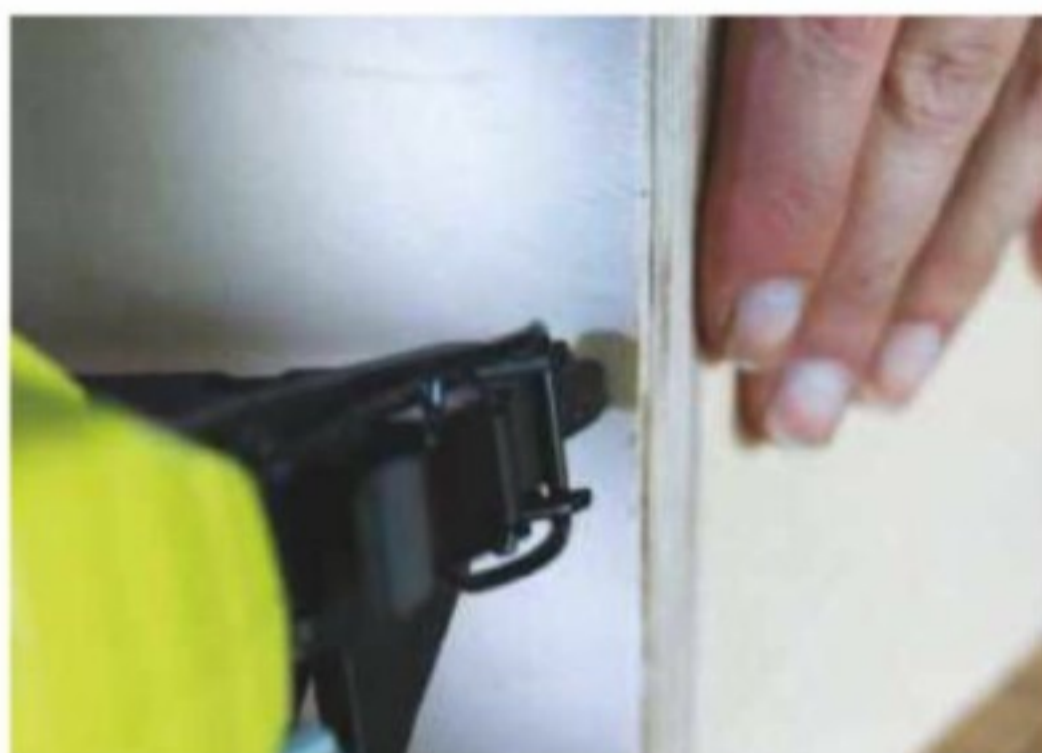
Constructing plywood cabinet components using 30mm nails
