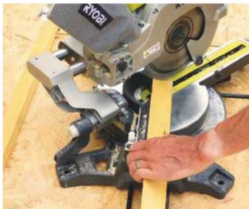
23 Arris rail is fixed around the perimeter of the roof tight to the walls. Cut sections to length with a powered mitre saw or with a hand saw
