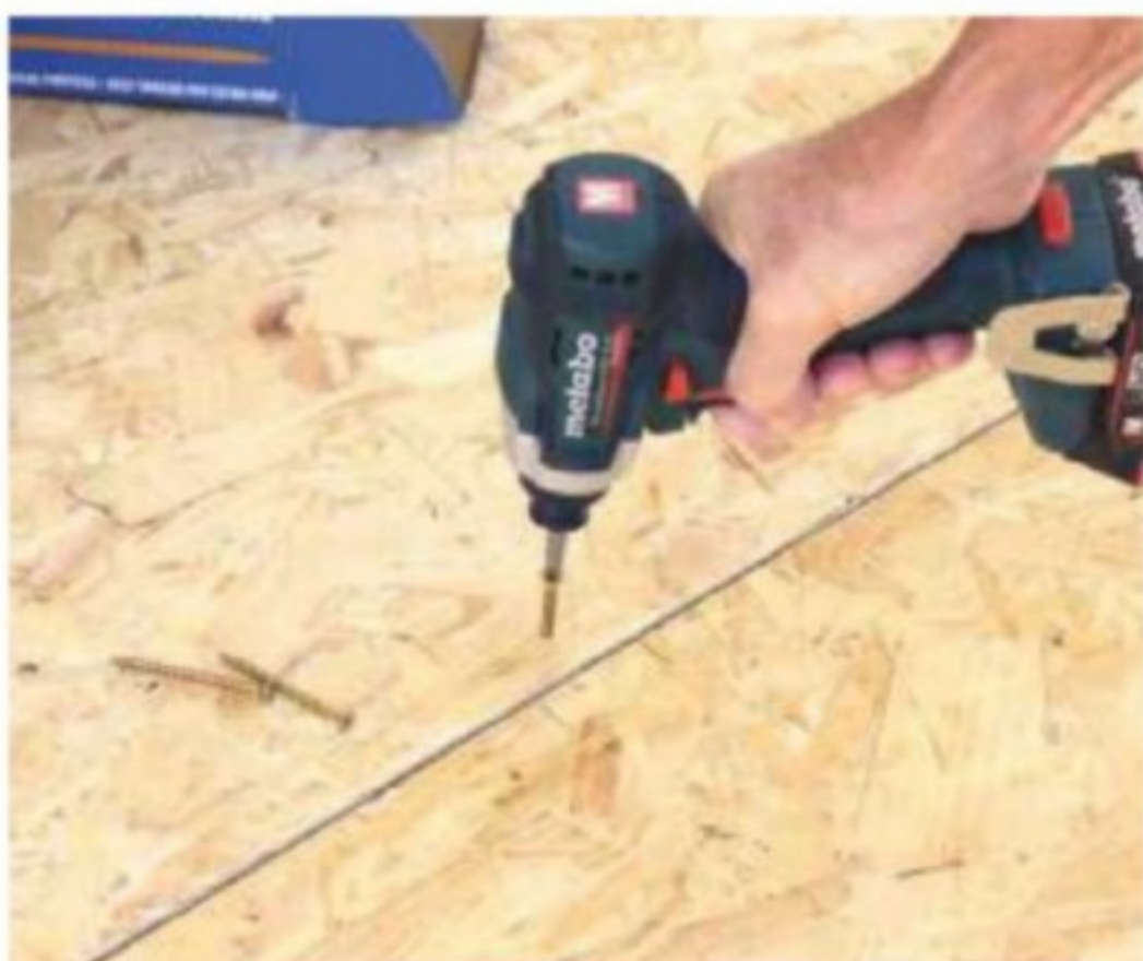
19 Fix the sheets down to the joists with countersunk screws, rather than nails. Nails could lift over time and puncture the roof covering
