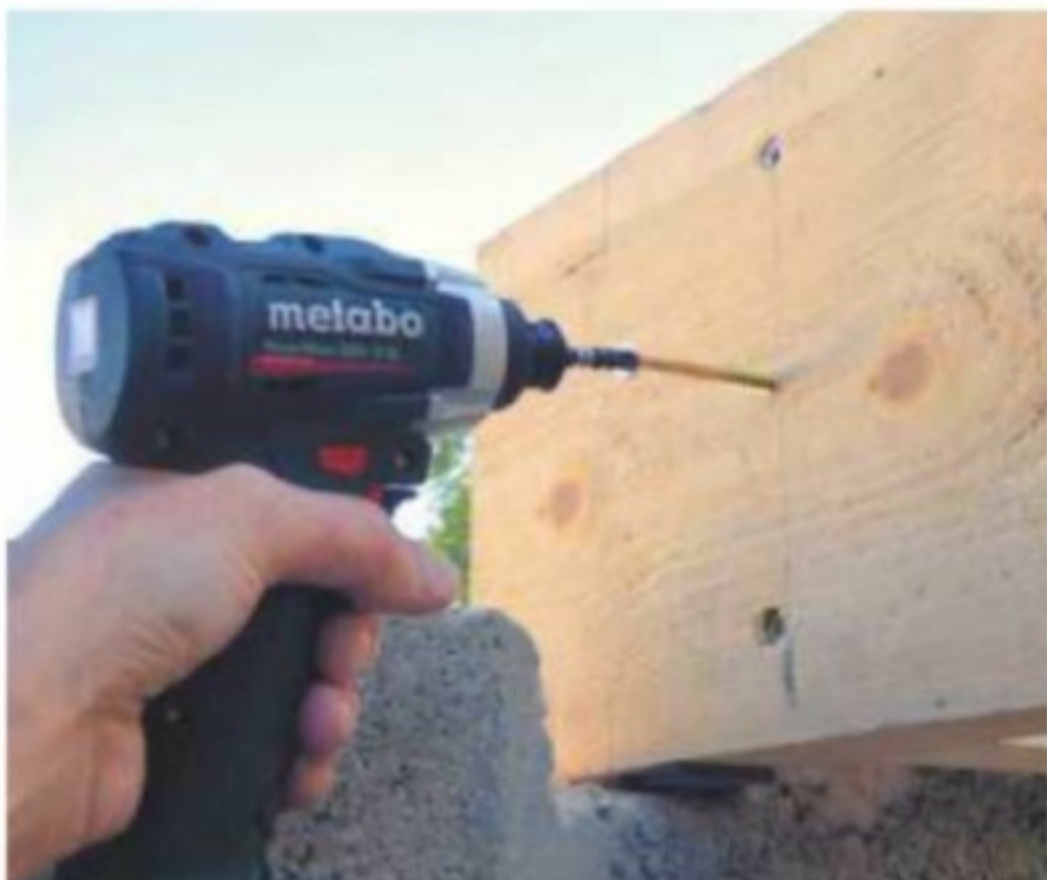
16 Where there's insufficient space for hangers you can fix joists with 6.0 x 100mm screws. Drill pilot holes and drive home with an impact driver
