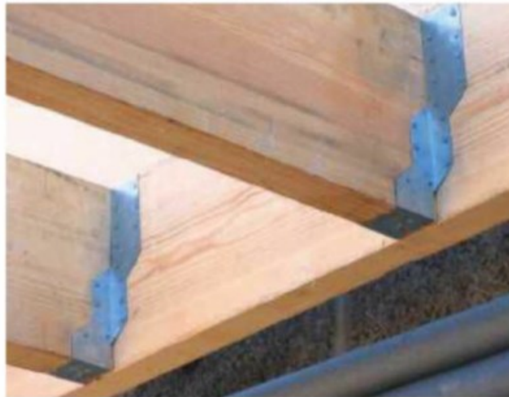
14 Bend the straps tightly over the top of adjoining joists. Use galvanised wire nails, starting from the bottom and working up
