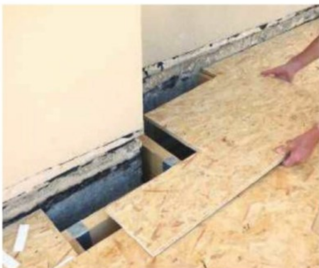
22 Use a jigsaw to cut boards around obstacles. These don't need to fit too tightly against the walls as any gaps will be covered by arris rails
