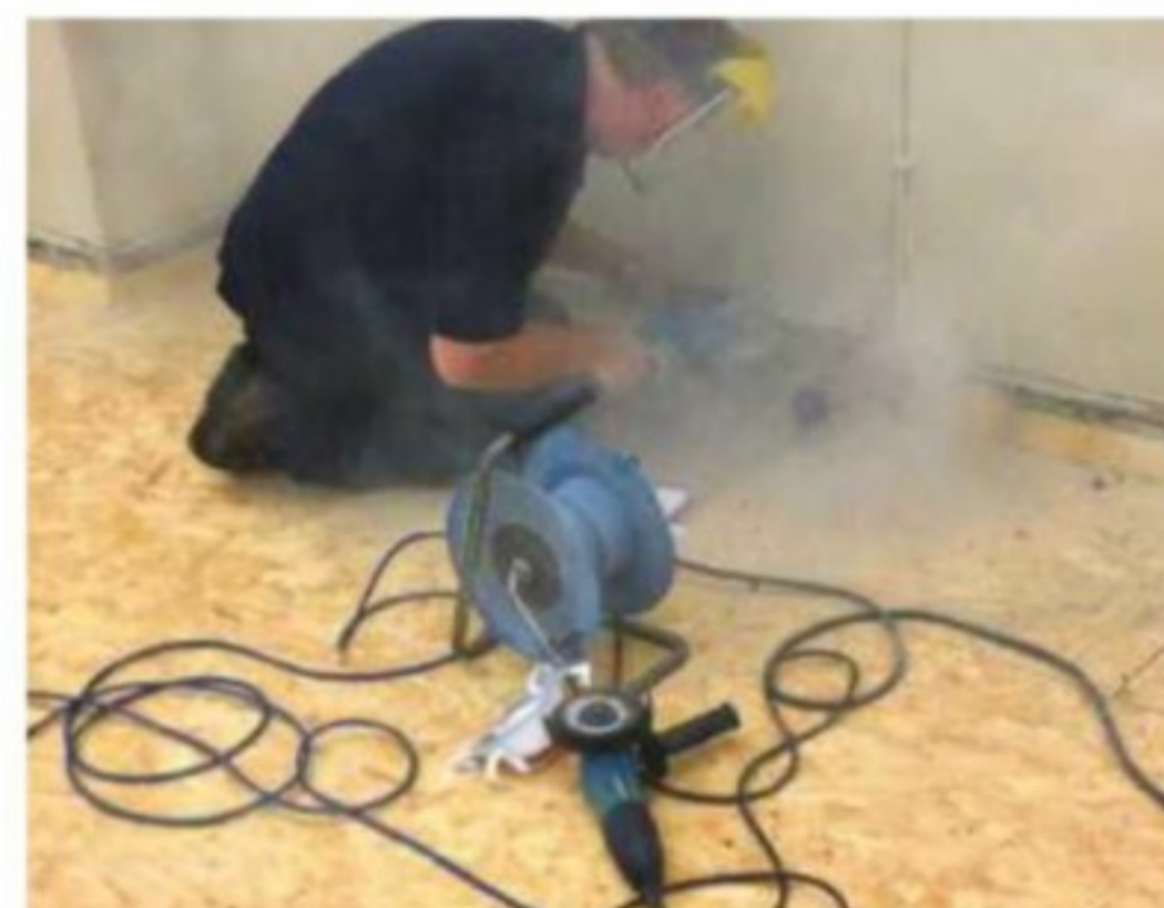
27 Once the roof covering is completed the arris rail is covered with lead flashing. The wall is chased out with an angle grinder to create the groove
