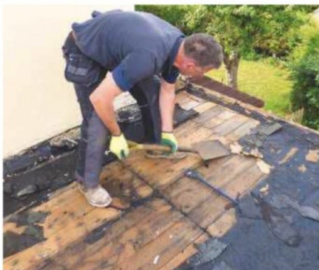
4 Stripping old roofing felt is often easier with a spade or similar tool. There are likely to be two or three layers on a flat roof, along with nails
