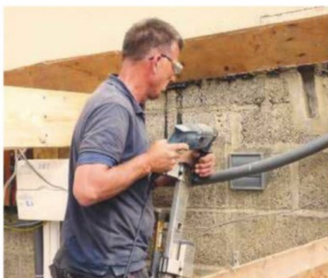
10 Where recesses in the wall are poorly spaced you may need to cut new ones. Use an SDS hammer drill to bore holes before using a bolster
