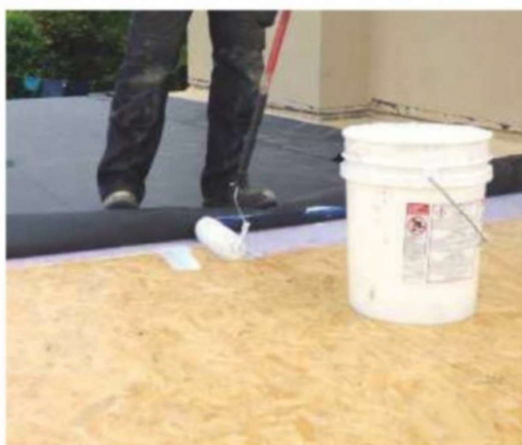
29 The rubber is glued to the decking with an industrial adhesive. This is applied with a roller and the membrane unfolded and spread across the roof
