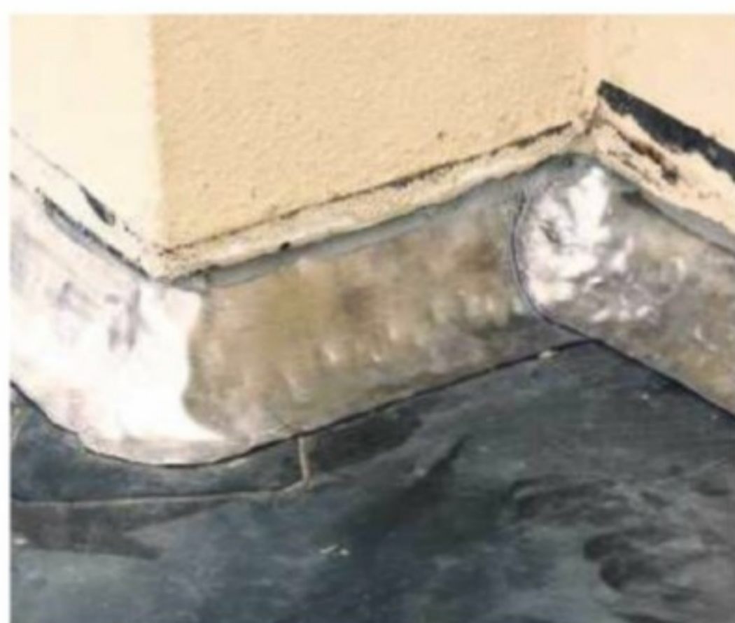
31 The membrane covers the perimeter arris rails. Lead flashing is then shaped, slotting into the gap around the wall and finished with sealant
