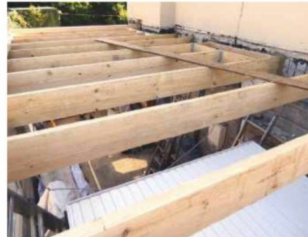
15 Here, most of the joists are fixed in their final positions. Use a long board as a straightedge to check that upper surfaces are all in line
