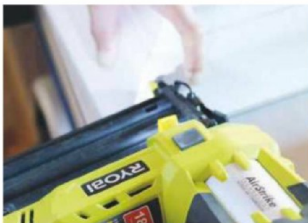
Pre-joining cornice mitres prior to installation
