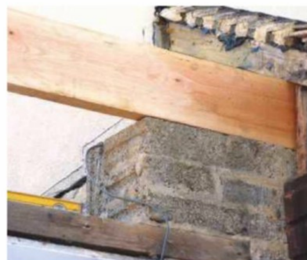
9 Starting at one end of the garage, place the first joist in position. This one sits on blockwork at each end and will be secured with steel straps
