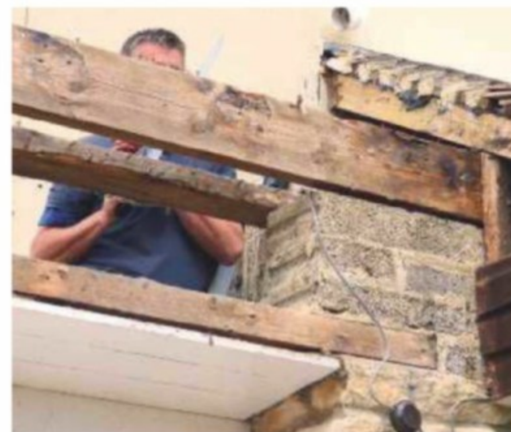
6 The existing joists had been built into the wall, so sawing through makes them easier to remove. Make sure cables are not in the way
