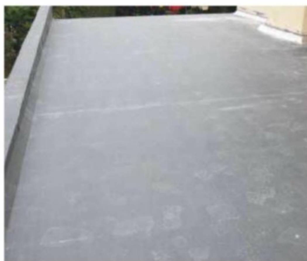
34 The completed roof and parapet wall, covered in a single piece of EPDM sheeting. Hopefully this will last for a good many years!
