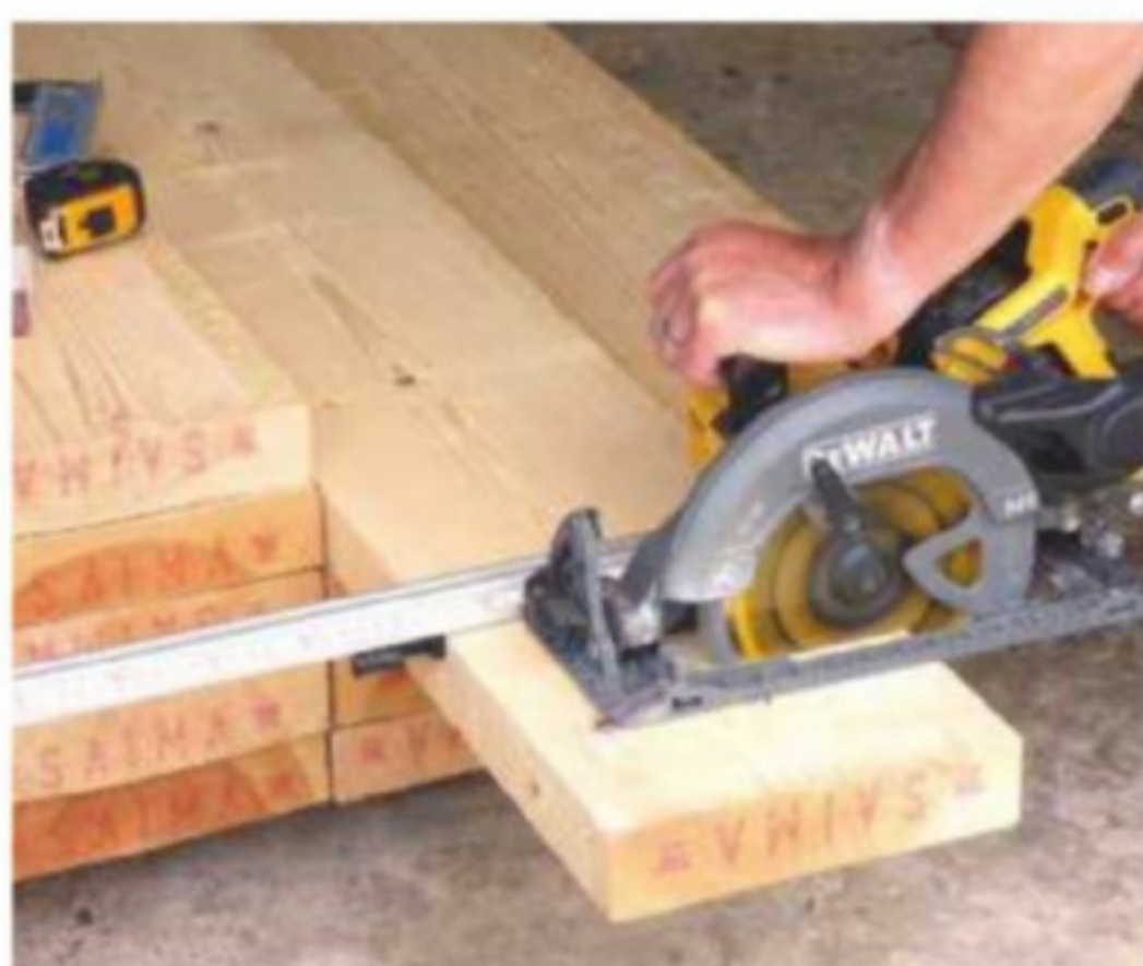
7 Measure and cut the first joist to length. If using a circular saw, use a guide clamp to ensure each cut is at 90°
