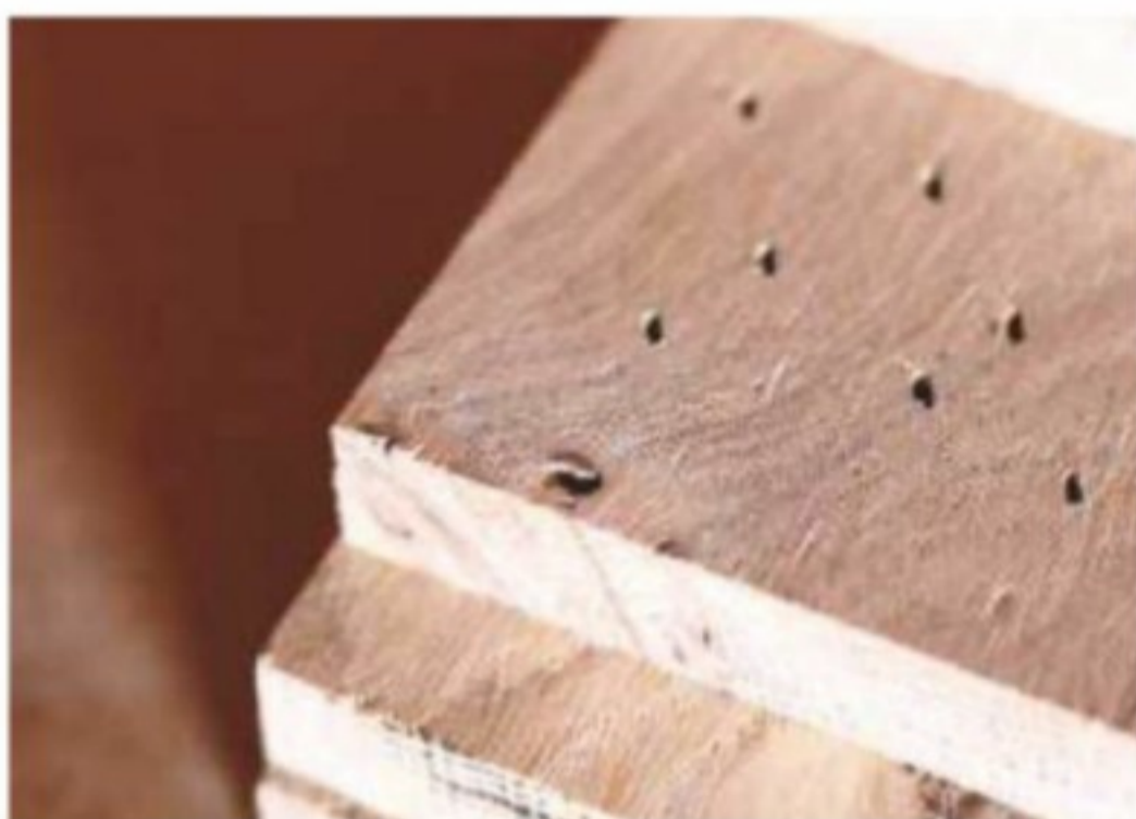
30mm nails fully sunk below the surface in solid oak
