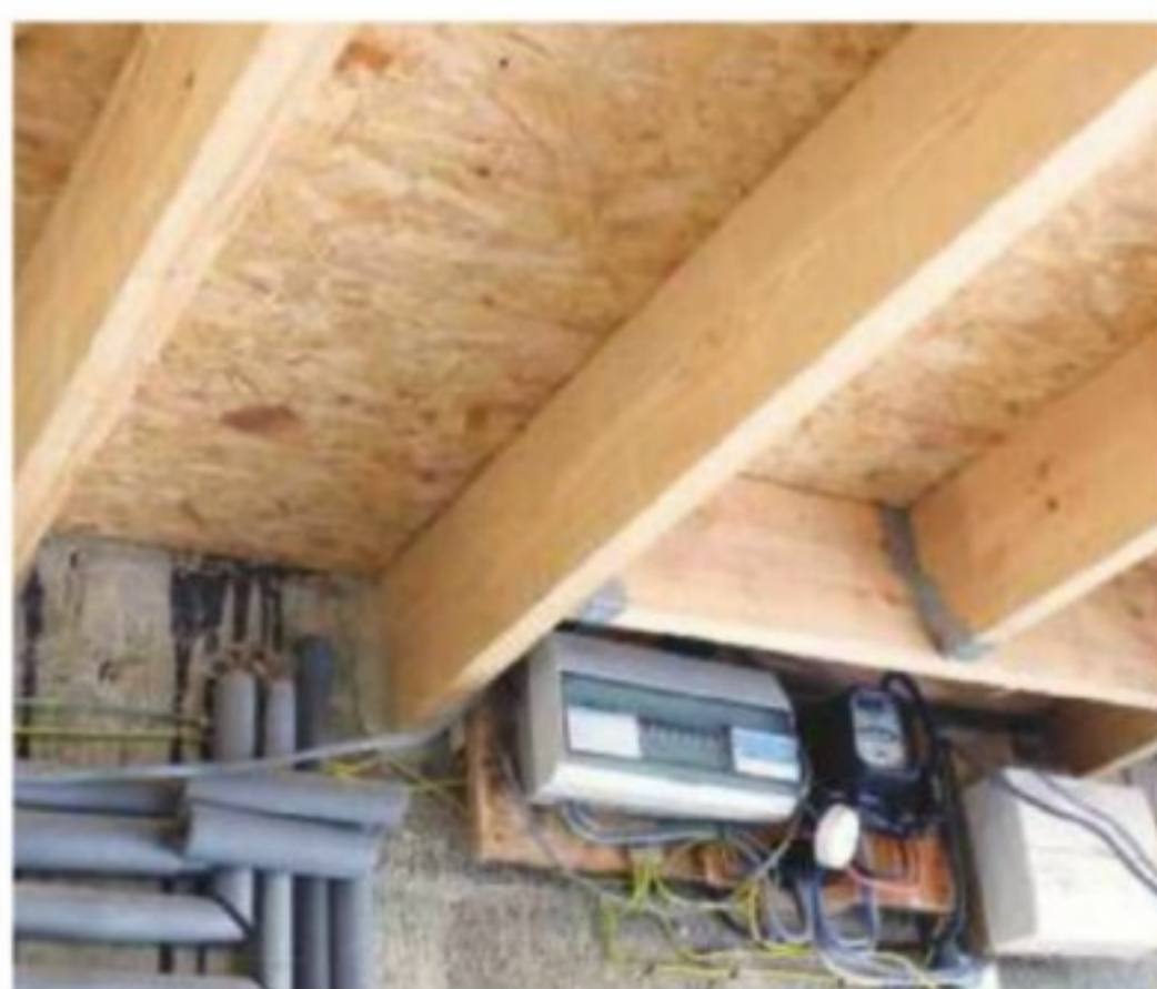
35 Trimming joists around the consumer units and other obstacles made a tricky job rather easier. Lighting cables will be re-routed along joists
