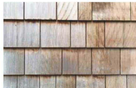
Weathered western red cedar shingles
