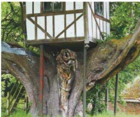
Britain's oldest existing treehouse Photograph courtesy of Pitchford Estate
