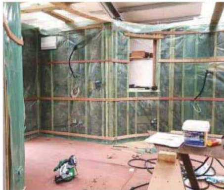
Interior walls insulated, ready for lining
