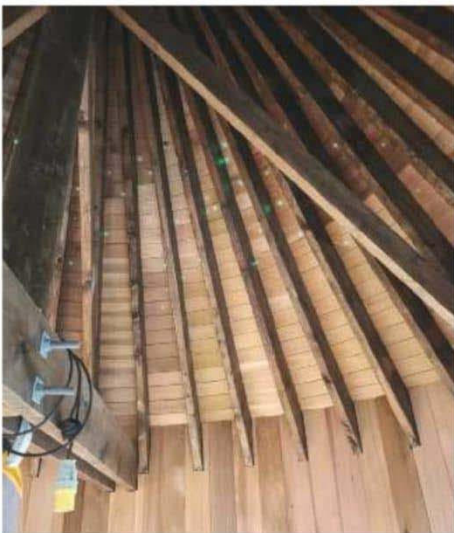
Interior cladding and second-fix electrics added
