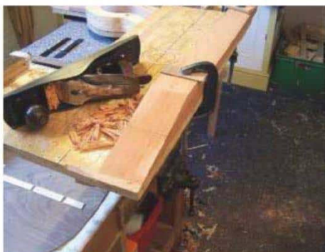
39 Planing the scarf joint for a perfect fit
