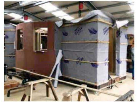
Walls being battened ready for cladding
