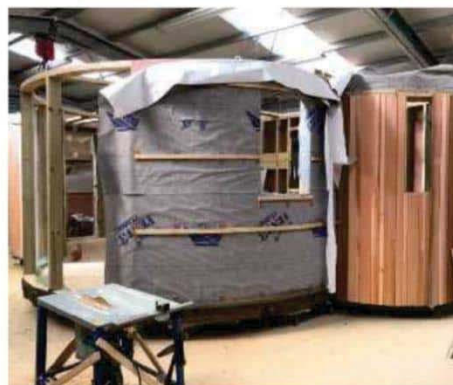
Exterior cladding being fitted...
