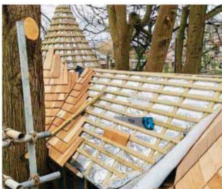
Cedar roof lining
