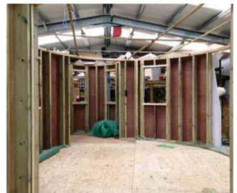
Treehouse stud walls erected
