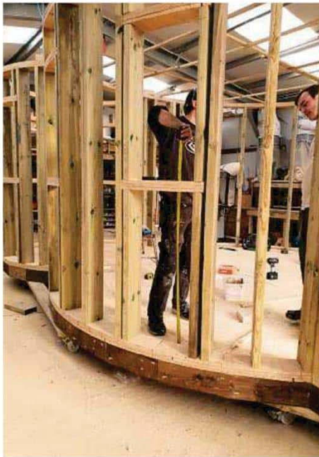
Treehouse wall framework
