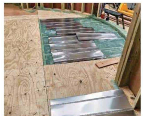
Underfloor heating trays being fitted
