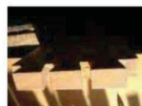
'Tails' cut showing accurate 90° from the face of the board
