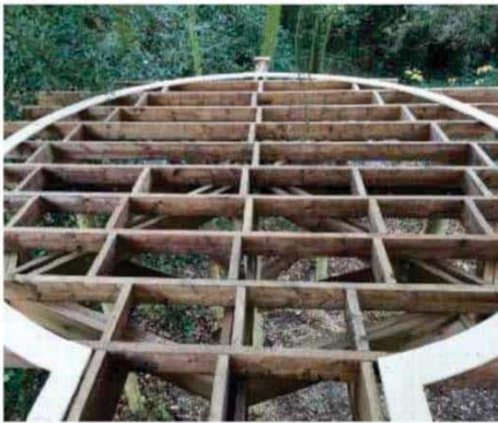
Floor joists and bottom plate
