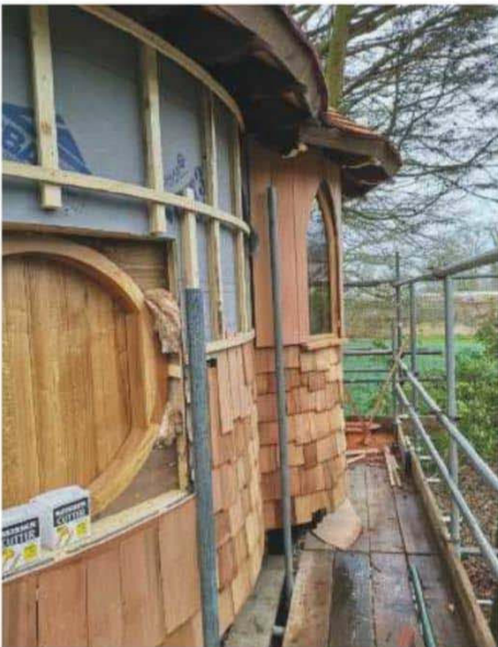
Wall cladding and fitting windows
