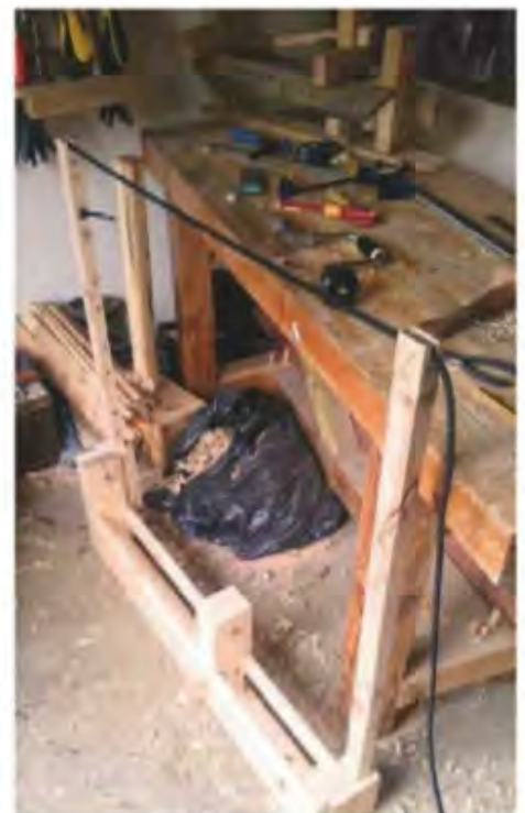
28 Testing the tension across the posts
