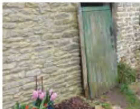
1 The original door to the outhouse was in a pretty bad way. A new frame was made and installed before work could start on a replacement door
