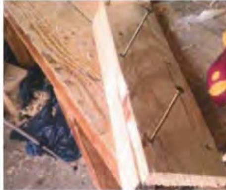
23 Screwing a back piece onto the post housing
