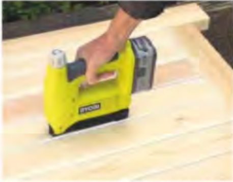
25 With pencilled lines as a guide, nail the boards to the mid and bottom rails. Use either brads or lost head nails, at least twice board thickness
