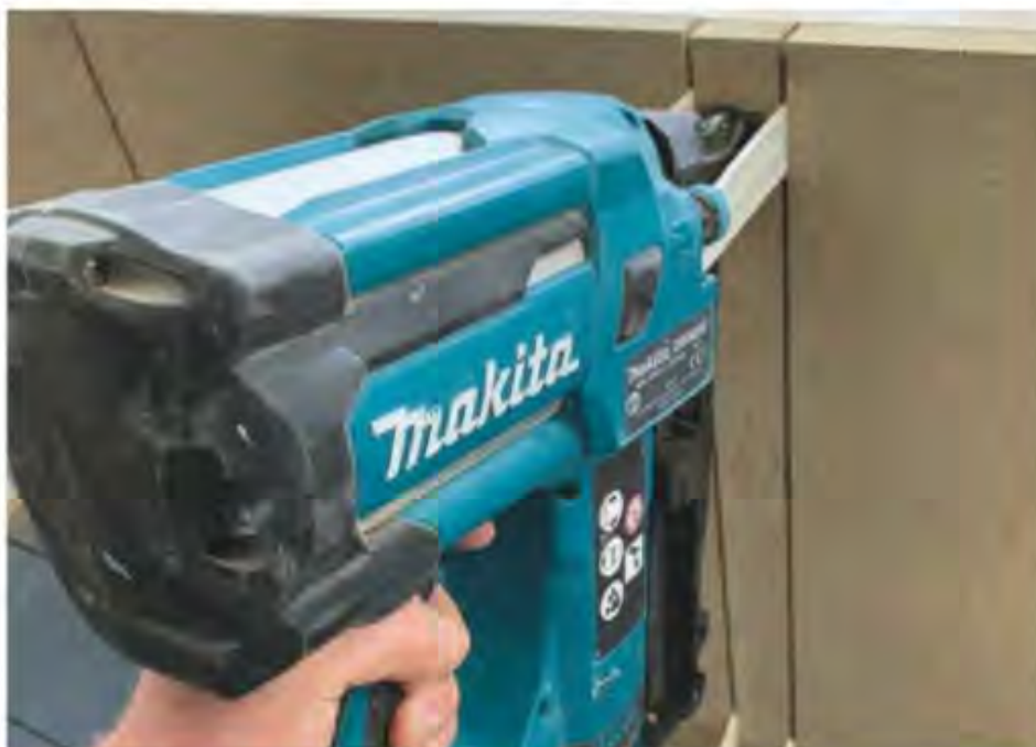
Material packed into position and fixed with the nailer
