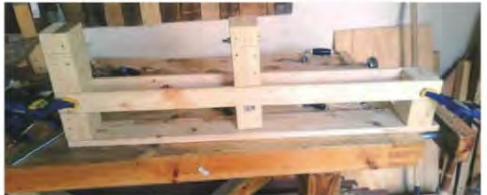
17 Clamping the rails to the stocks to make drilling and screwing easier
