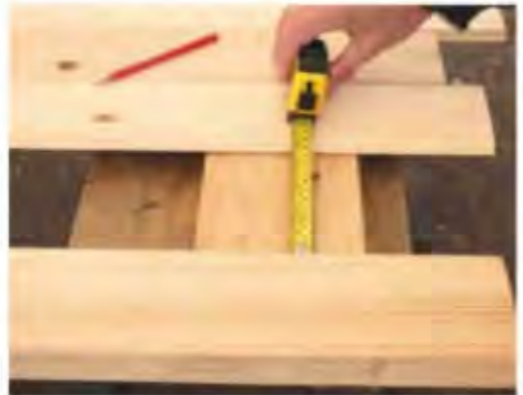
21 Fit the matchboard loosely together and check the distance you'll need to fill with the outer two boards. These will probably need to be cut down
