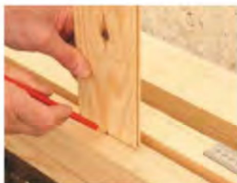
4 The mid and bottom rails are thinner to accommodate the matchboard thickness, which in turn determines the position of the mortises
