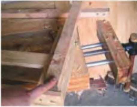
19 Finding the position for the vertical posts
