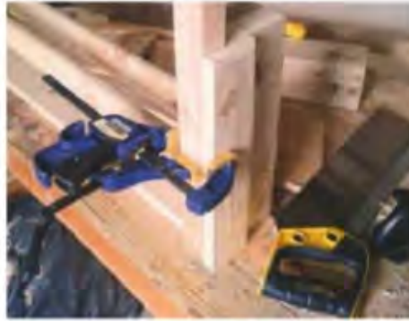
20 Clamping sections to hold the posts
