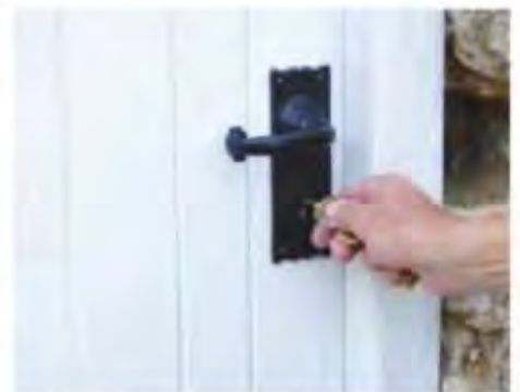
36 Finally, drill mounting holes for the handle and check that the lock operates smoothly. Then you can undercoat and complete with a final top coat
