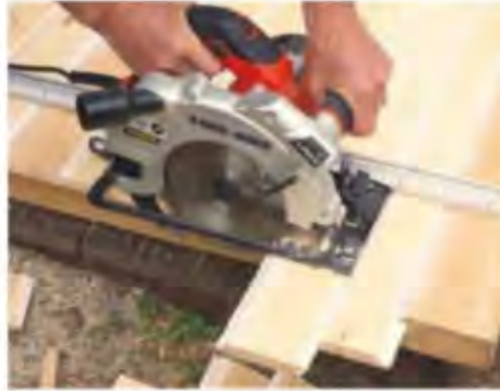
26 Mark the door for final length and cramp a guide rail across the bottom. Set blade depth and cut the stiles and boards in one pass of the saw
