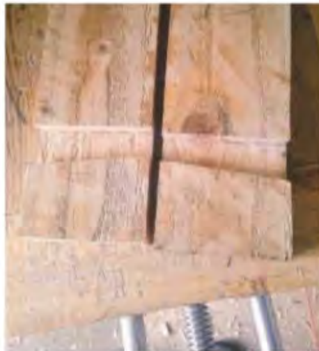
6 The wedge mortise cut out
