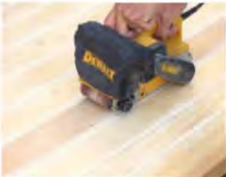
31 Check the front and back surfaces of the door and clean up with a bench plane. Finally, sand the front ready for brushing on a coat of primer
