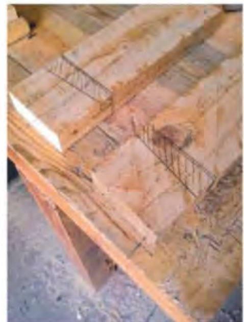
5 Marking the correct angle for the wedge
