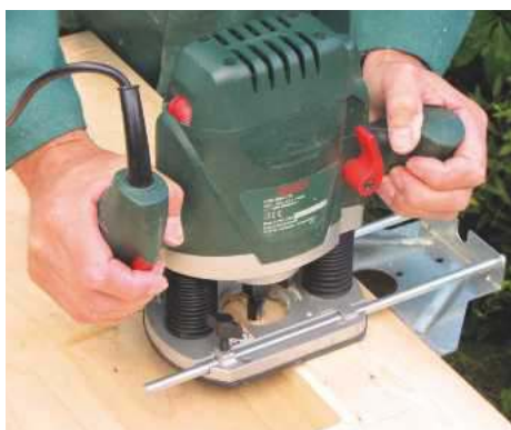
7 Rout a 7mm-deep rebate around the inner edge of the frame, using a fence or guide rail
