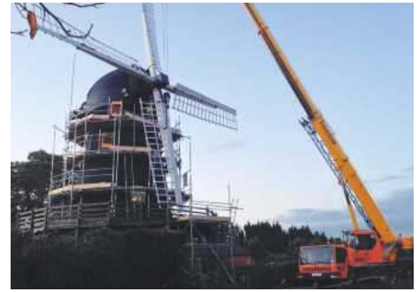
13 Crane lifting up sails to be attached Photograph courtesy of Luke Bonwick
