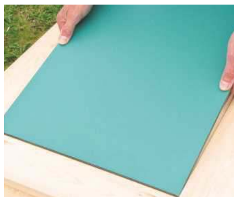
9 Check that the mirror glass fits into the frame. There should be a slight gap to allow timber to move
