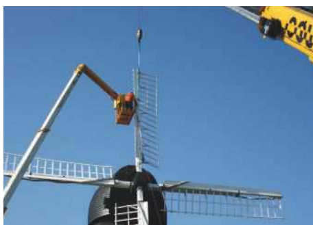
5 Here a cherry picker is used to carry out 'operation cherry picker'
