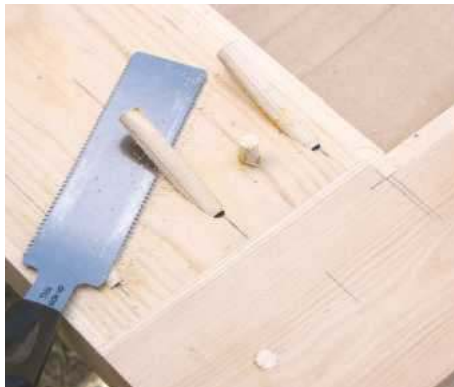
20 Cut off projecting plugs with a flush-cut saw when the glue is dry. Trim with a block plane
