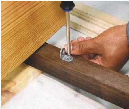
30 Screw small brackets to the end frames to support each shelf
