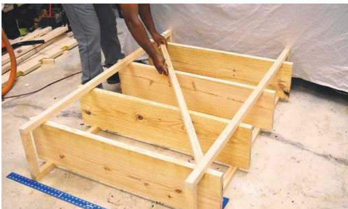
11 Check the first cross support is a snug fit between the two uprights
