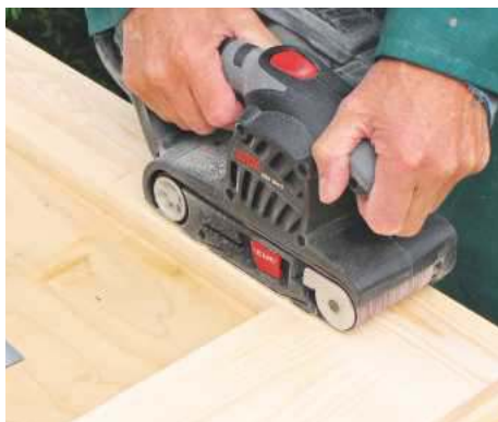
11 Before fitting the front shelf, sand the face of the frame ready for painting
