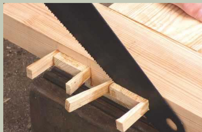
Simply saw off the excess tenons and wedges and clean up with a plane
