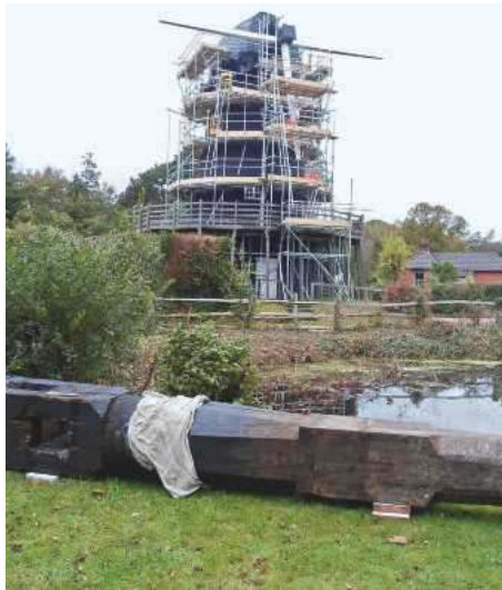
12 Scaffold tower in front and scaffolding behind so you have good access when fitting the sails Photograph courtesy of Luke Bonwick
