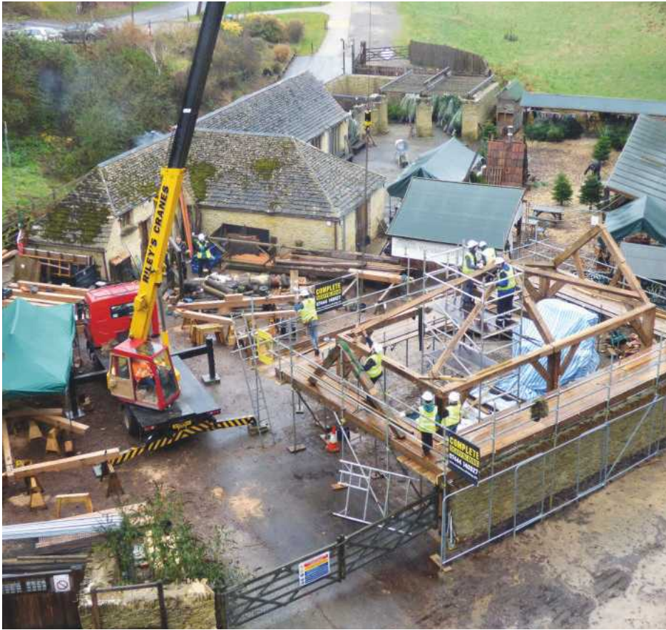
When I visited, a crane was lifting some of the substantial roof trusses into position
