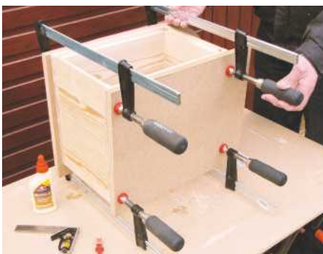
7 Assemble the box with PVA glue. Measure across diagonals to check for square, adjusting cramps if necessary
