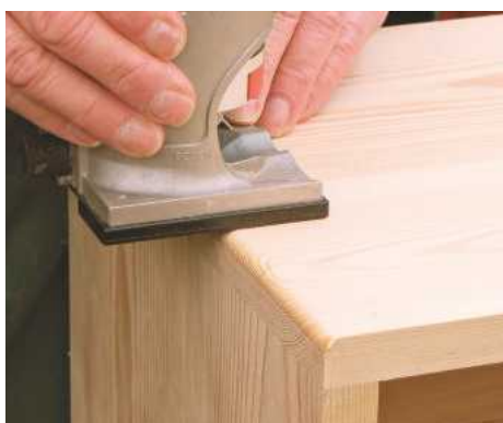
11 Rout vertical and bottom edges with a bearing-guided round-over bit. Lightly chamfer the top edges
