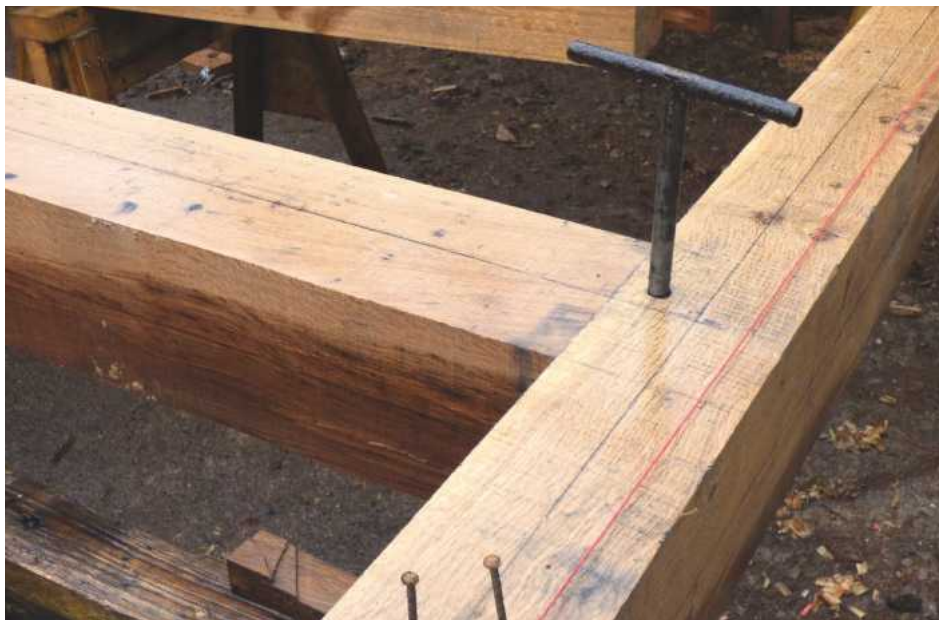
Framing pins, a familiar tool for timber framers, ensured that joints pulled up tightly
