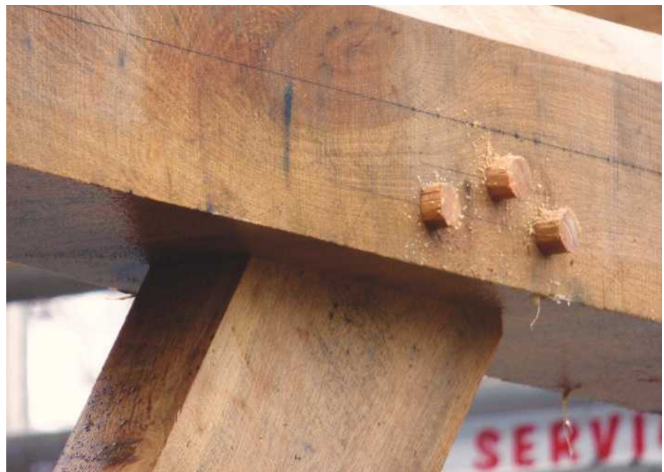
... with tenons pegged after they'd been slotted into their mortises
