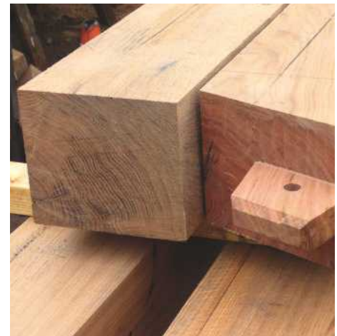
From green oak, all joints were cut on site...
