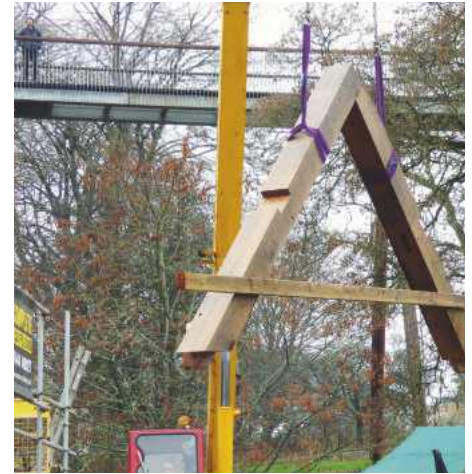
When I visited, a crane was lifting some of the substantial roof trusses into position
