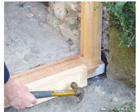
30 Use a timber offcut to prevent damage if you need to whack the frame into position with a hammer...
