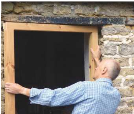
28 You will probably need to check the frame several times if it's a fairly tight fit. Here, the lintel was bowed so shims were needed
