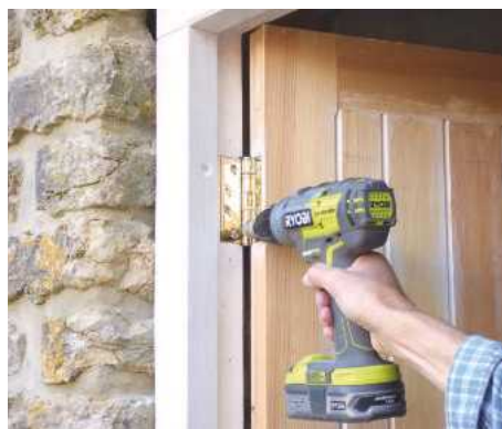
35 After cutting hinge recesses, screw the door into the frame and check it closes properly. Install a mortise lock and lever handles
