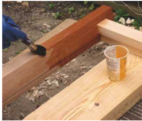
26 After final sanding, brush on two coats of wood preservative. Allow this to dry for a couple of days before painting
