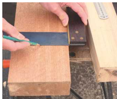
6 Select face sides and edges on all components. Next, mark the head and threshold to length while cramped together
