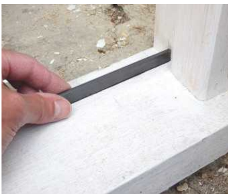
34 Cut the water bar to length with a hacksaw and tap into the threshold groove. The door is rebated and conceals it when closed
