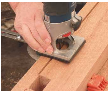
16 Rout a groove along the threshold for a galvanised steel water bar. Typically 4mm thick, this should be a fairly tight fit
