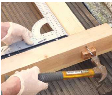
20 Assemble the frame with 125mm round wire nails. Hold a large square inside each corner as you nail them together
