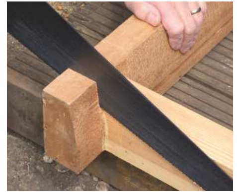
27 If necessary, saw off horns to fit the frame in the opening. It's better to allow for these by building them into the masonry, though
