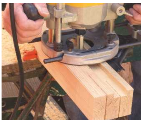
11 Cut rebates for the new door along the inner faces of the head and both jambs with a router. These should finish at 12mm deep
