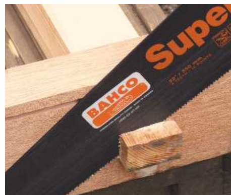
21 When the glue has dried saw off the excess from each tenon. Punch nail heads below the surface before doing this, though
